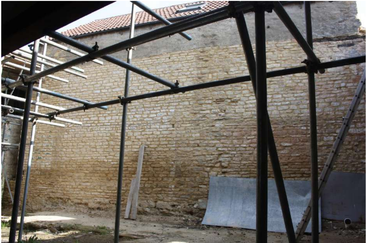
Plate 17: Courtyard area 3-4 looking northeast.
