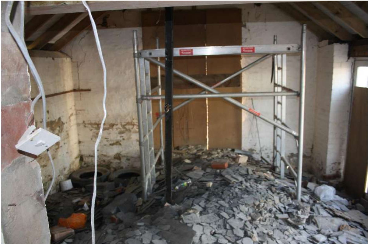
Plate 26: Old Bake House element of 5 looking southeast.
