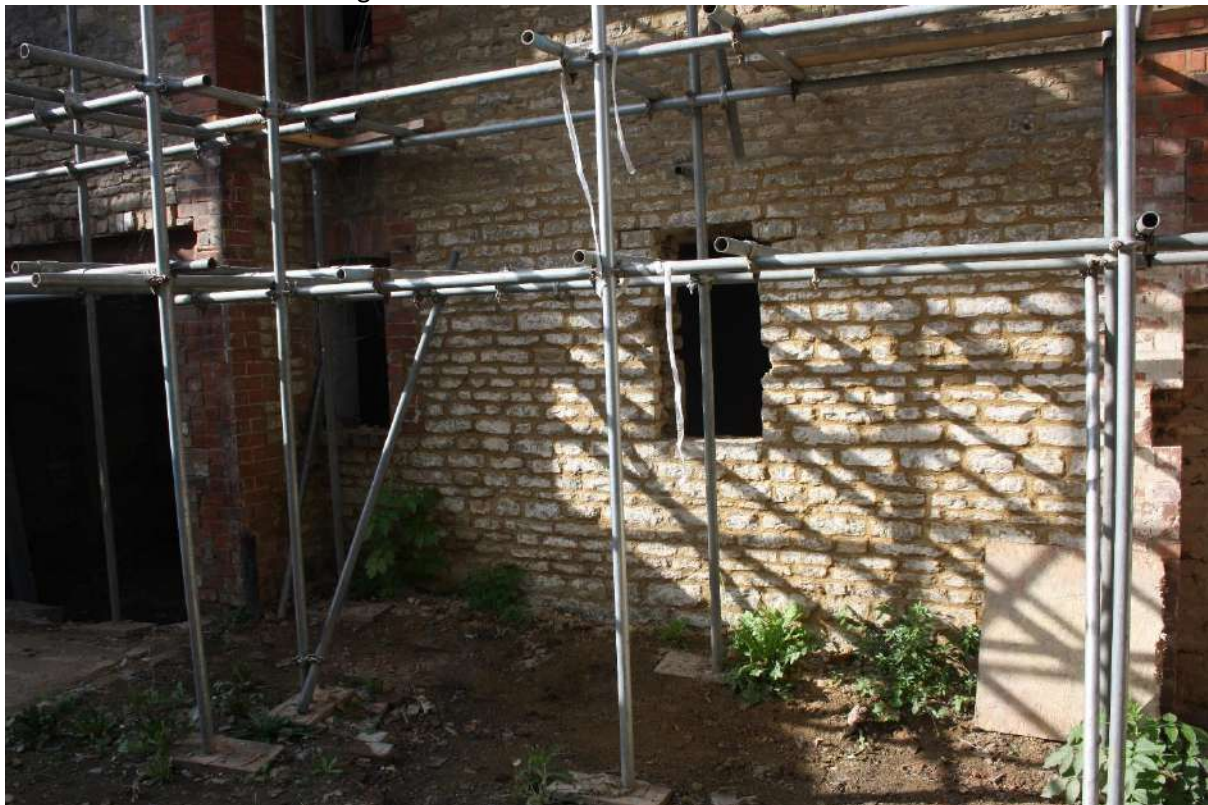
Plate 14: Yard area looking southwest at east facing elevation.
