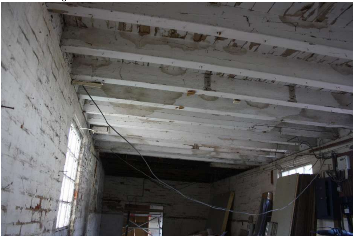
Plate 28: 5 looking south at ceiling.
