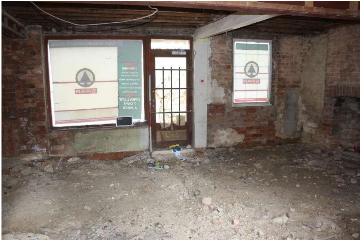
Plate 11: 3-4 looking northwest towards main entrance.
