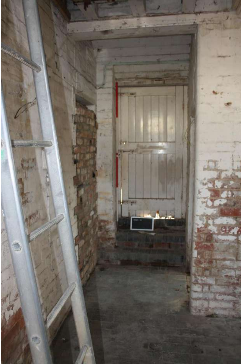
Plate 32: Entrance to yard area looking east.
