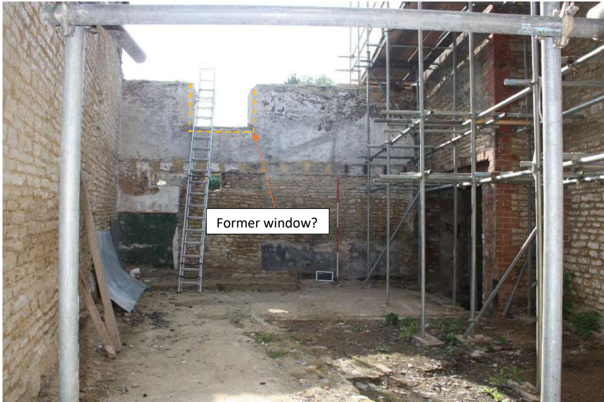
Plate 13: Yard area 3-4 looking southeast.
