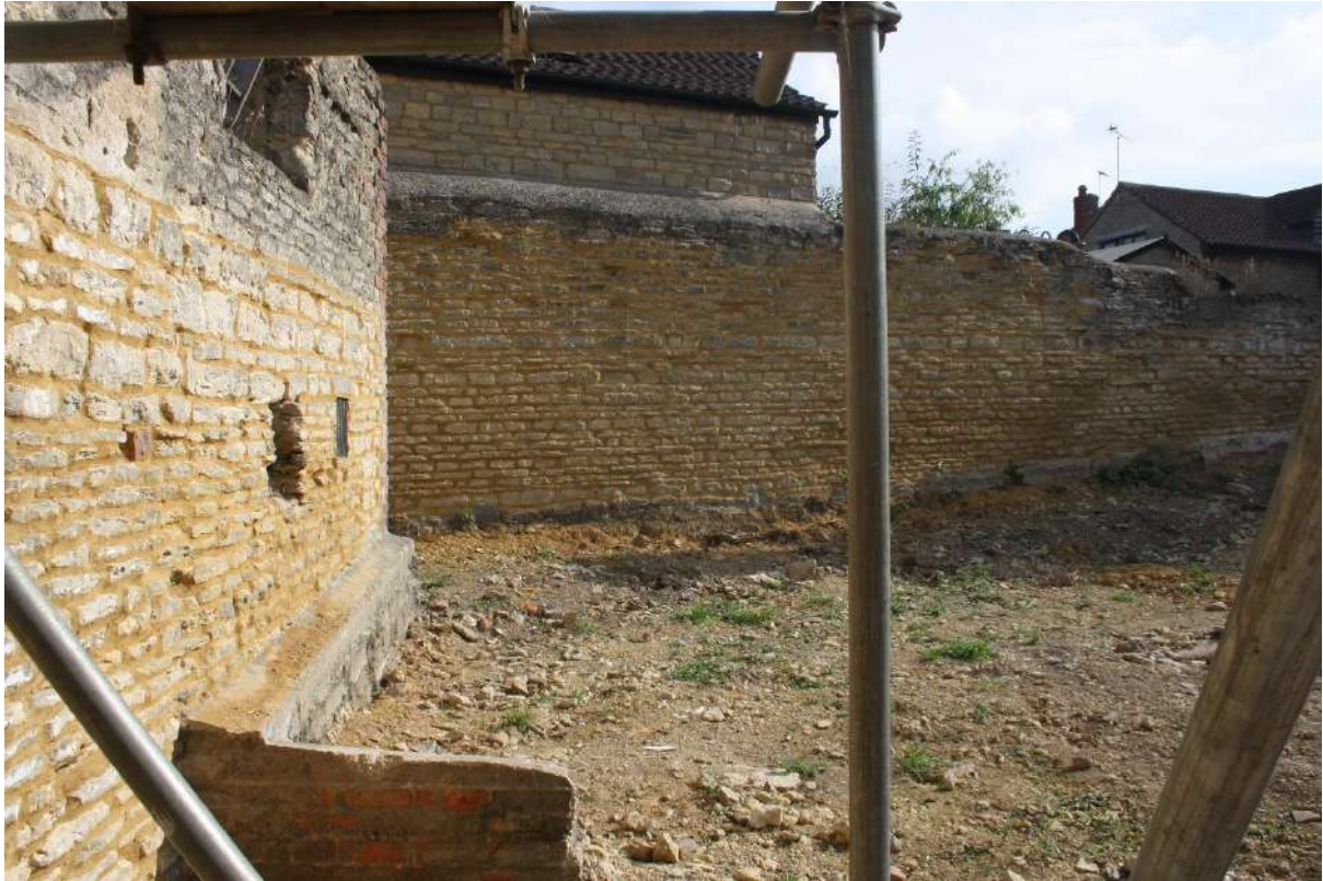
Plate 25: Yard area to east of 5 looking west.
