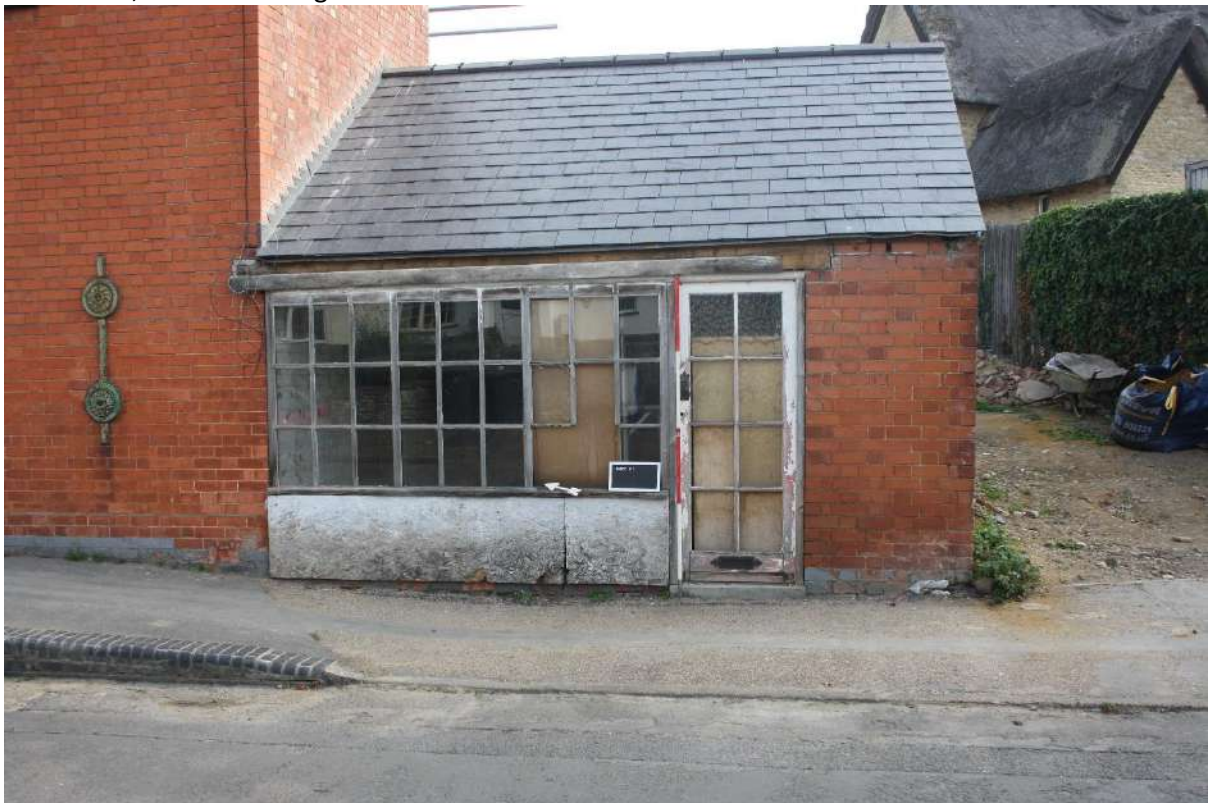
Plate 20: Old Bake House attached to south of 5 looking east.
