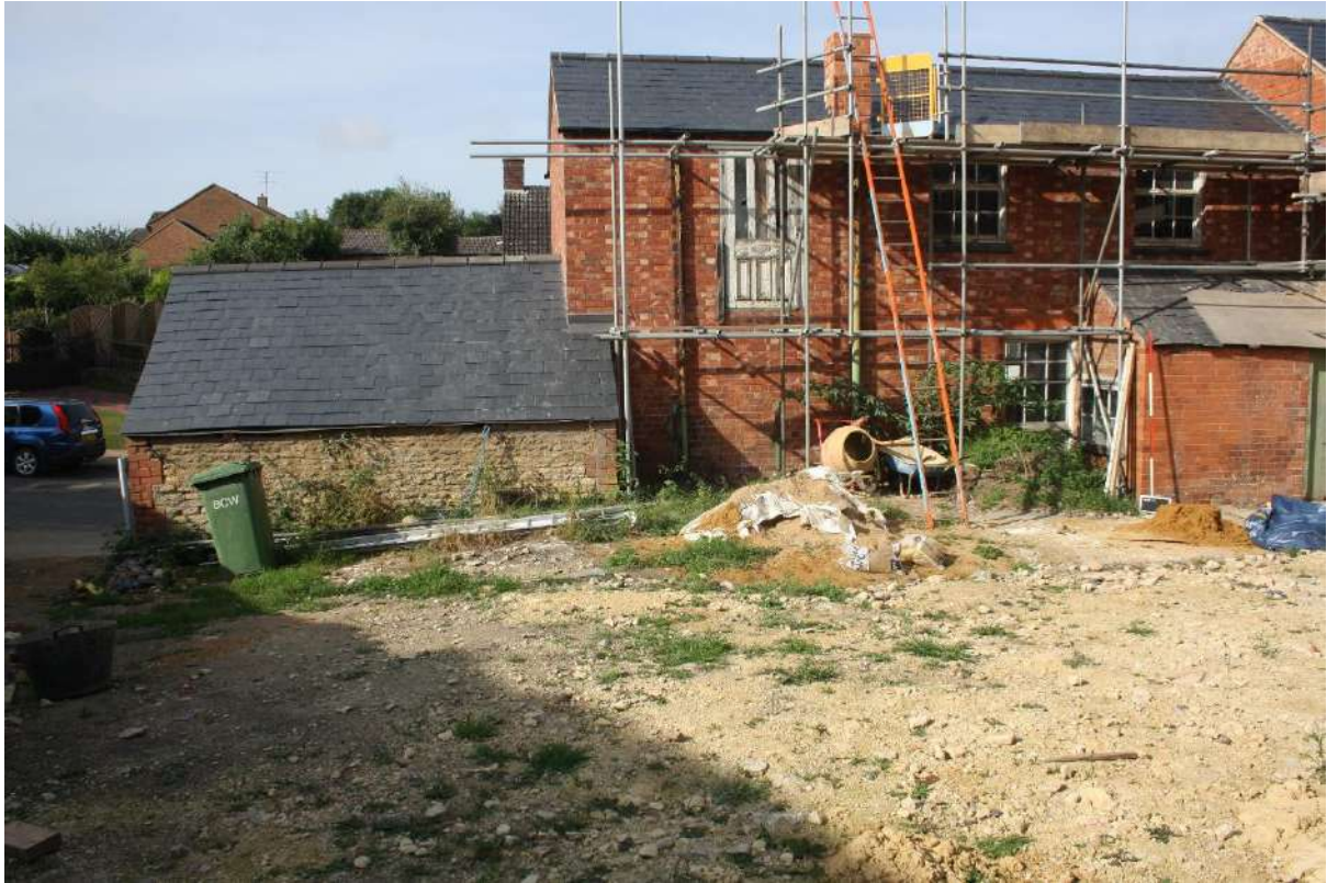
Plate 23: East elevation of 5 looking west.
