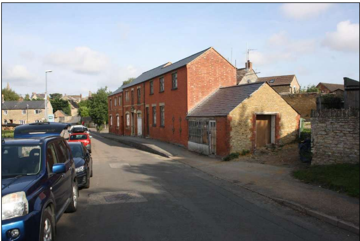
Plate 1: No.5, 3, 4 Camden Square, with Bakers Shop in foreground.
