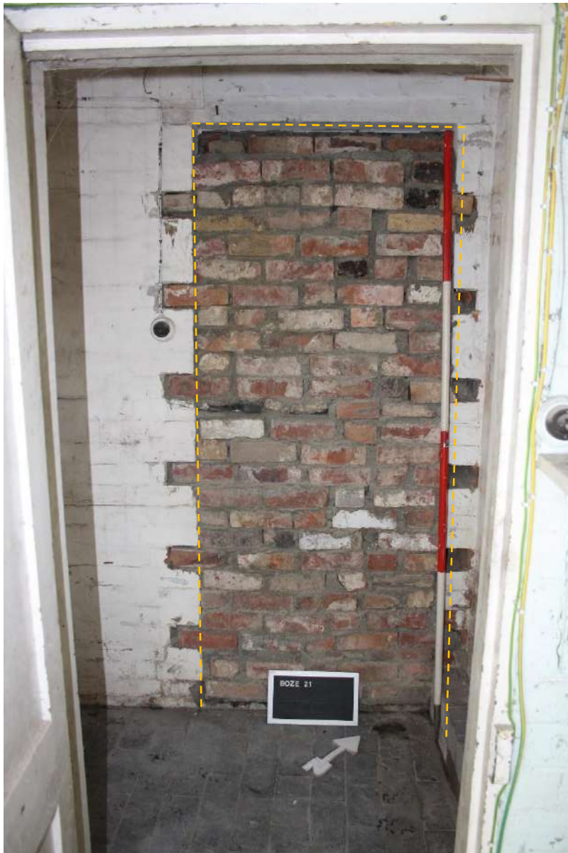
Plate 31: Blocked entrance leading from 5 into 3-4 looking northwest.
