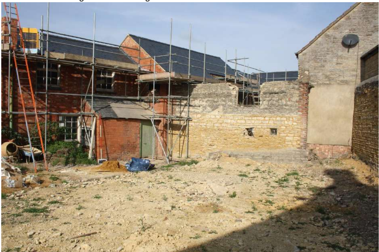
Plate 22: Yard area to east of 5 looking northwest.
