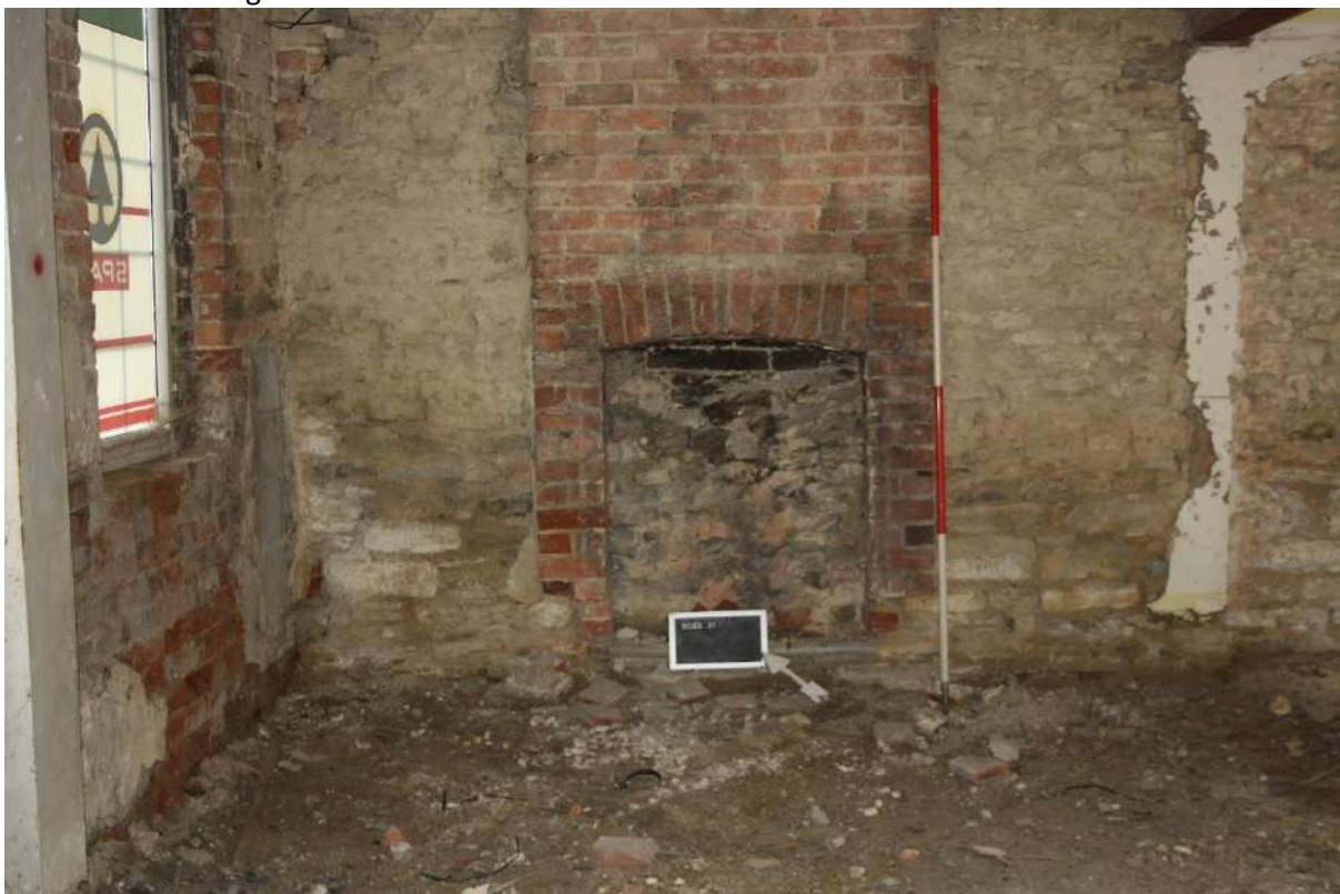
Plate 10: 3-4 fireplace opening looking northeast.
