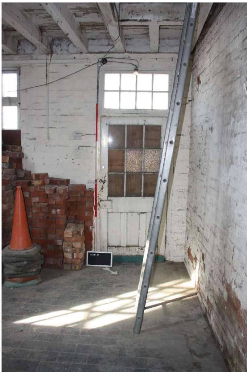
Plate 29: Entrance to 5 looking southwest.
