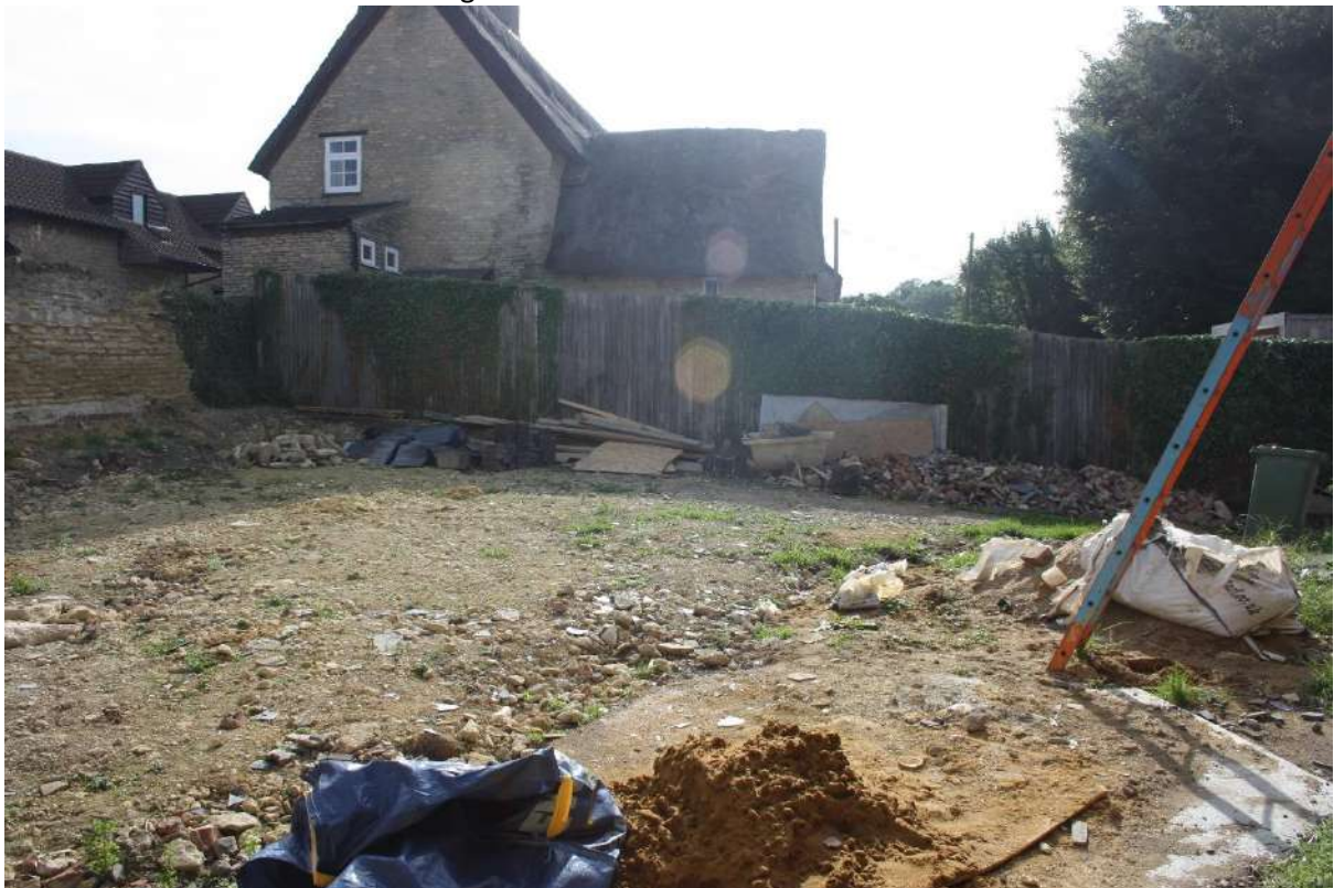
Plate 24: Yard to east of 5 looking southeast.
