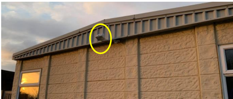
7. External light on side of the Small Hall
