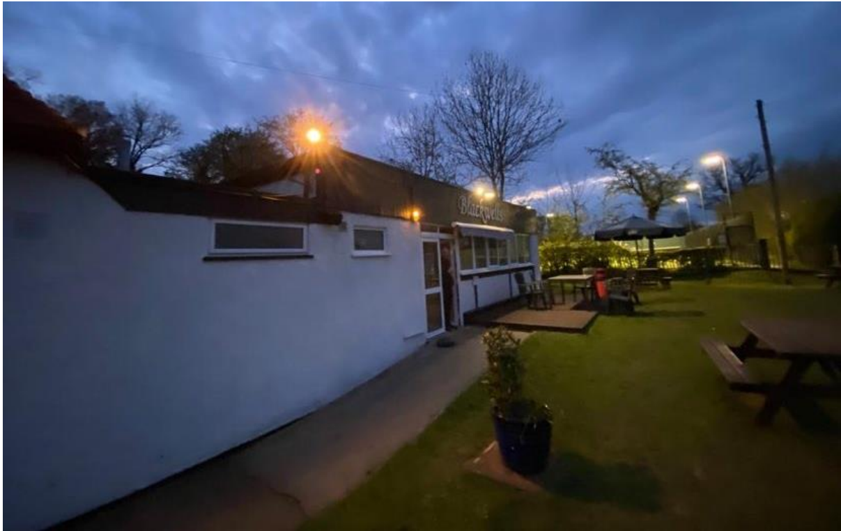
3. Side of Blackwells facing front court. 4x external lights
