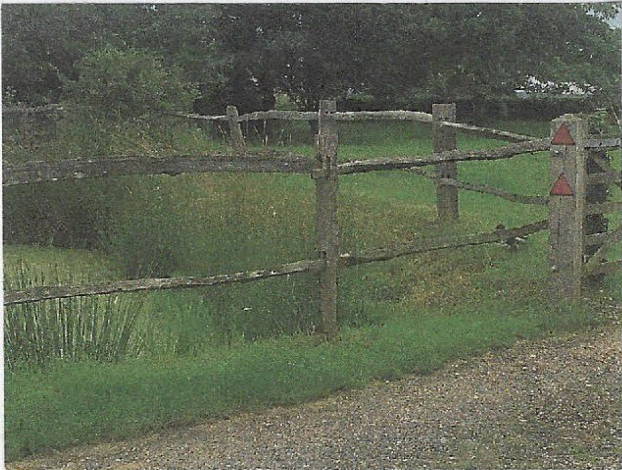
1.2m Post & Rail Fencing.
