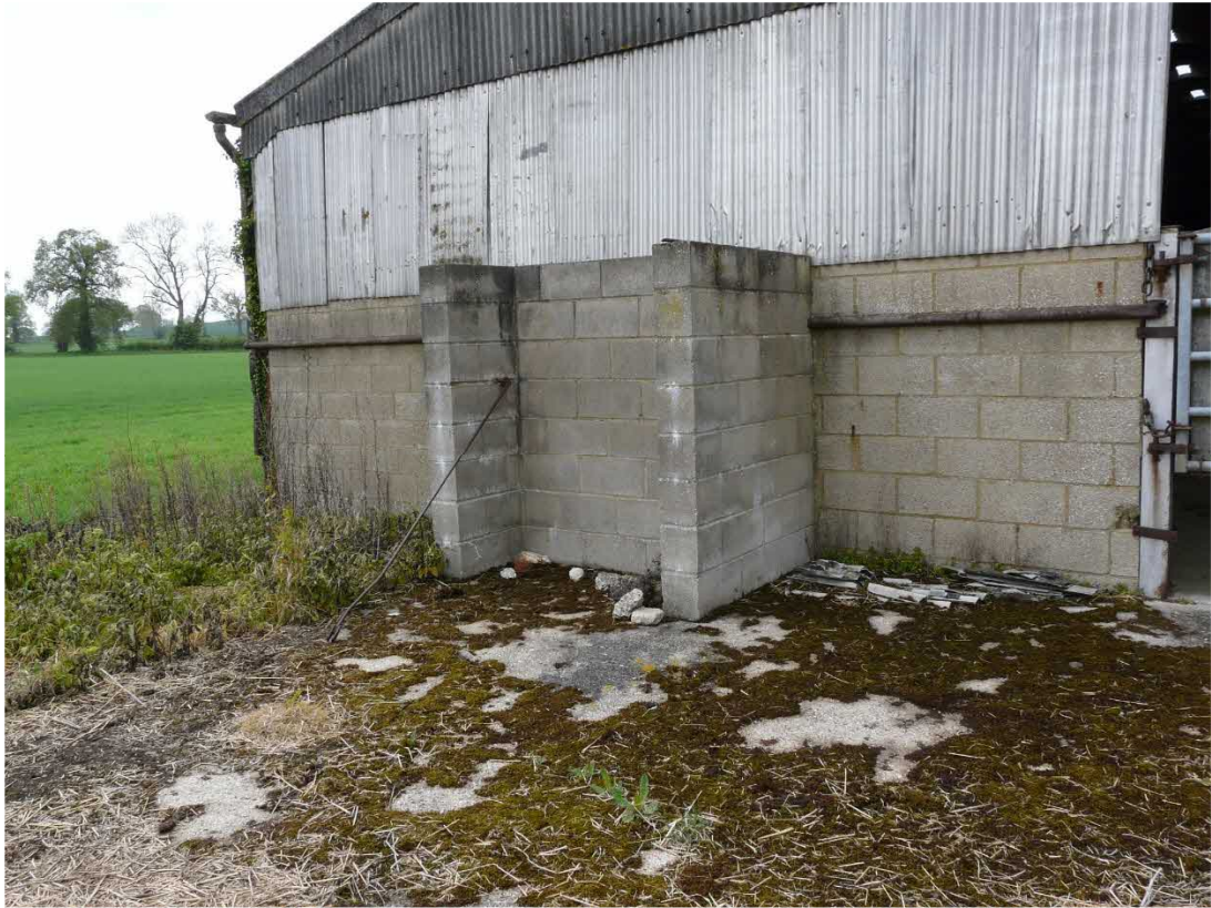
Plinth for former fuel tank
