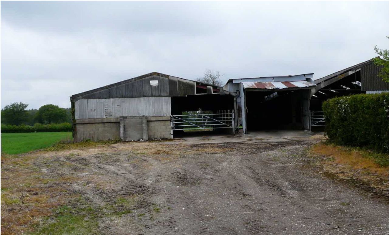
Southern side of barns viewed north-west
