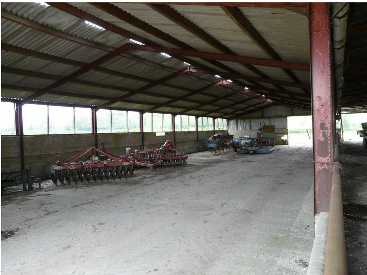
Interior of western barn to be converted
