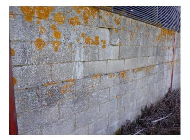
**2.12** To the 5<sup>th</sup> and 6<sup>th</sup> bays along the left side part of the top course blockwork has been displaced and some blocks are missing. Again this appears to be due to impact damage from the inside and merely requires to be rebuilt as necessary.
