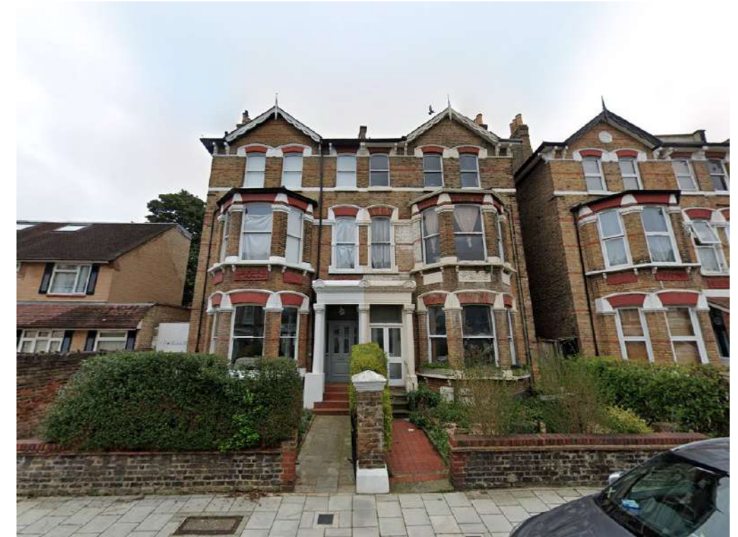
Front elevation of 17&19 Montrell Road
