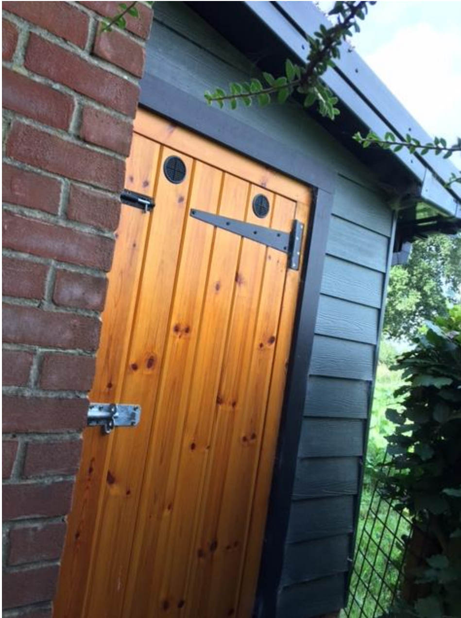
Rear/norther elevation of new extension
