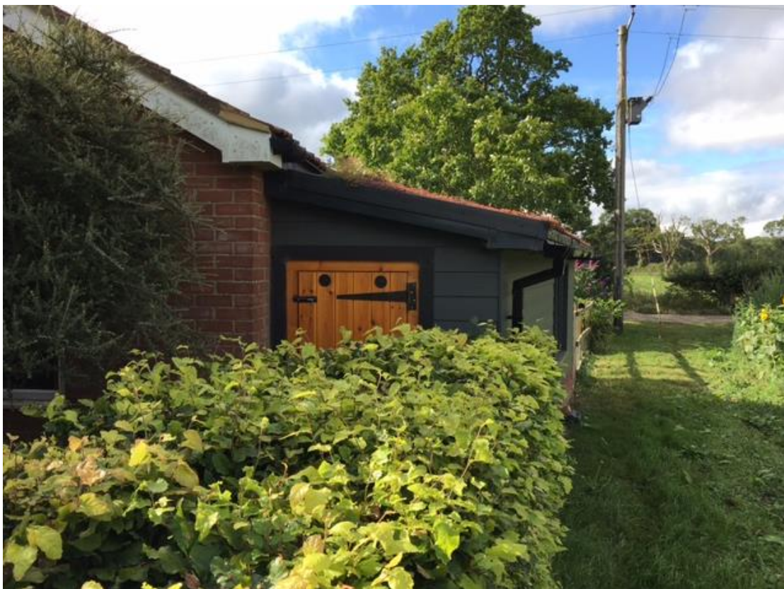
Northern elevation on new extension
