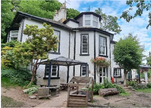
Photo 1. Main building onsite.
