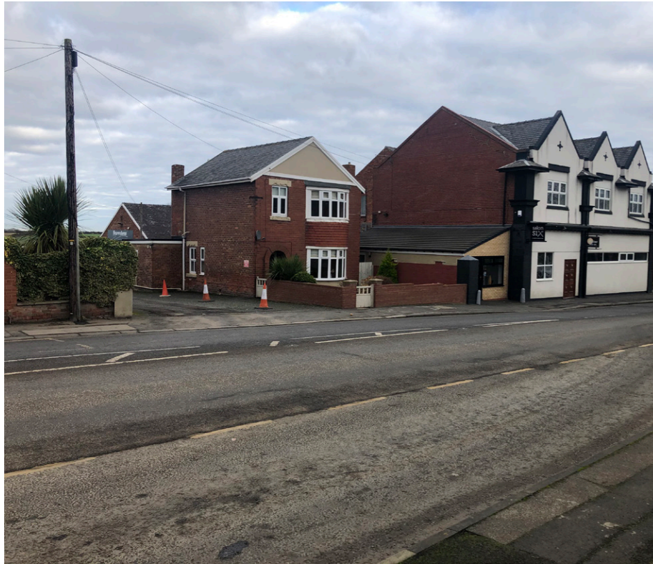
A - Site access point, Seaside Lane showing Longlea (to be demolished) and existing Jupiter Club to remain
