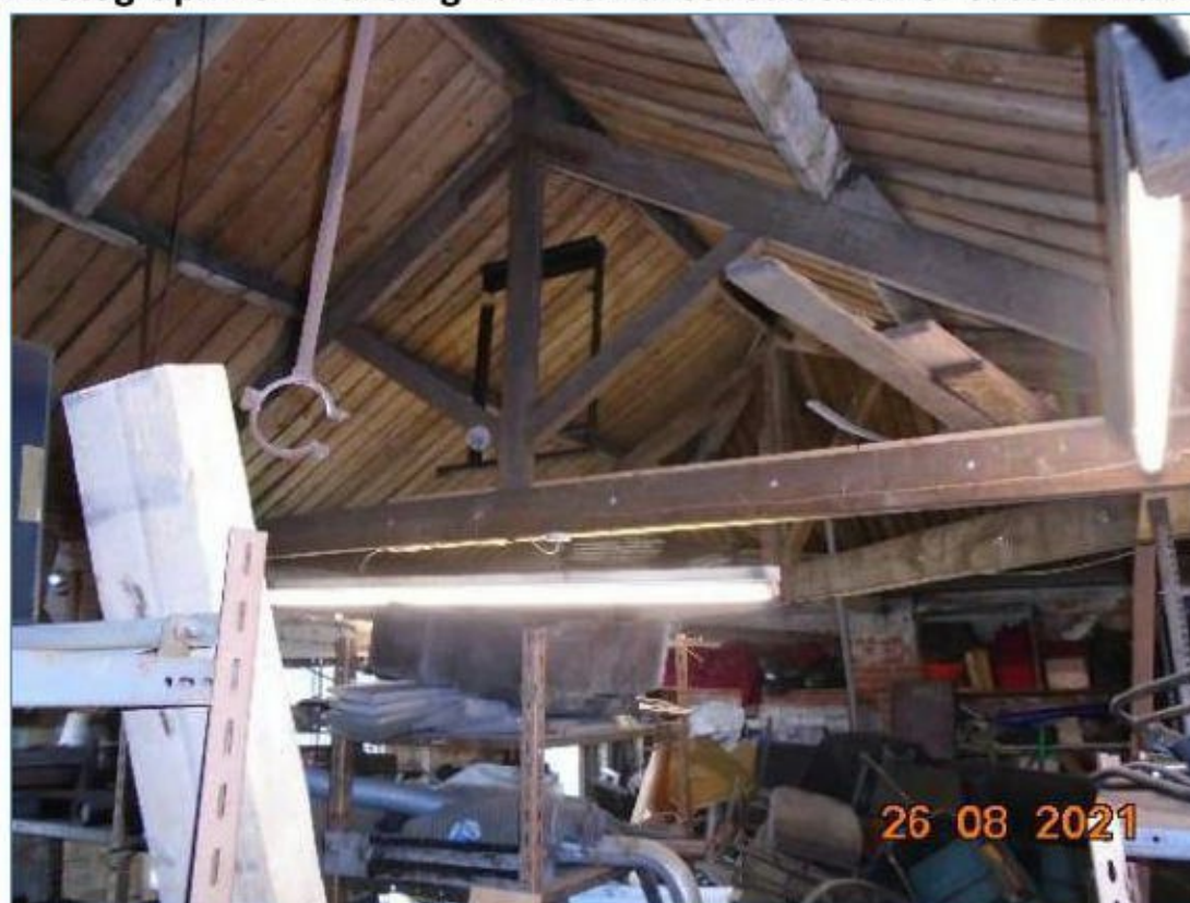
Photograph 16 – Building 1: Internal construction of eastern half of building.
