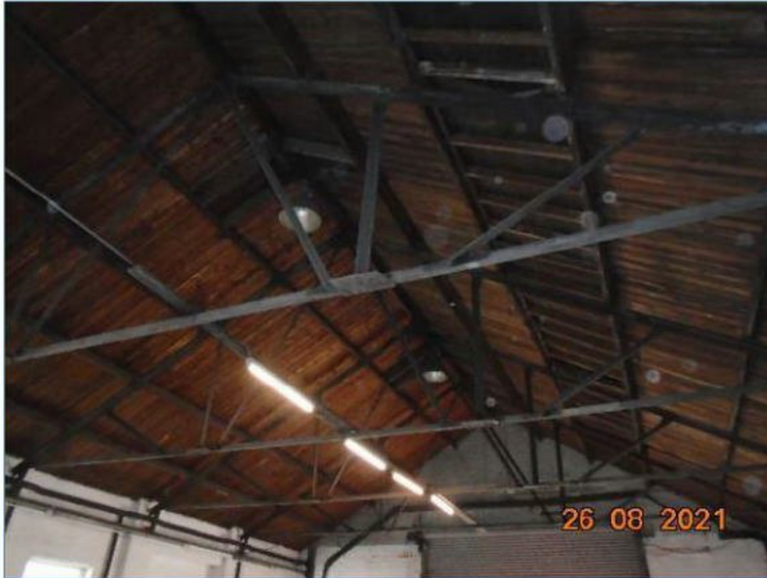
Photograph 17 – Building 1: Internal construction of western half of building.
