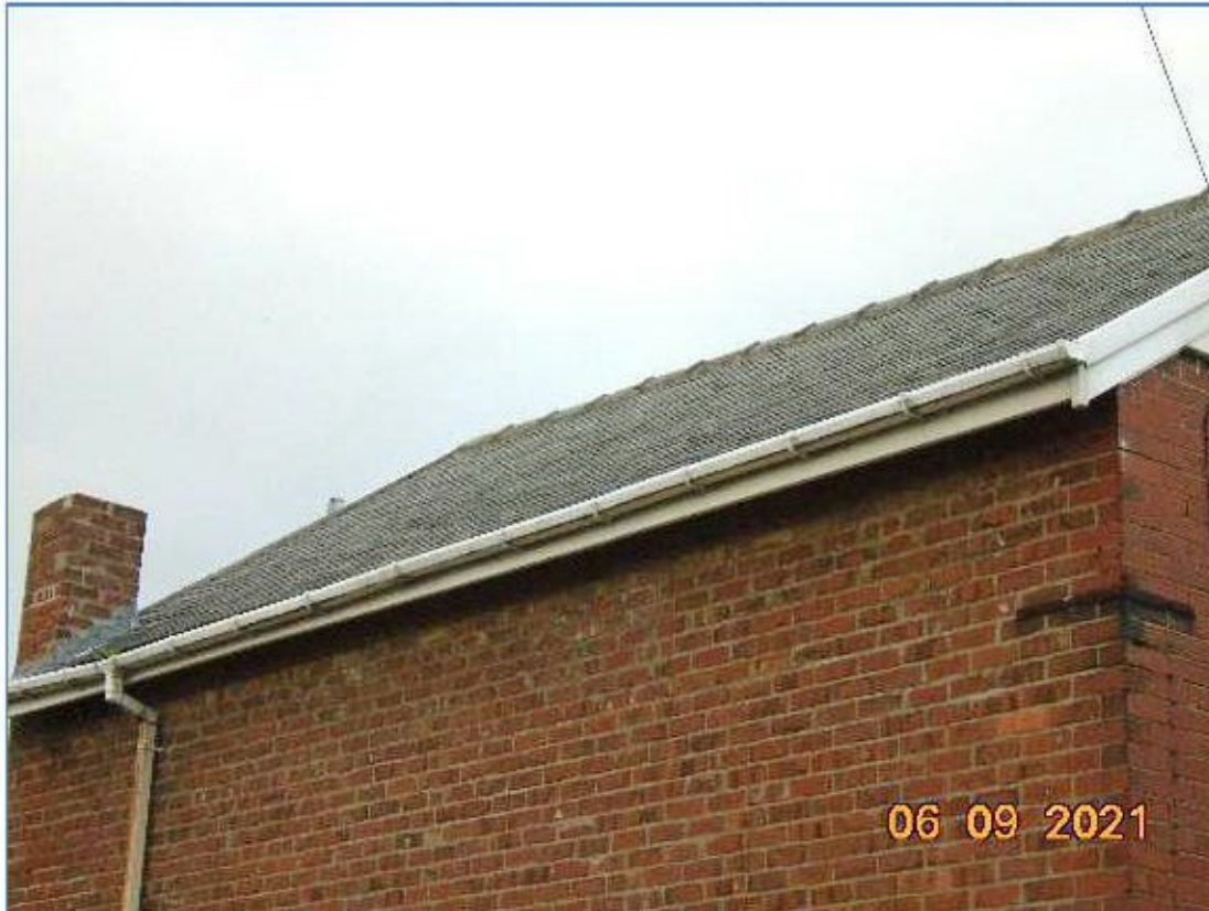
Photograph 18 – Building 2: Roof covering provides no potential bat access gaps.
