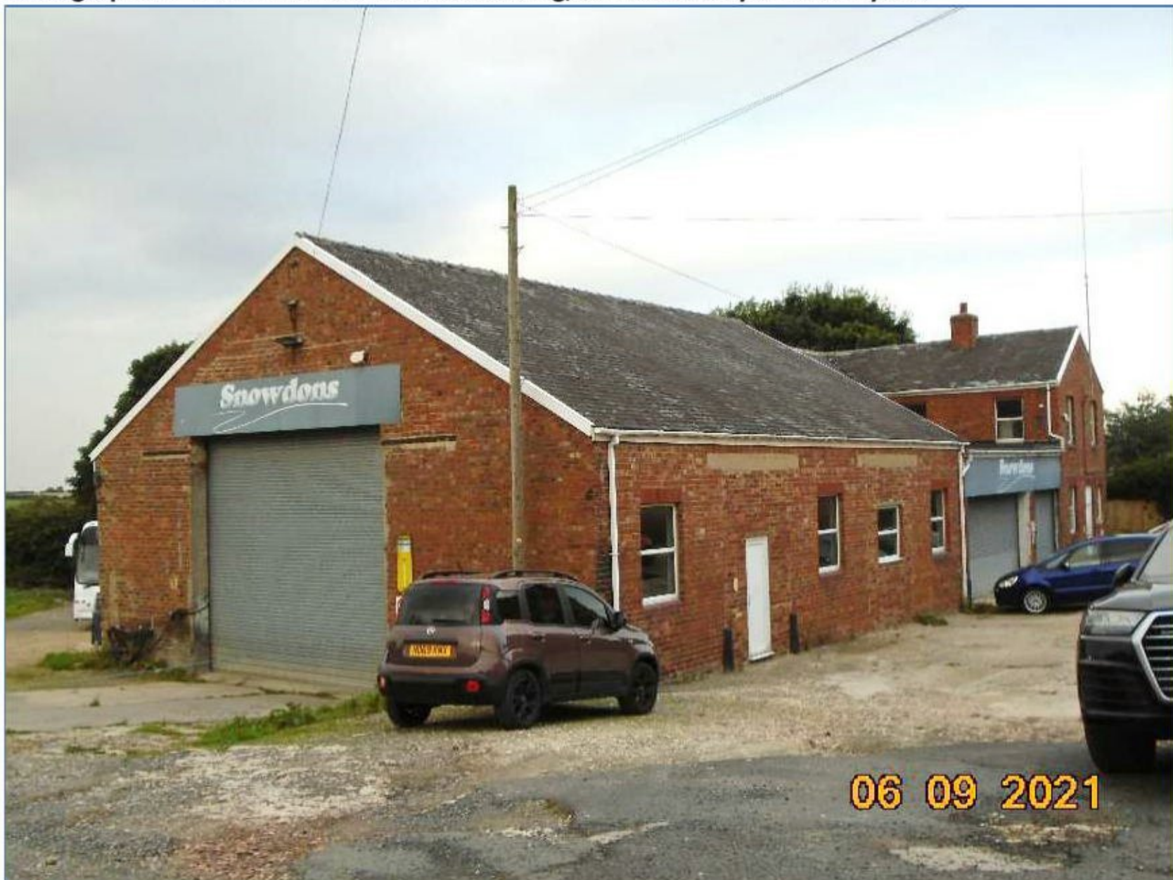
Photograph 10 – Coachworks and office building, surrounded by unsealed yard.
