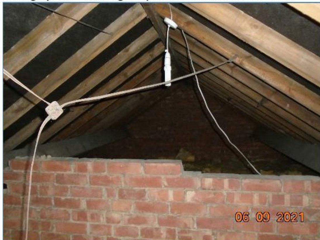
Photograph 22 – Building 2: Open and uncluttered roof void.
