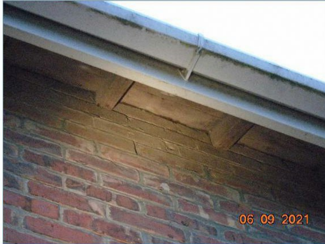
Photograph 20 – Building 2: No potential bat access gaps were noted at the eaves.
