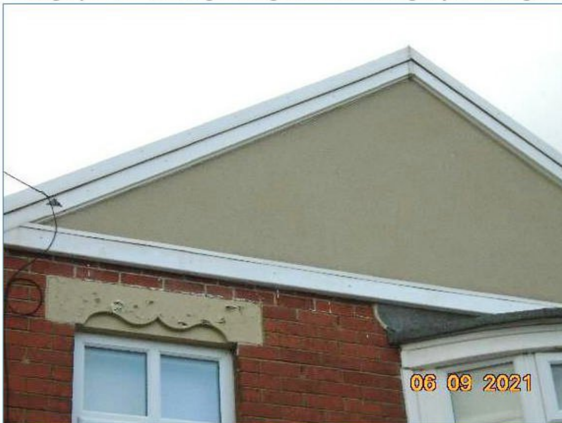
Photograph 19 – Building 2: Barge boards seal tightly to both gables.
