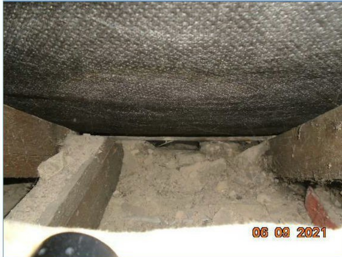
Photograph 21 – Building 2: Wall tops are sealed internally.
