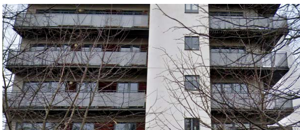
Blockwork with cementitious render direct onto blockwork
