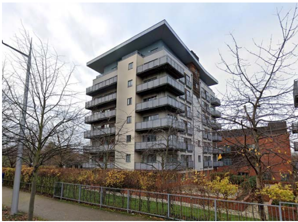
Elevation from Lakeside Drive
