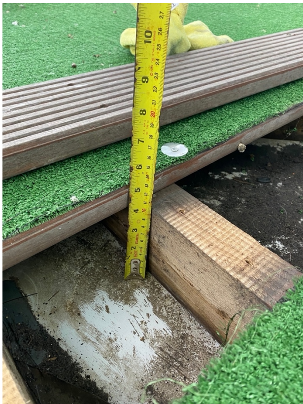
Timber Decking inspection
