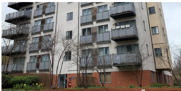
Front façade showing the brick work on the ground floor
