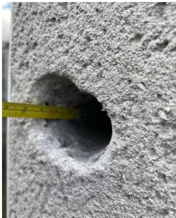
Zoomed in blockwork inspection hole
