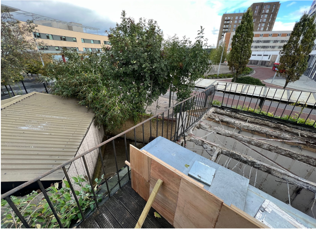
View from Balcony Level (post demolition) to rear of Application Building
