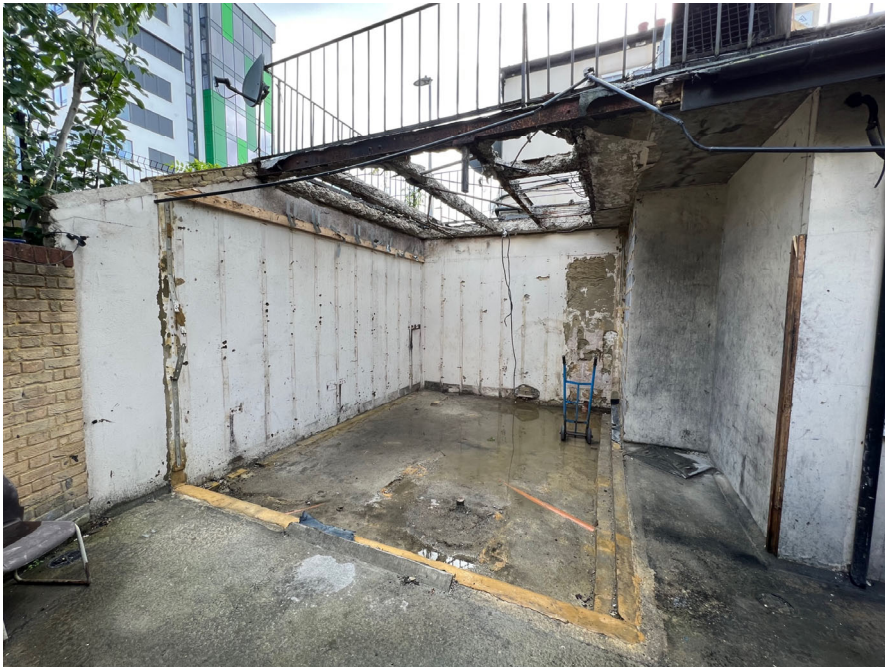
View of Studio No. 16 (post demolition) from ground level
