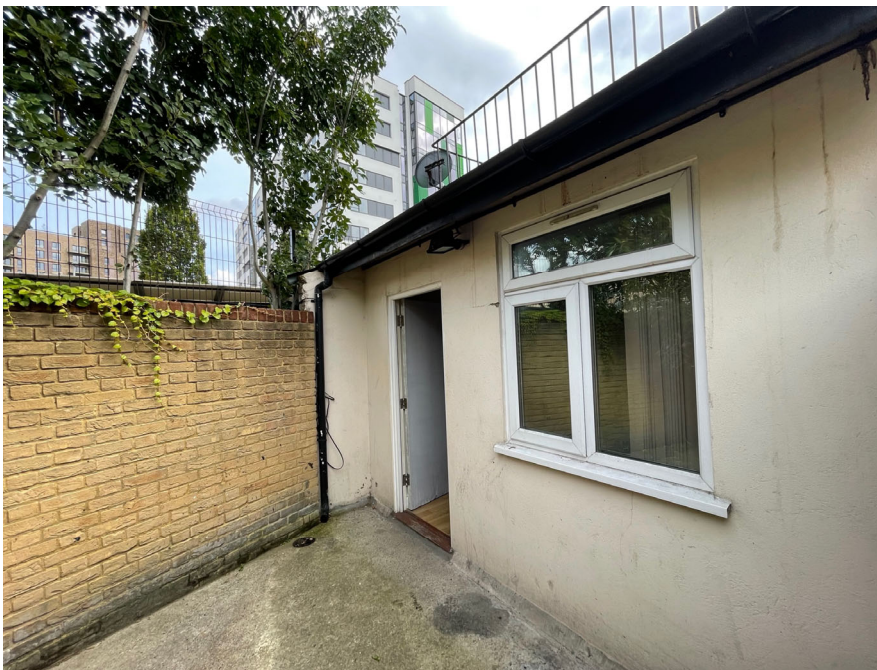
View of Studio No. 16 (prior to demolition) from ground level
