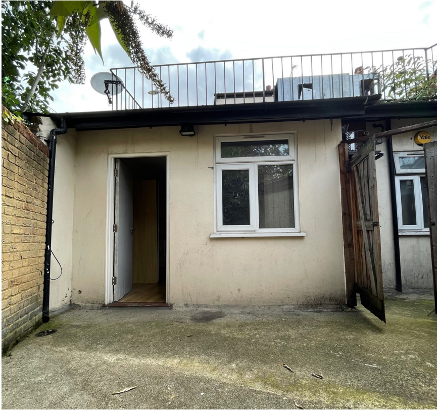
View of Studio No. 16 (prior to demolition) from ground level
