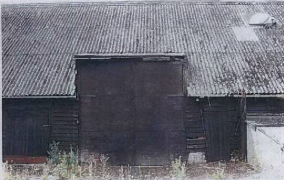
The double doors are LC20th marine ply replacements.
