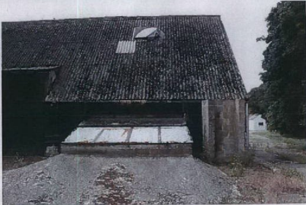
Concrete ramp and hopper to feed the pre-dresser.
