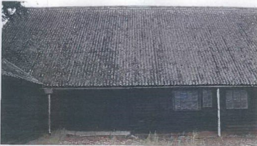
The eastern end of the northern elevation.
