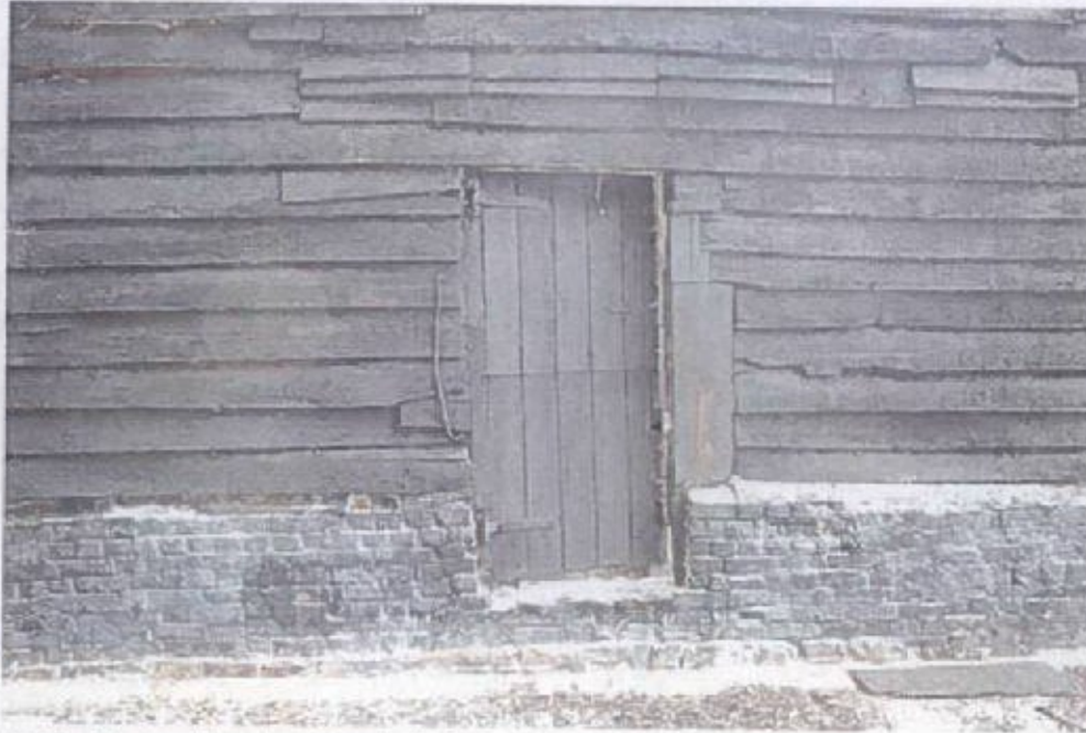
Detail of the weather-boards and plinth on the western elevation.
