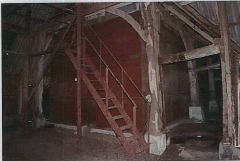
Truss 3 looking NE.
