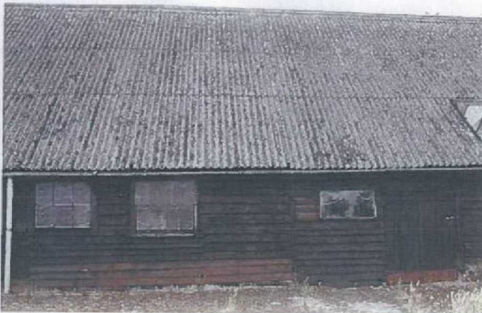
Detail of the C20th windows and C19th door.
