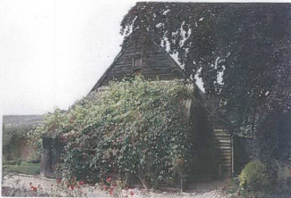
The eastern elevation of the Barn and Lean-to.
