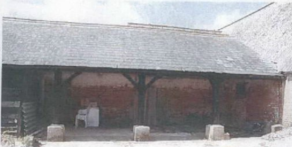
The open bays of Shelter 3.
