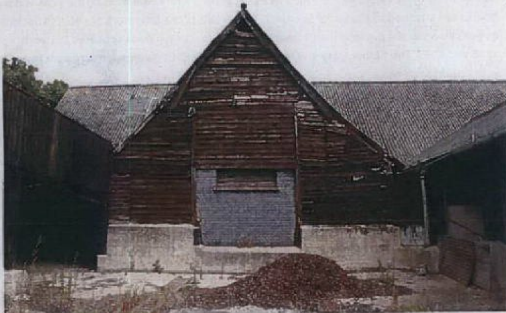
Looking N into the Western Farmyard. The midstrey porch of the Barn.
