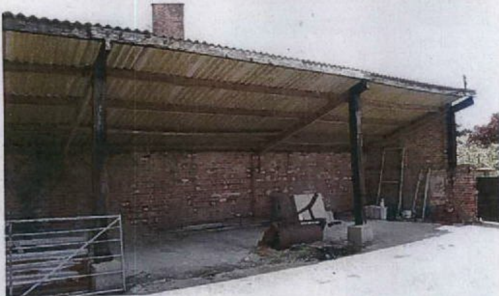
Looking ESE into Shelter 4.
