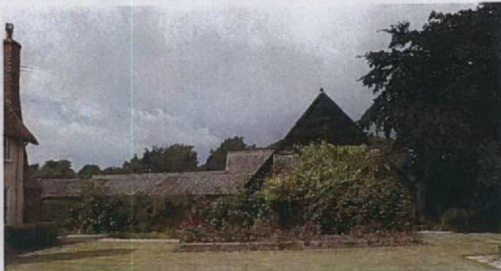
The eastern elevation from the garden.
