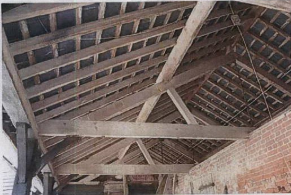
Looking NE inside Shelter 2.
