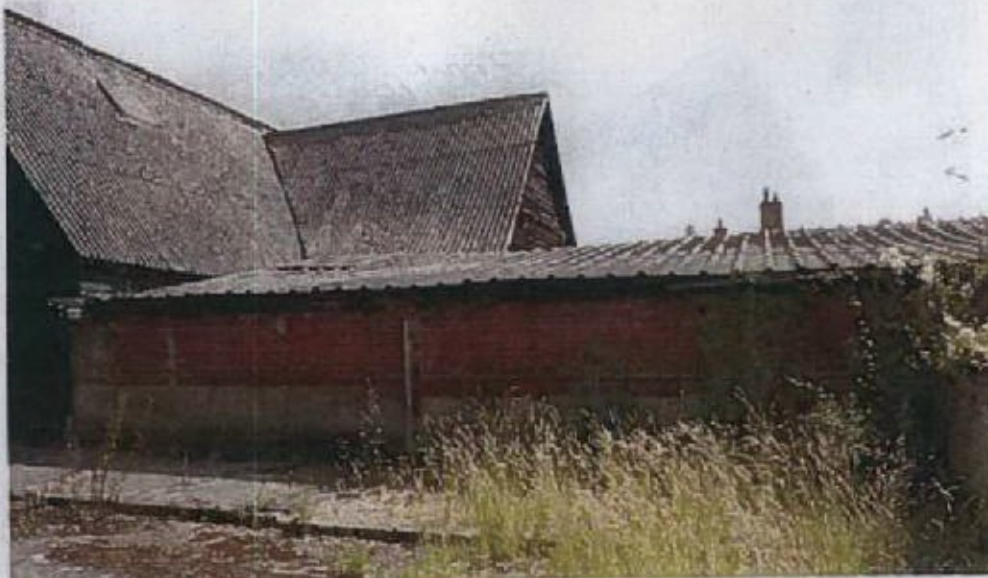
The western elevation of Shelter 1.
