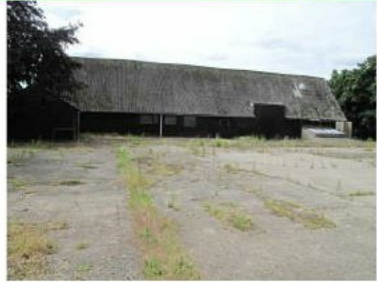
The listed timber barn, north elevation
