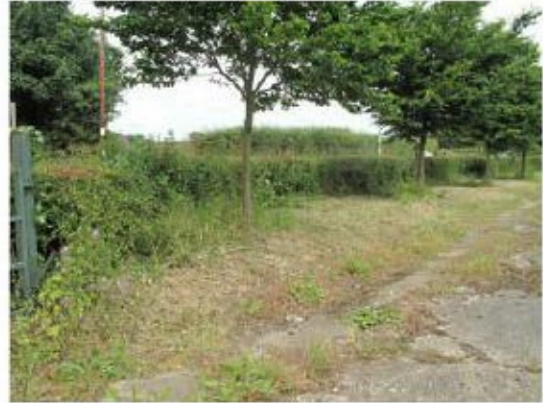
West boundary of the concrete yard
