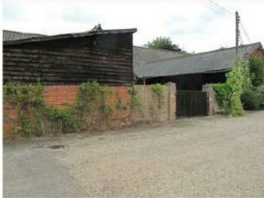
Southern elevation of the shelter sheds
