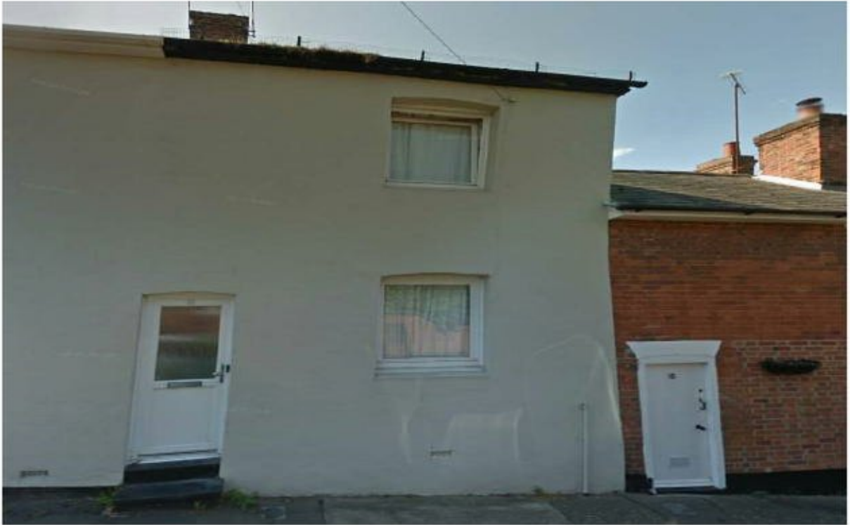
Fig. 2 – Front view from Brook Street
