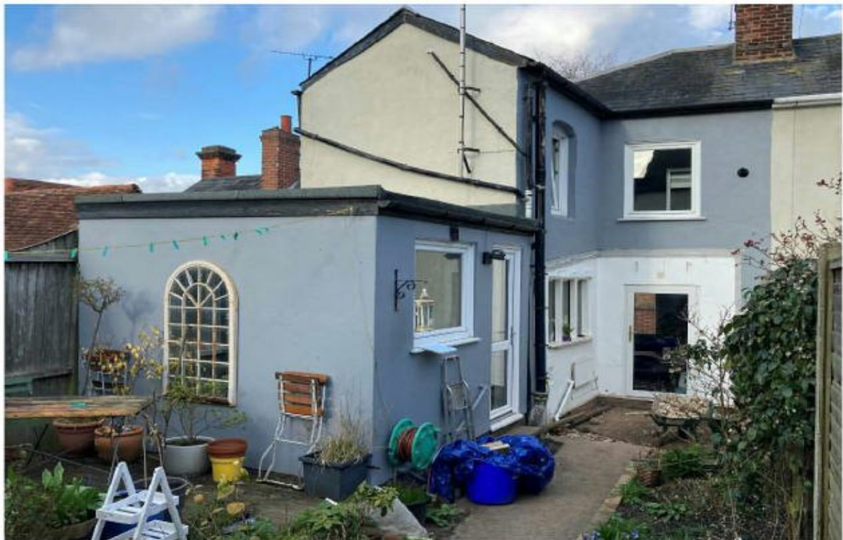
Fig. 3 – Rear view – proposal to be built above flat roof area in foreground.
