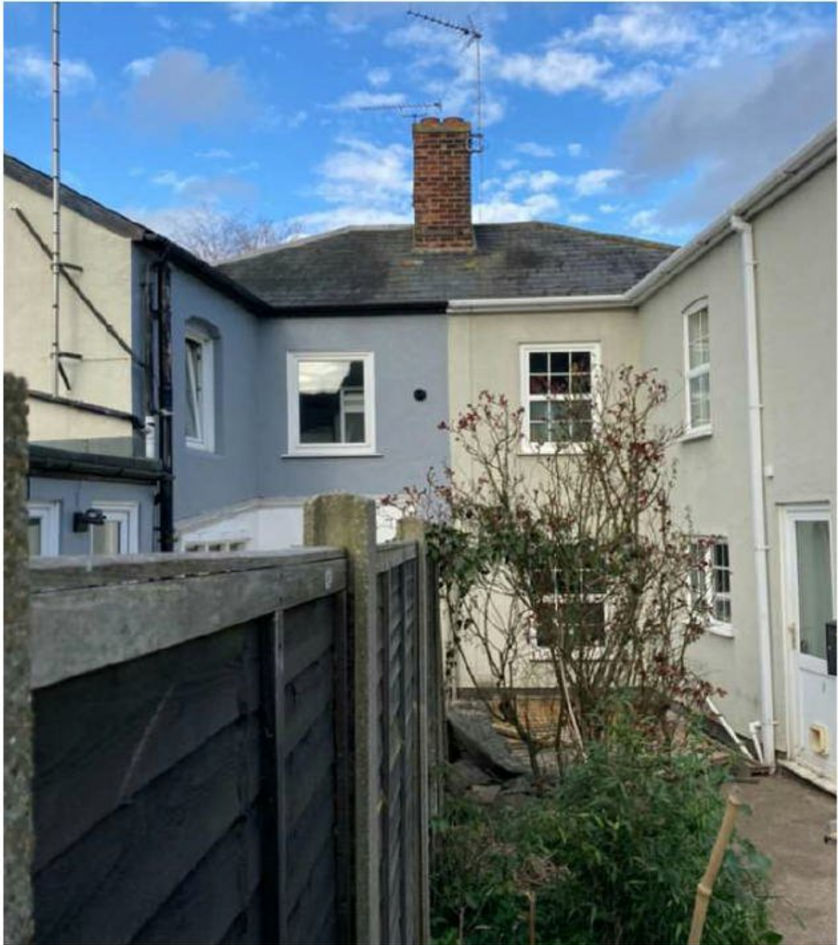
Fig. 4 – Rear view of 18 Brook Street & 2 Railway Street.
