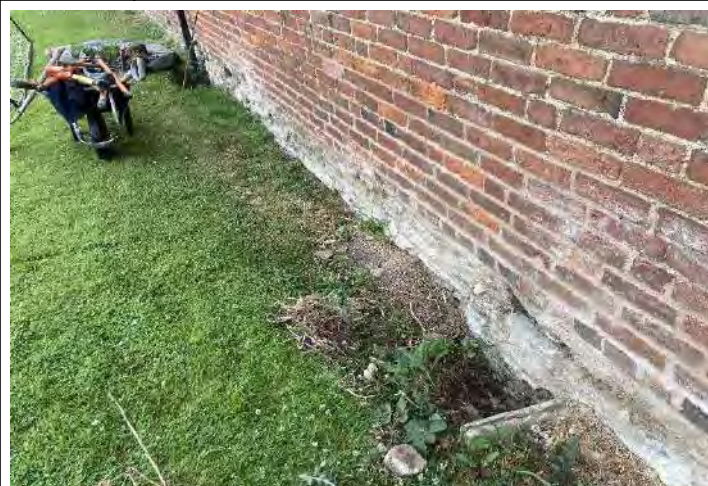
Plate 4 Line of gulley along E elevation of barn to drain.
