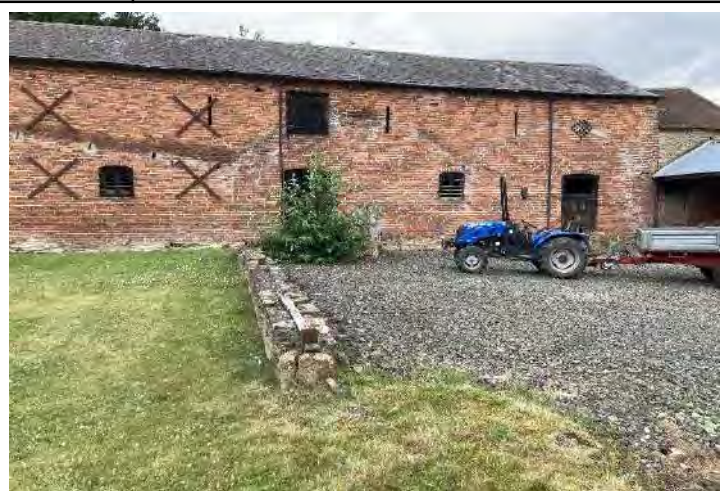
Plate 5 | Structural wall ties/bolts on E elevation of western limb, evidence of former agricultural structure (wall line & markings on E elevation).
