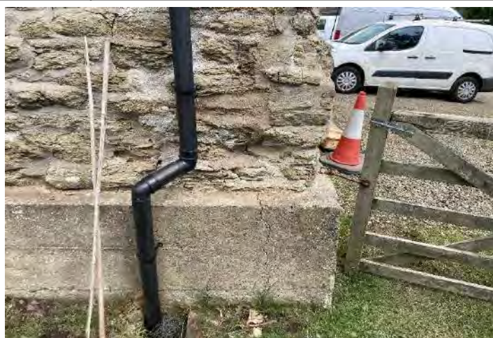
Plate 16 | Localised cracking within concrete.
