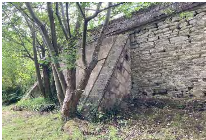
Plate 19 Proximity of trees to buttressed wall. Bedrock is visible at the base of the stonework.
