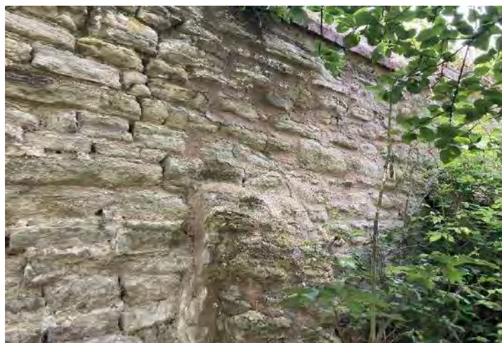
Plate 20 Localised repointing of stonework.
