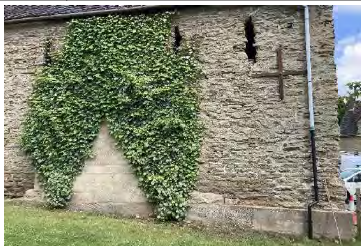
Plate 15 | Infilled opening (& concrete underpinning?) of E end of southern limb of barns.
