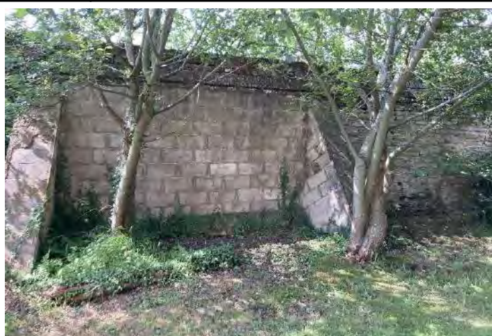
Plate 18 | Boundary wall to curtilage of 'Race House', with infilled opening between buttresses.
