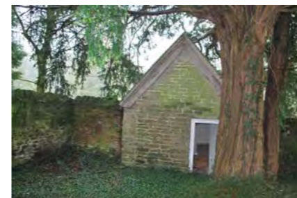
Photo 14. HOUSE KITCHEN & PATIO
