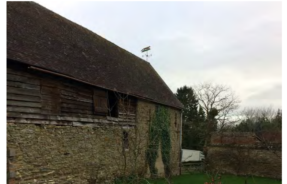
Photo 6. BARN 'A' - SOUTH-EAST END
