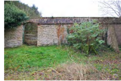
Photo 1B. GARDEN WALL TO THE SOUTH
