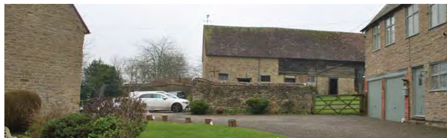
Photo 13. COURTYARD: NORTH ACCESS NEXT TO COACH HOUSE
