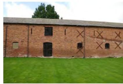
Photo 5. WEST: BARN 'C'
