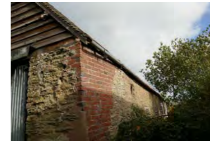
Photo 5A. BARN 'B' - SOUTH-WEST END
