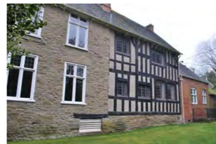
Photo 13. HOUSE KITCHEN & PATIO
