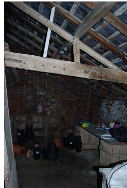
Photo 1B. POTTING SHED - INTERIOR
