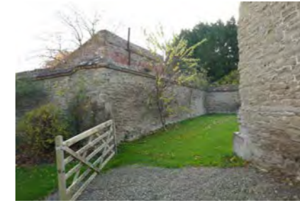
Photo 2. EAST ACCESS BETWEEN BARN 'A' & WALLED GARDEN
