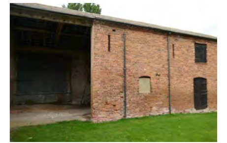
Photo 4. WEST: BARN 'C'
