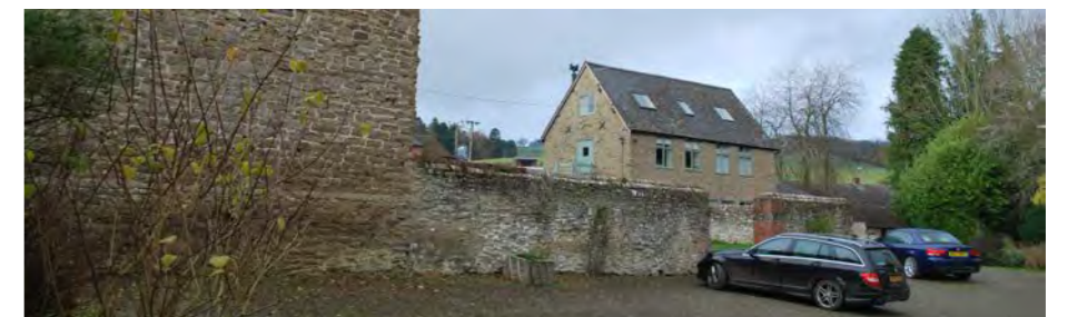
Photo 15. COURTYARD: EAST ACCESS FACING MAIN DRIVE & HALL
