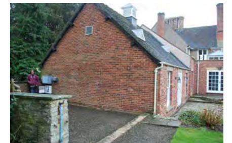
Photo 13. AREA IN BETWEEN NORTH GATE & KITCHEN
