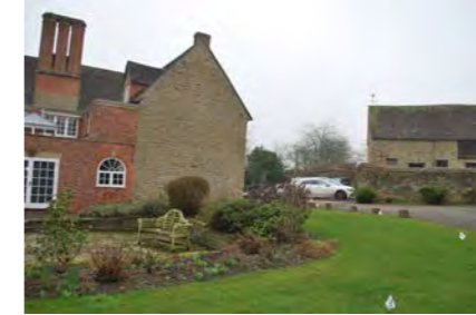
Photo 3. HOUSE WEST SIDE & COURTYARD TO THE WEST
