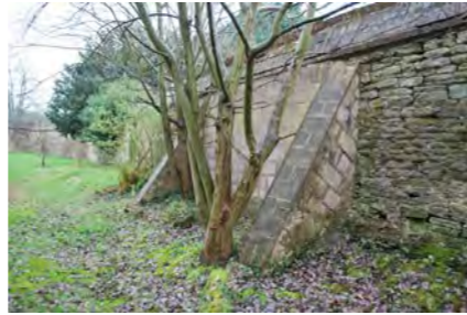
Photo 1A. GARDEN WALL TO THE SOUTH
