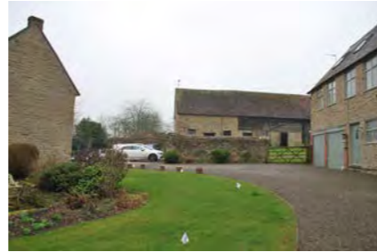
Photo 4. AREA IN BETWEEN HALL, COURTYARD & COACH HOUSE
