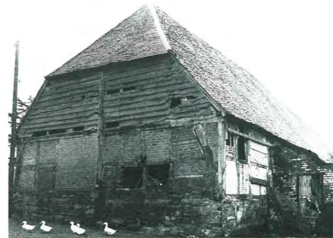
POOL BARN - LOCAL EXAMPLE FOR THE GREEN OAK FRAME MEDIEVAL CRUCK BLADES - LEIGH HEREFORD & WORCESTER
