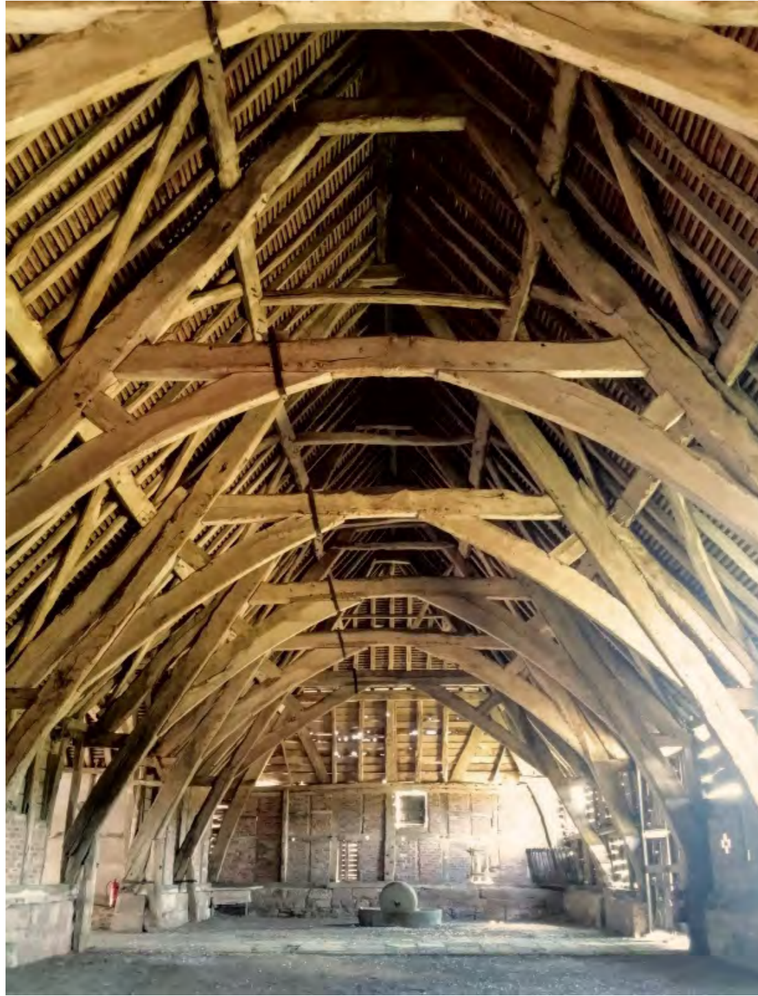
POOL BARN - LOCAL EXAMPLE FOR THE GREEN OAK FRAME MEDIEVAL CRUCK BLADES - LEIGH HEREFORD & WORCESTER
