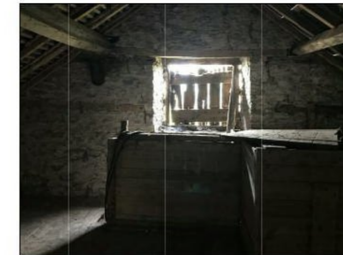
34 Remove timber partitioning.
