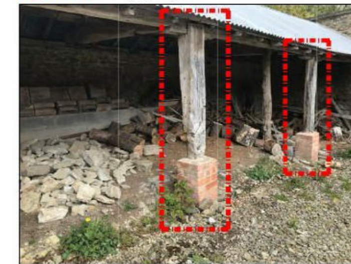
15 Remove timber propping to reinstate brick columns.
