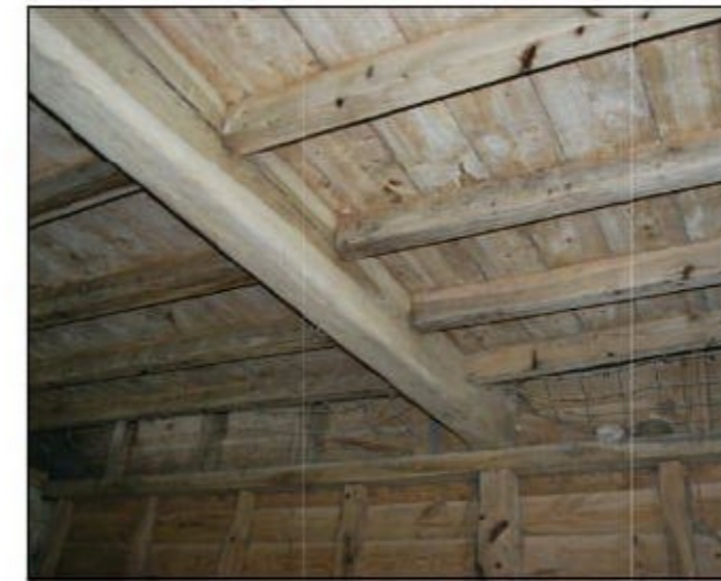
24 Rebuild modern timber floor.
