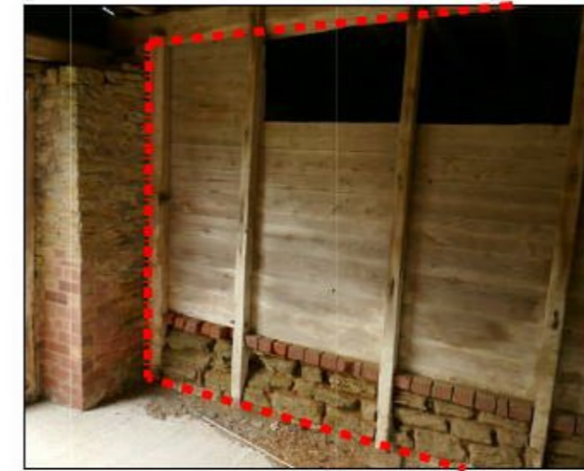
07 Remove modern stud partition & brick/stone plinth.
