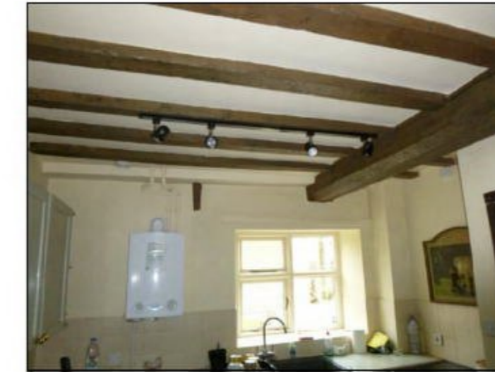
18 Remove internal partition and strip out kitchen to create accessible accommodation at GF.
