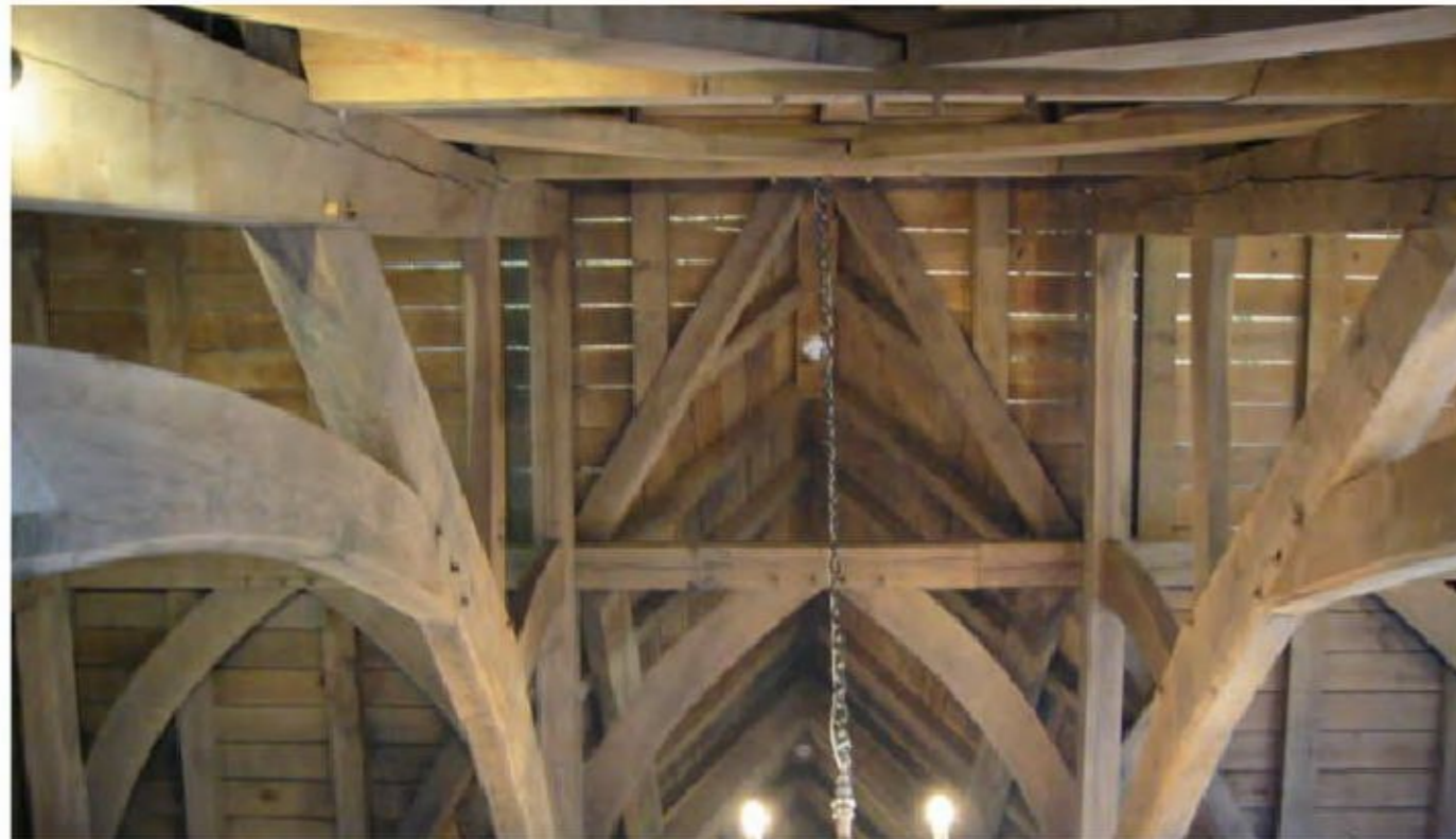
New Green Oak dining room roof.
