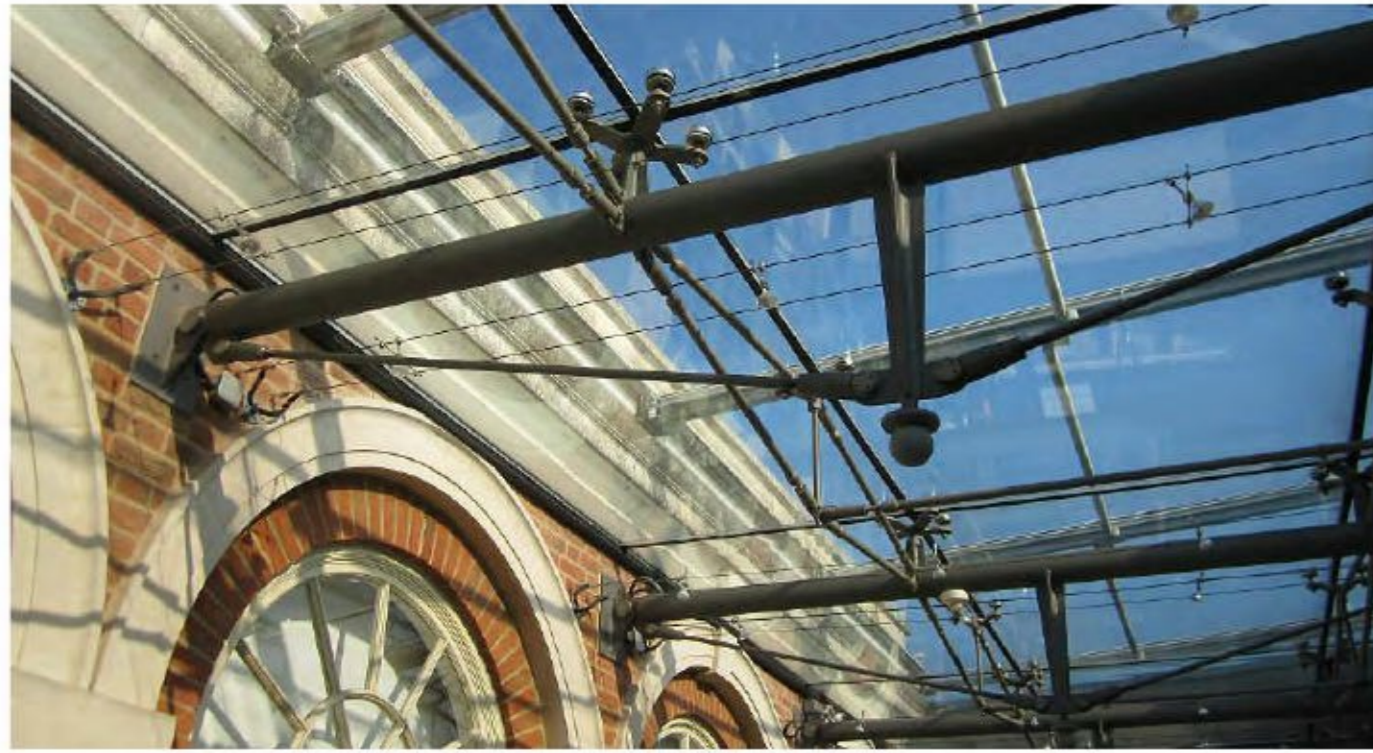
Glazing to conservatory.
