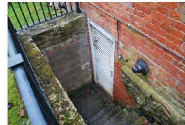
Photo 12. HOUSE KITCHEN & PATIO
