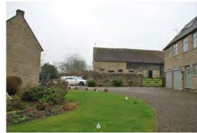
Photo 4. AREA IN BETWEEN HALL, COURTYARD & COACH HOUSE
