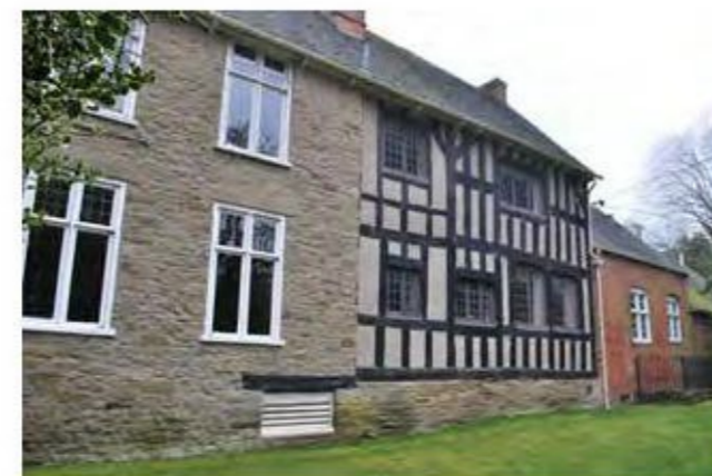
Photo 13. HOUSE KITCHEN & PATIO
