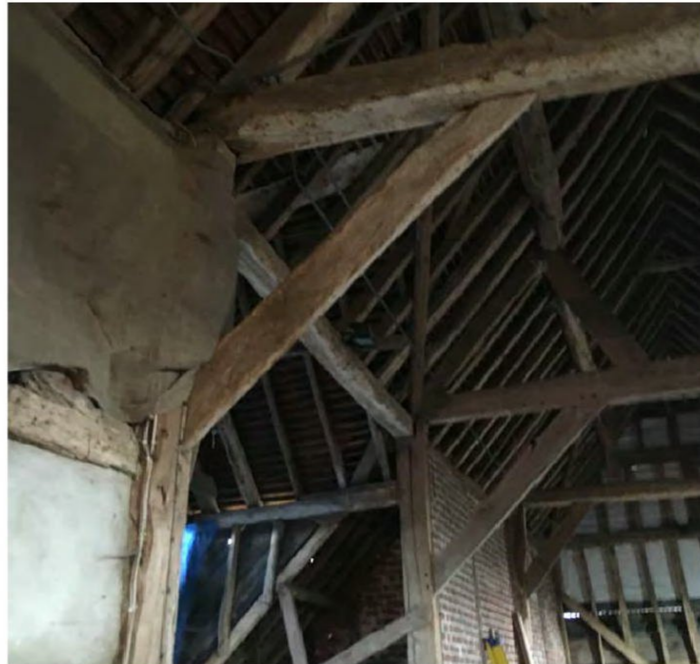
Purlin supporting truss.
