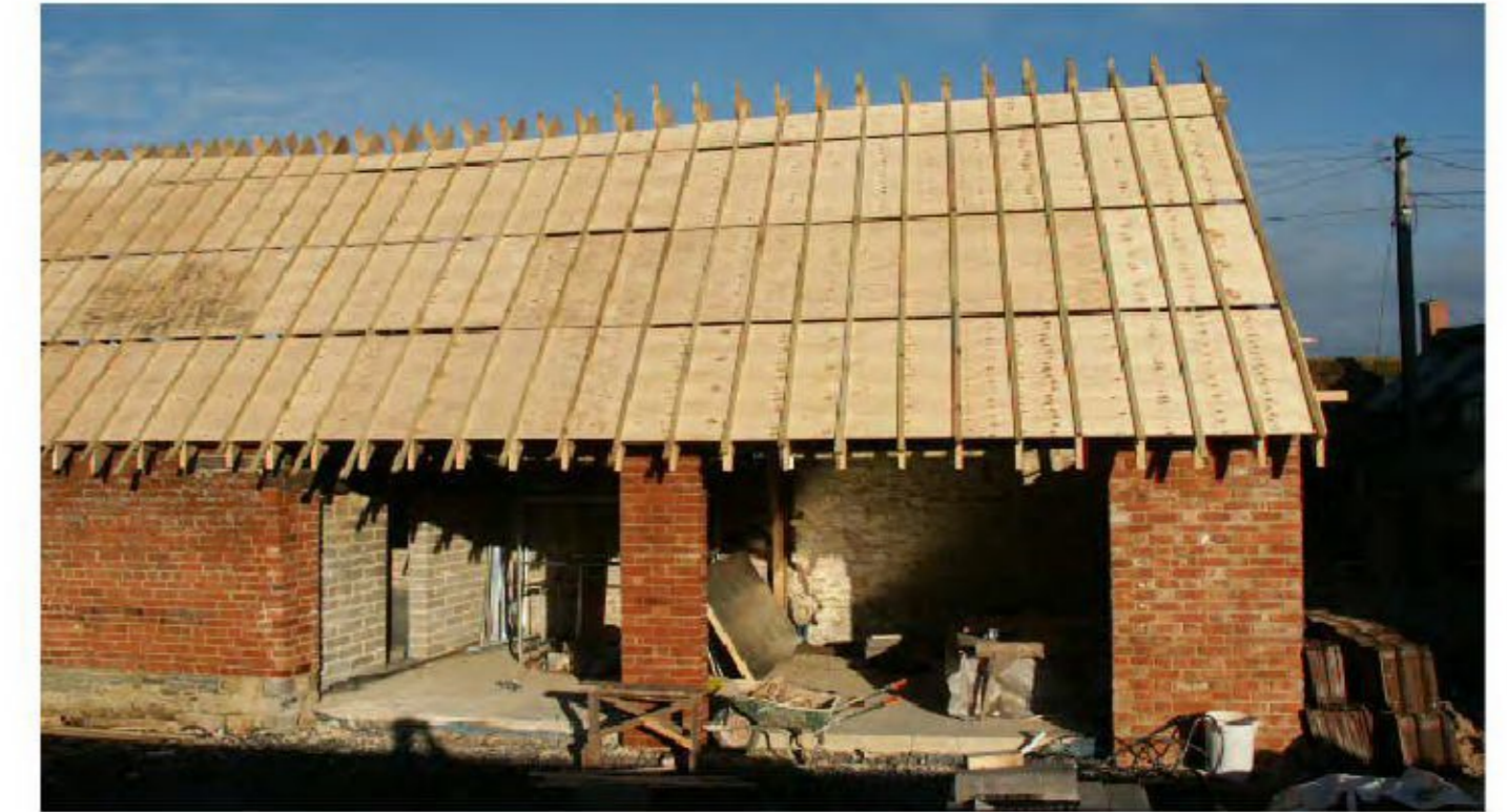
Adjoining barn mid restoration.
