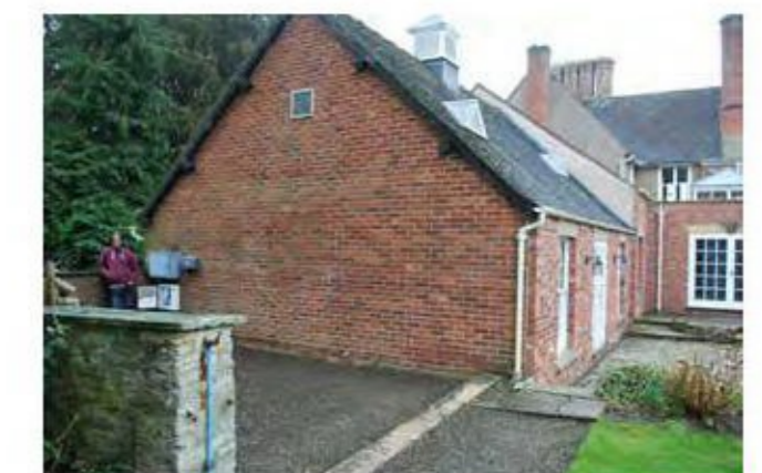
Photo 13. AREA IN BETWEEN NORTH GATE & KITCHEN
