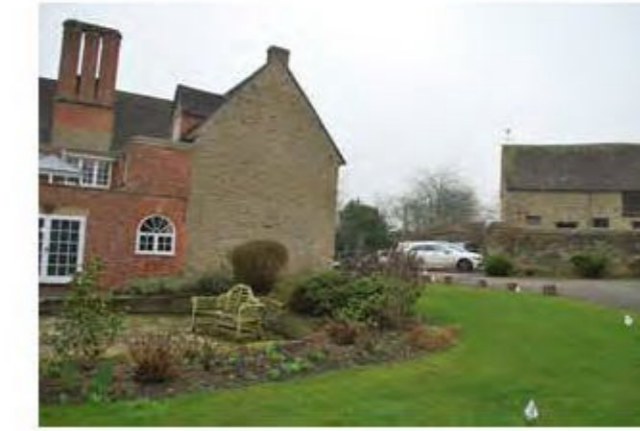
Photo 3. HOUSE WEST SIDE & COURTYARD TO THE WEST
