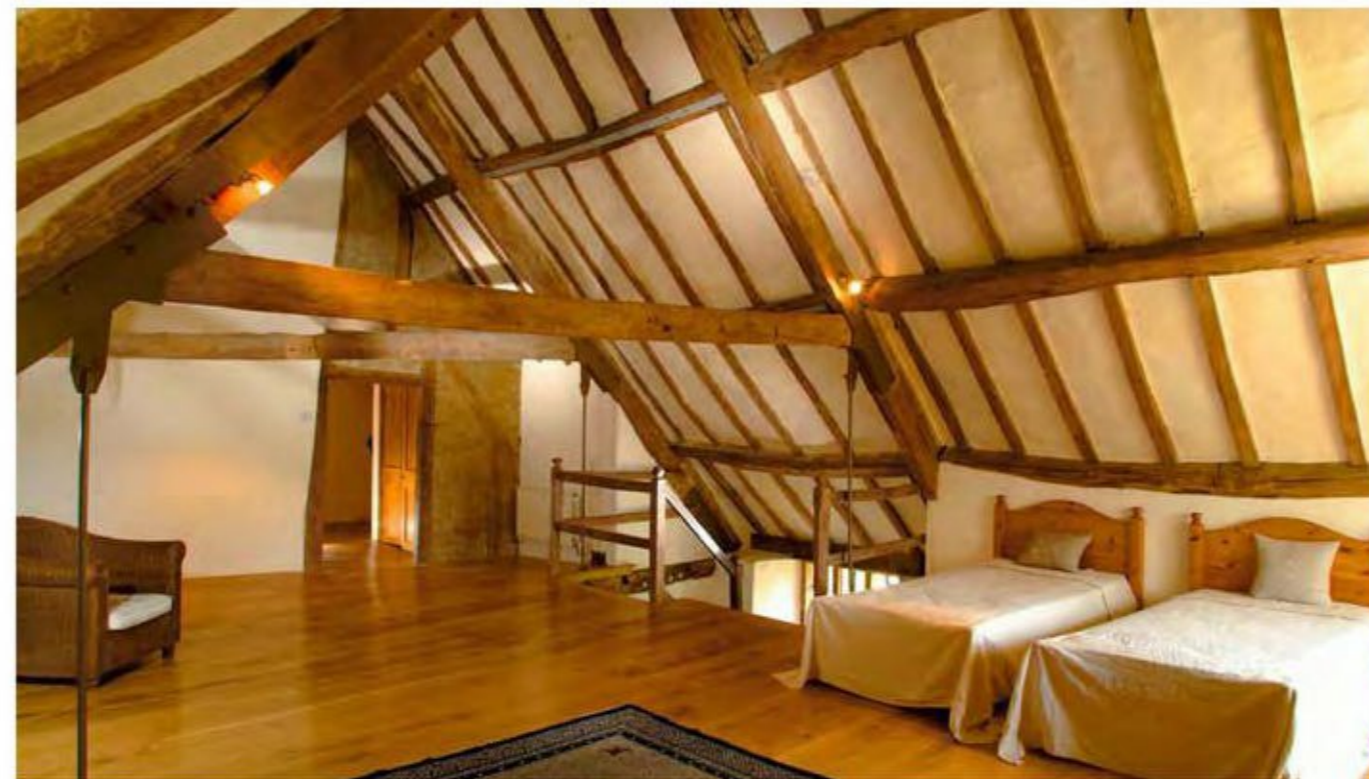
Steel hangers in attic of the house.
