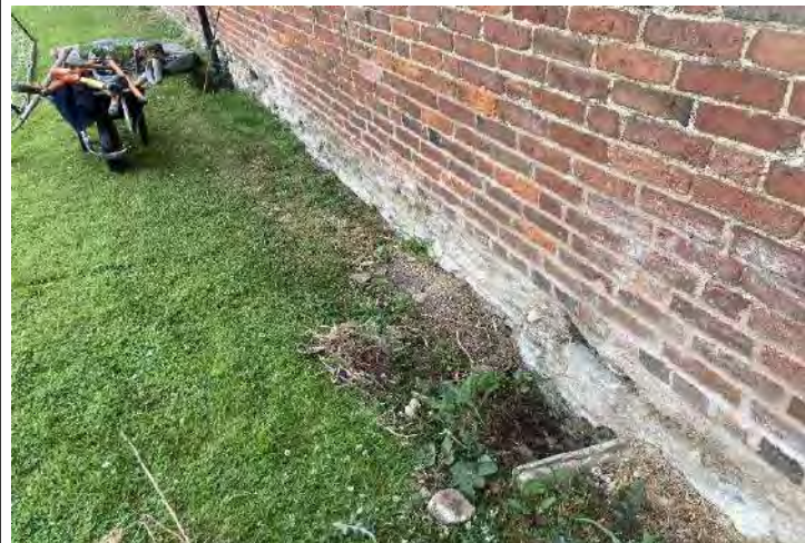
Plate 4 | Line of gully along E elevation of barn to drain.
