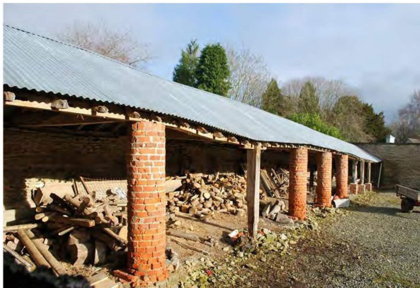
Photo 1. MAIN ELEVATION ALONG COURTYARD
