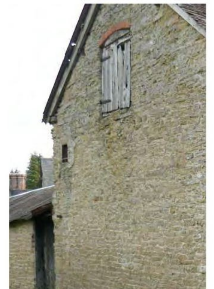
Photo 12. BARN 'D' - NORTH ELEVATION LOFT OPENING
