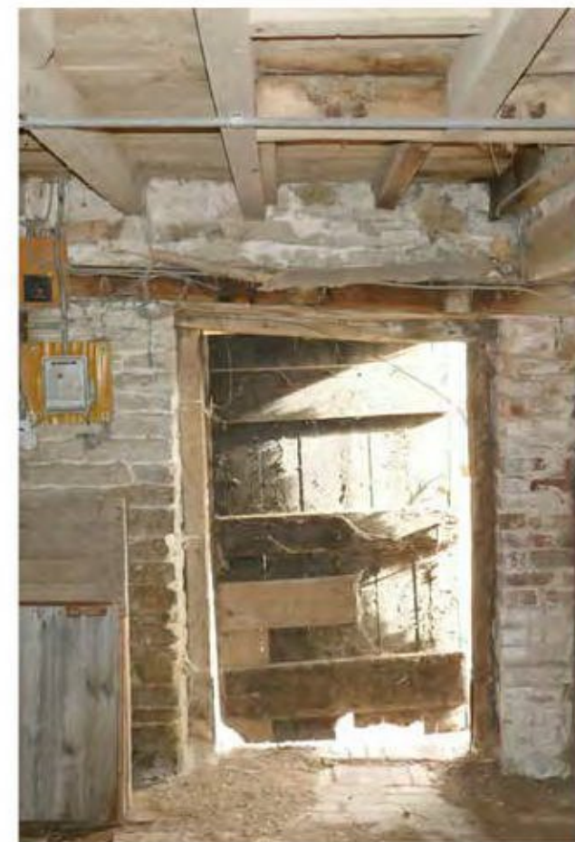
Photo 10. BARN 'D' - WEST ELEVATION ACCESS TO OTHER PROPERTY
