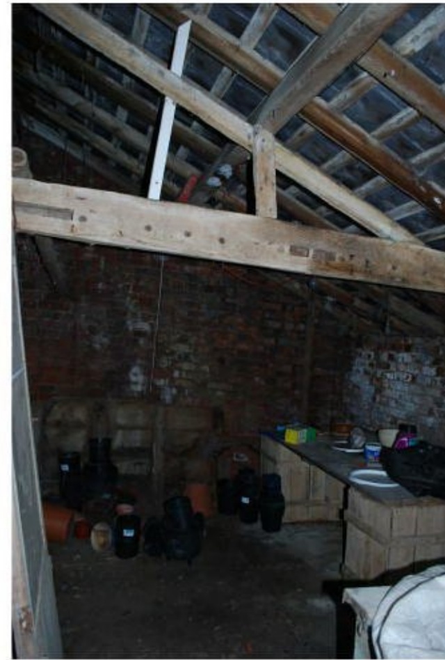
Photo 1B. POTTING SHED - INTERIOR
