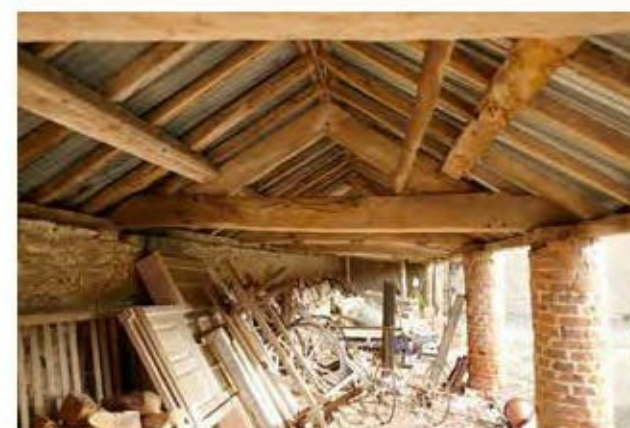
Photo 3. OPEN BARN ROOF
