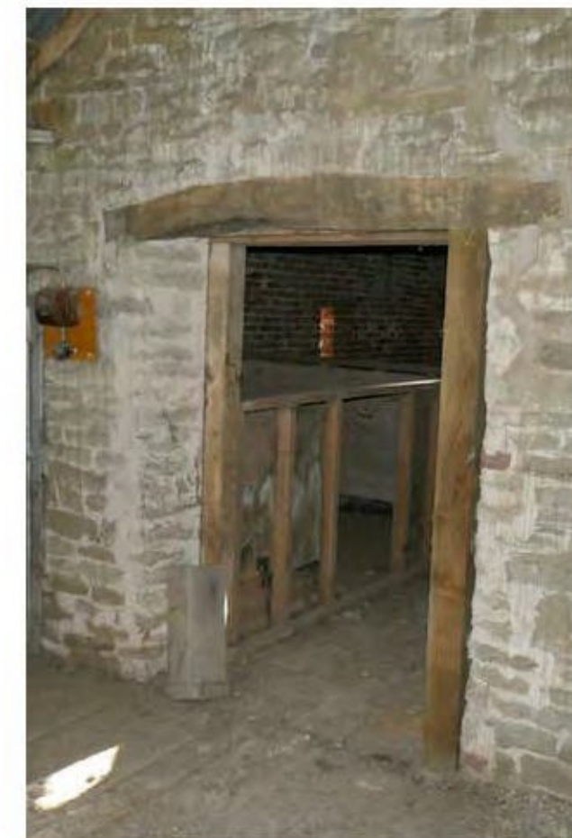
Photo 11. BARN 'C' & 'D' - 1ST FLOOR PASSAGE THROUGH
