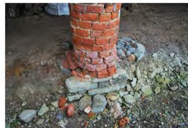
Photo 2. BRICK COLUMN DETAIL
