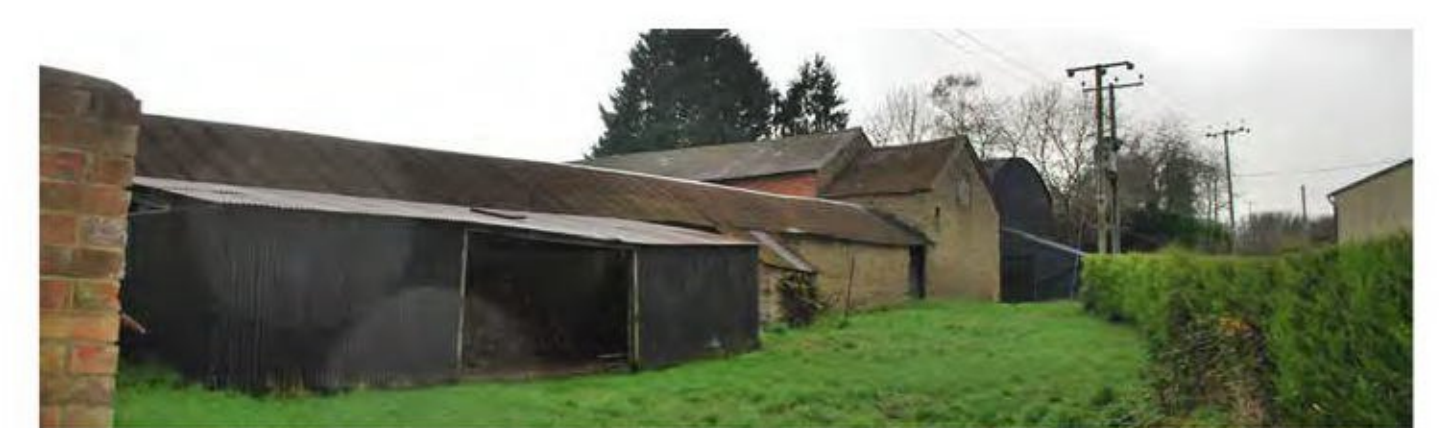
Photo 7. BACK ELEVATION FACING OTHER PROPERTY
