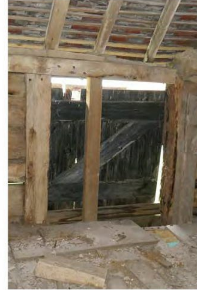
Photo 4. BARN 'A' - SOUTH ELEVATION LOFT ACCESS
