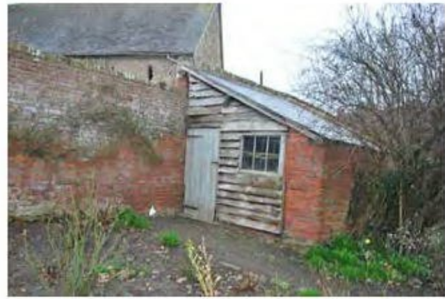
Photo 1A. POTTING SHED
