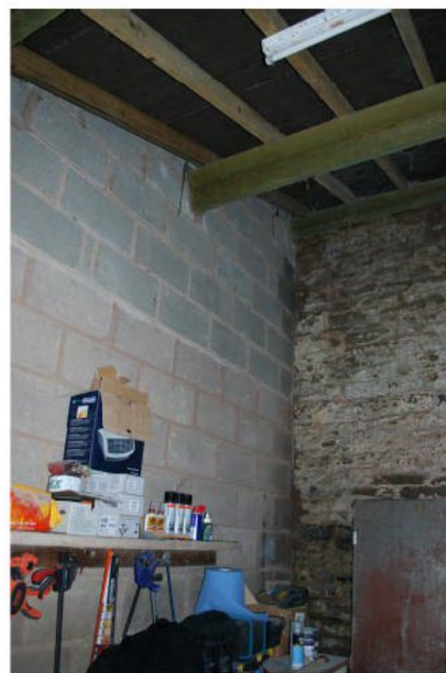
Photo 3B. NORTH UNIT - INTERIOR
