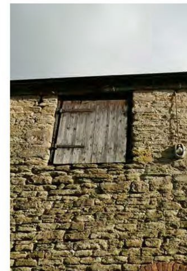
Photo 11. BARN 'C' - WEST ELEVATION LOFT OPENING
