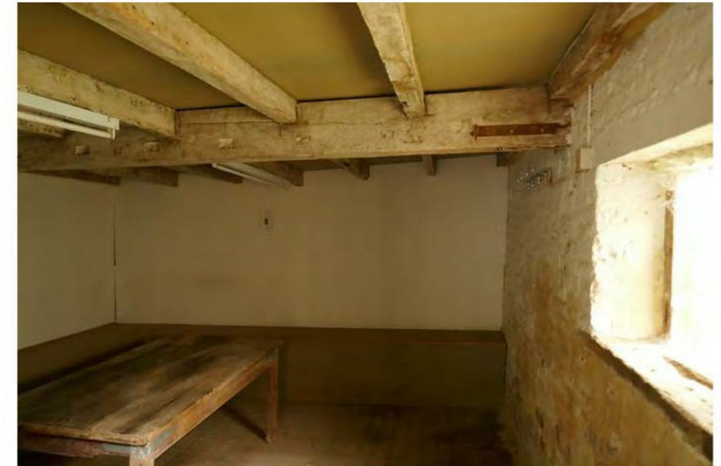
Photo 9. BARN 'C' - GROUND FLOOR CONVERTED OFFICE / TEA ROOM
