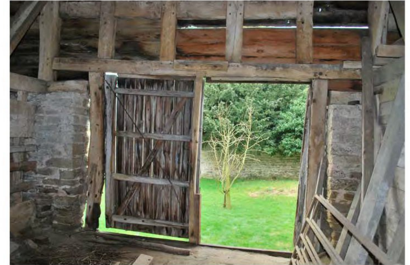
Photo 3. BARN 'A' - CENTRAL PASSAGE (GF) THRESHING BARN CONSERVING DOUBLE HEIGHT SPACE
