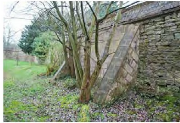
Photo 1A. GARDEN WALL TO THE SOUTH
