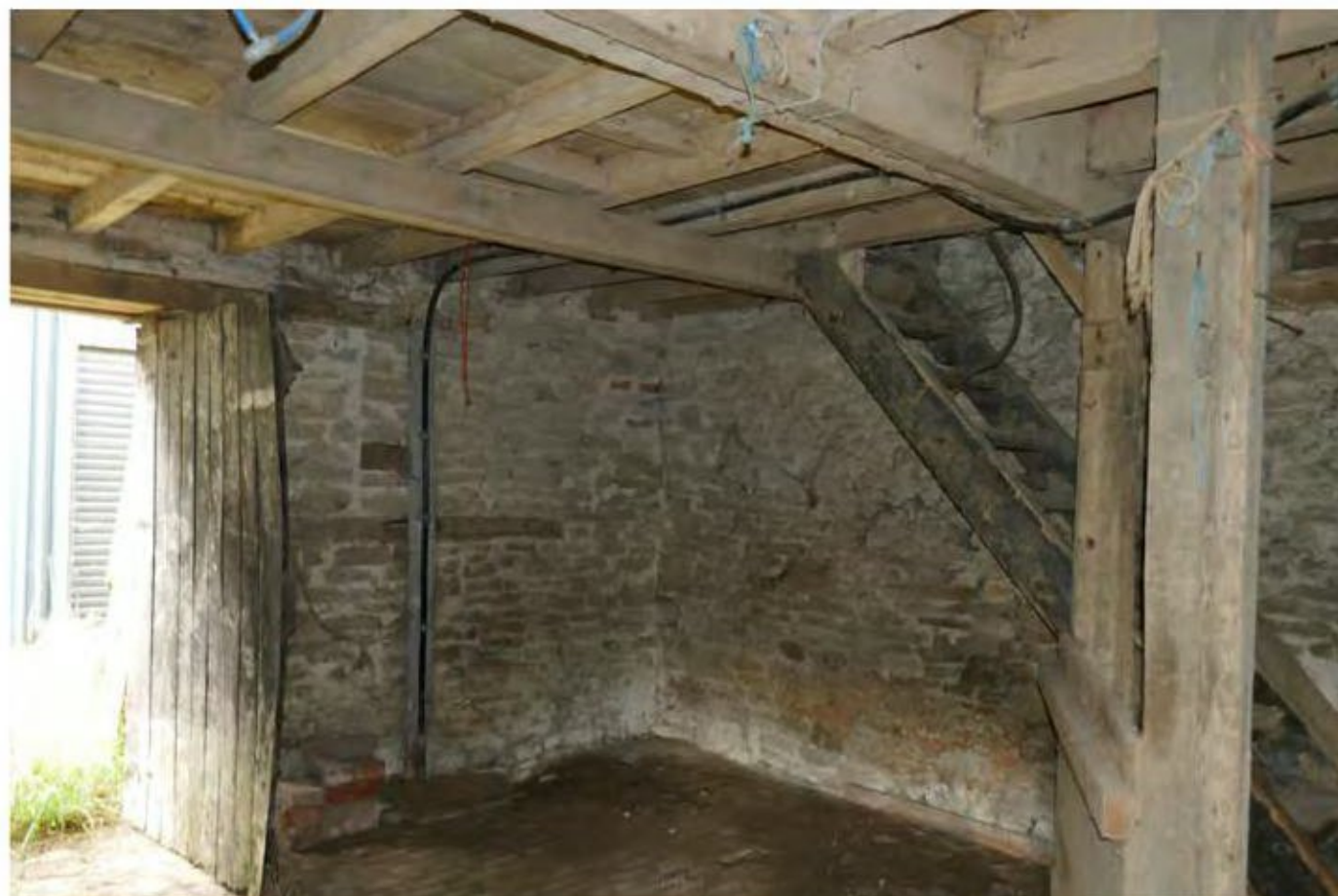
Photo 10. BARN 'D' - GF PASSAGE TO OTHER PROPERTY BARN & ACCESS TO LOFT
