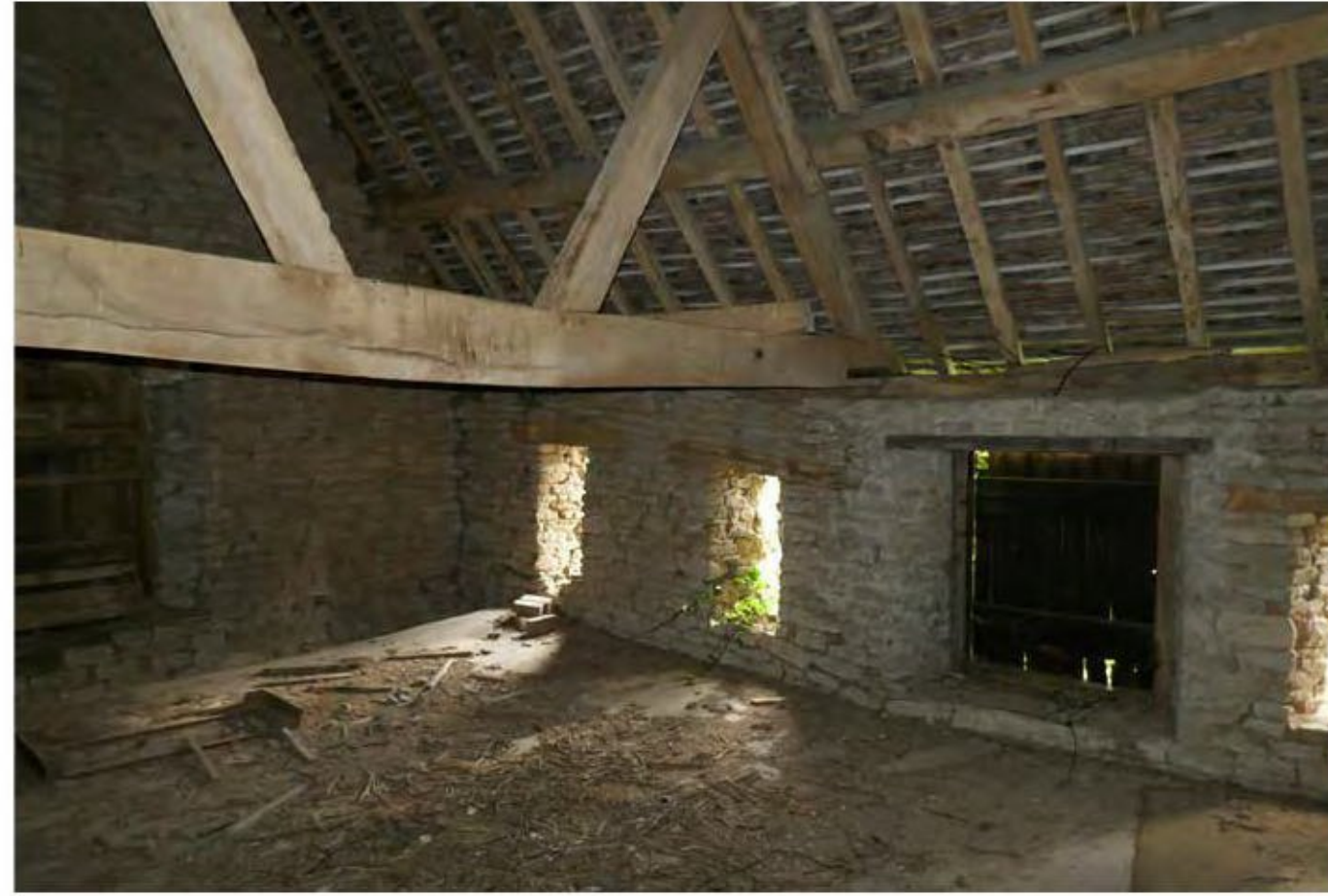
Photo 2. BARN 'A' - SOUTH-EAST CORNER (1F) STONE END BUILDING
