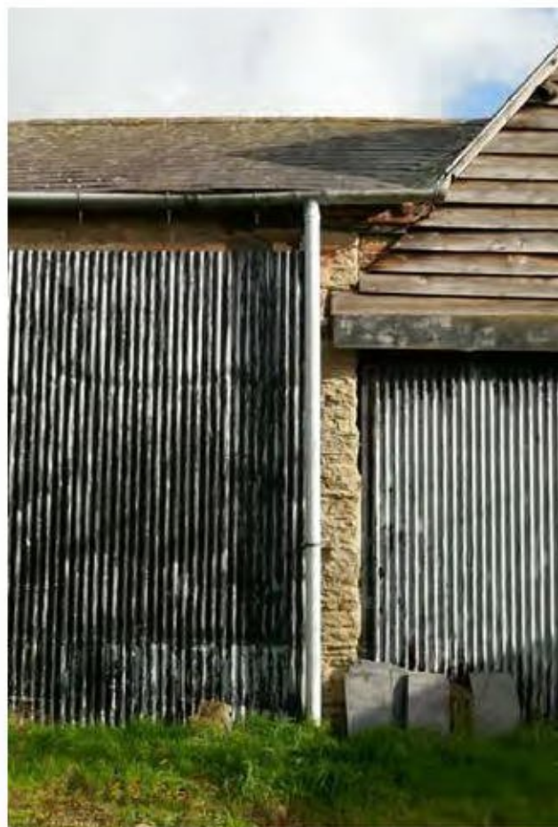
Photo 8. BARN 'B' & 'C' - WEST ELEV. CORRUGATED IRON DOORS
