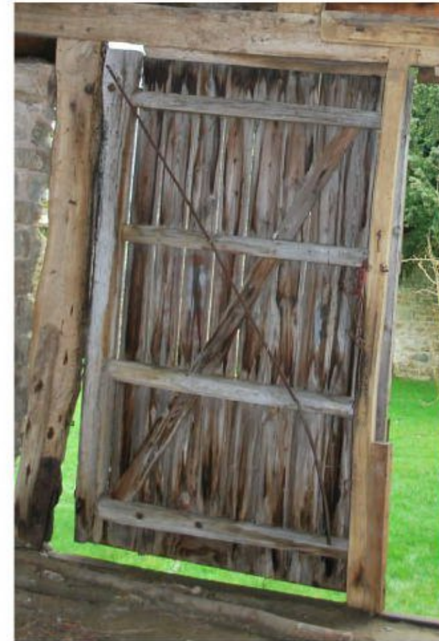
Photo 4. BARN 'A' - SOUTH ELEVATION THRESHING BARN
