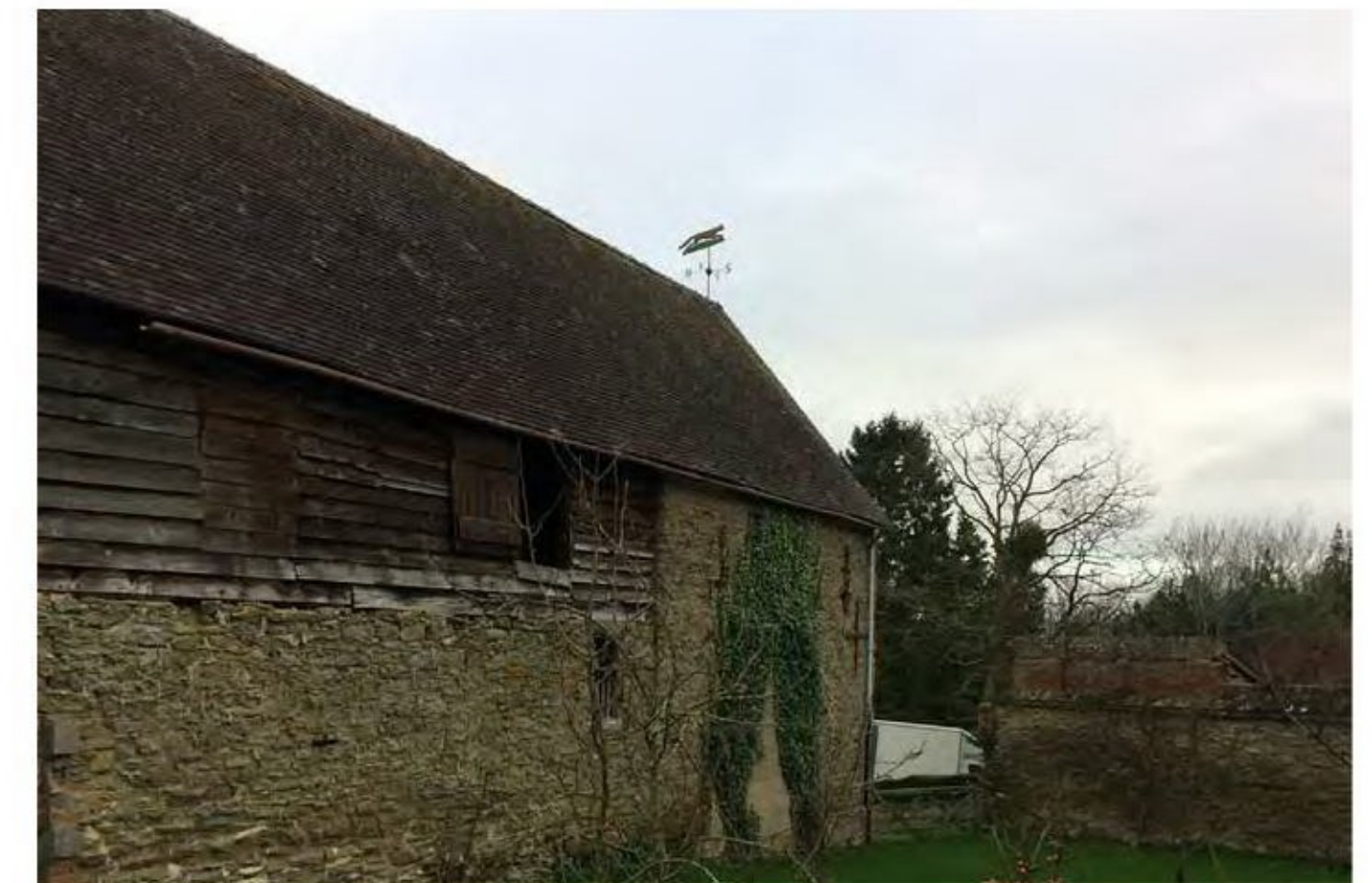
Photo 6. BARN 'A' - SOUTH-EAST END
