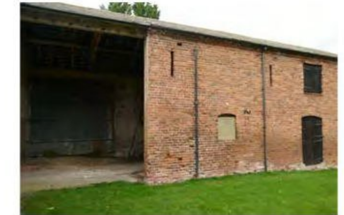
Photo 4. WEST: BARN 'C'
