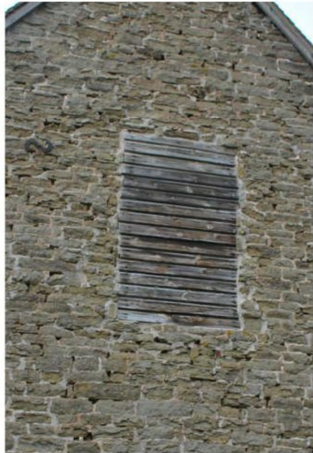
Photo 1. BARN 'A' - EAST ELEVATION LOFT OPENING
