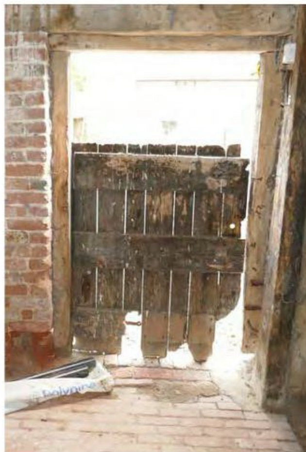
Photo 9. BARN 'C' - EAST ELEVATION STABLE DOOR
