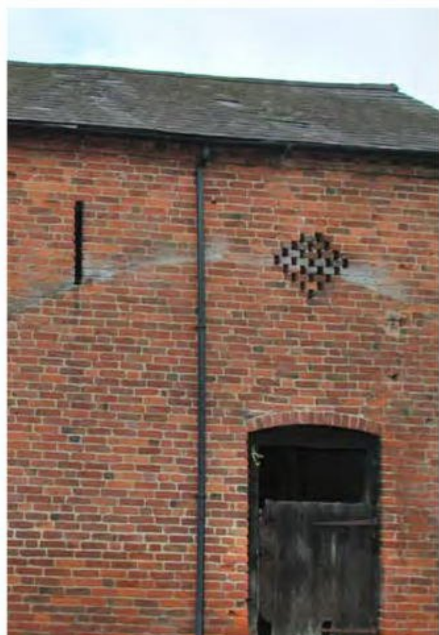
Photo 7. BARN 'C' - EAST ELEVATION SLITS & BRICK VENTS
