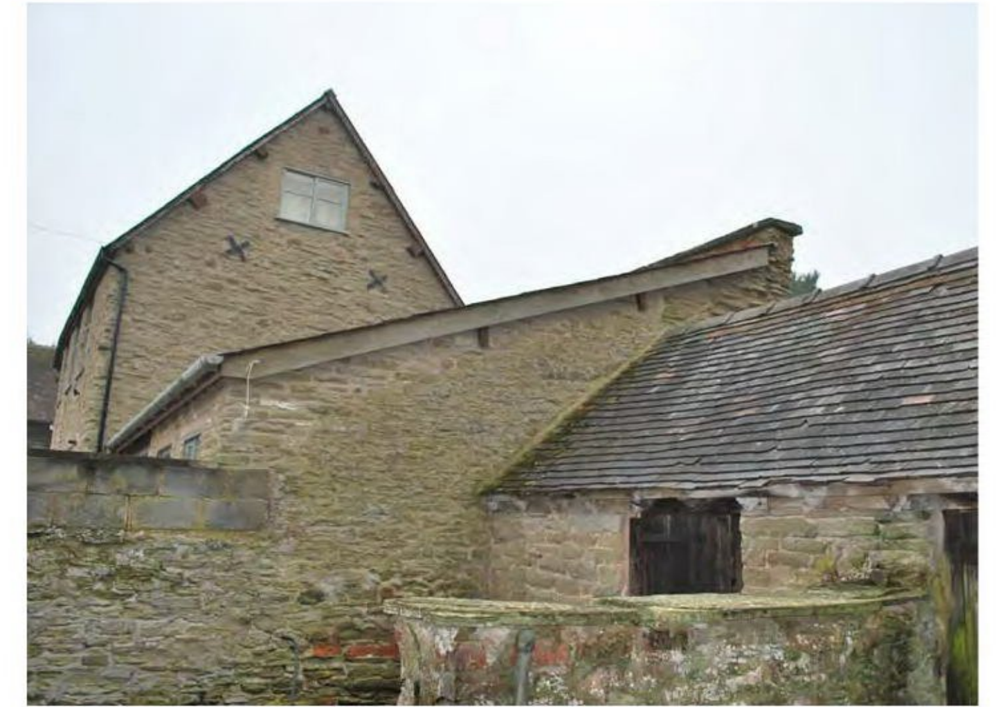
Photo 4. NORTH ELEVATION & DOG KENNELS TO NORTH SIDE
