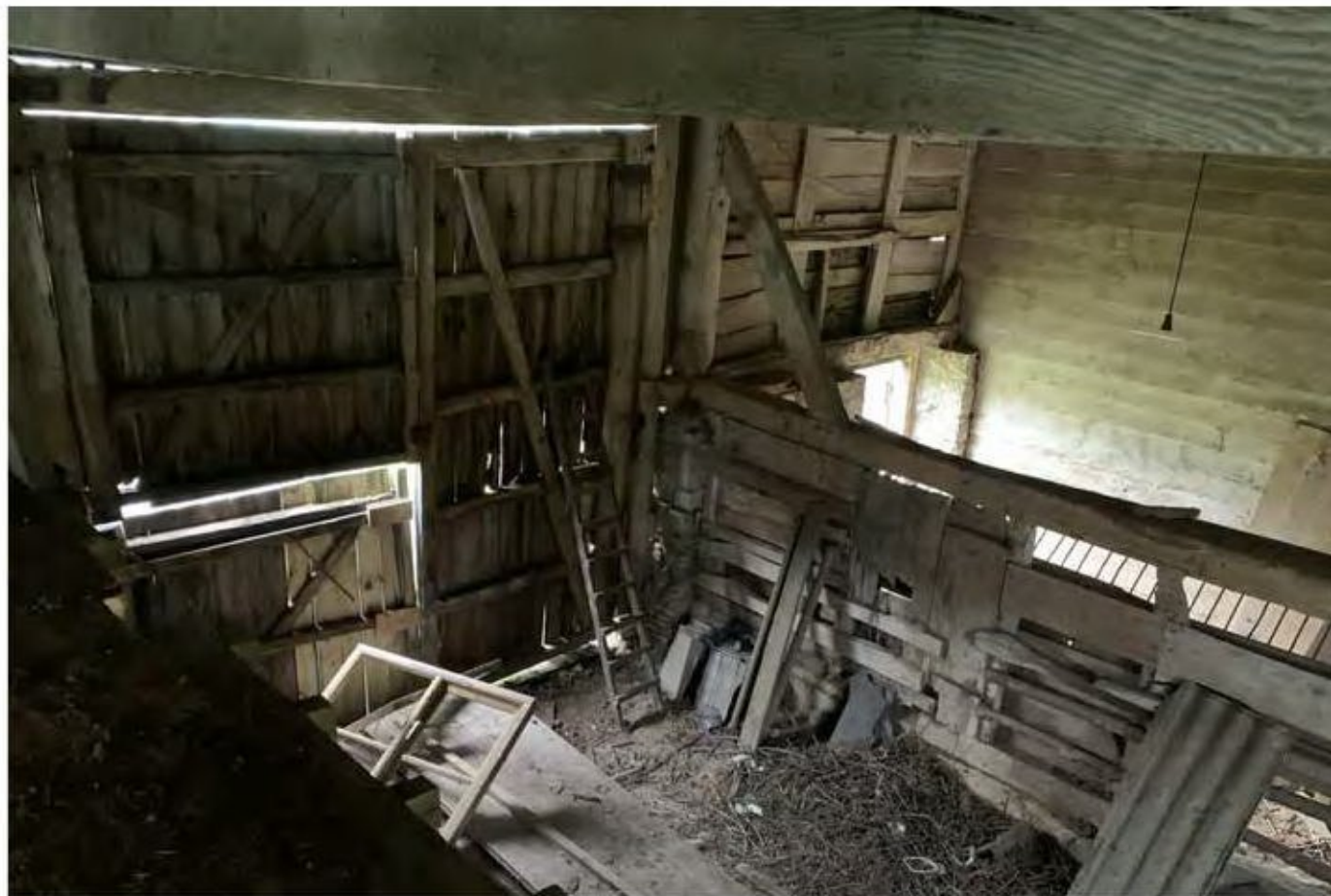
Photo 4. BARN 'A' - CENTRAL PASSAGE (GF) THRESHING BARN CONSERVING DOUBLE HEIGHT SPACE
