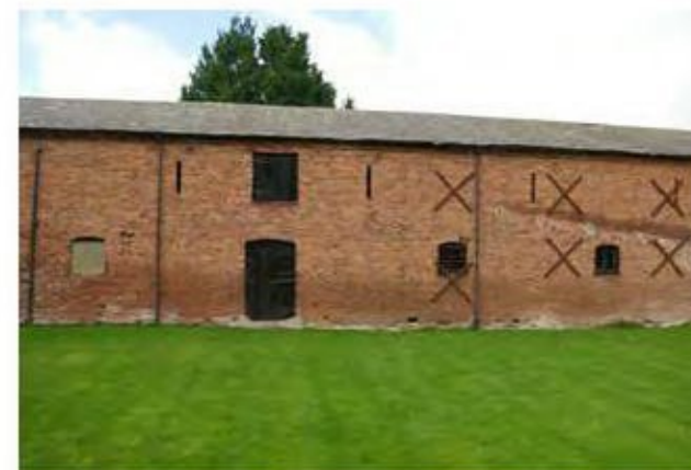
Photo 5. WEST: BARN 'C'
