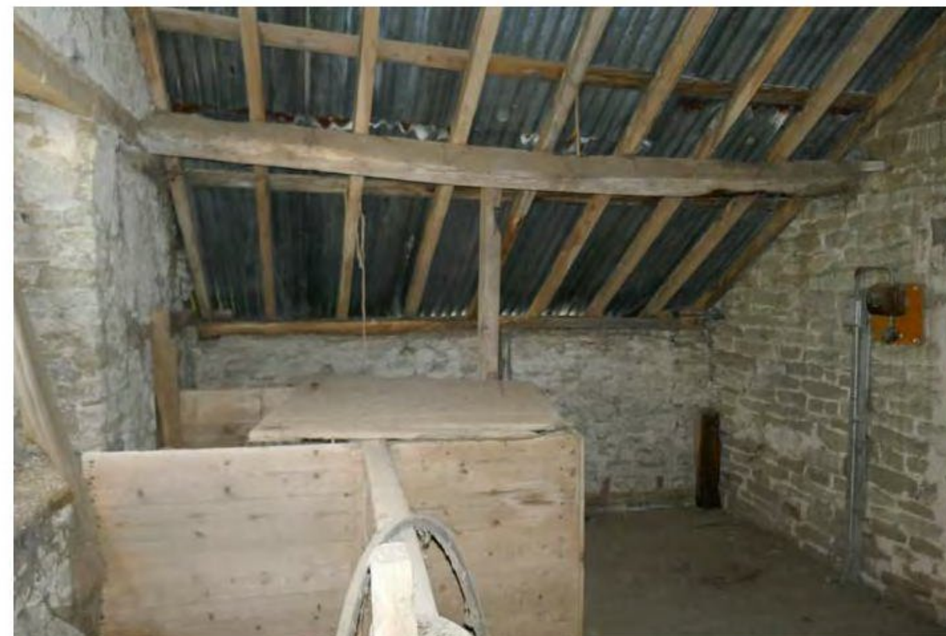
Photo 11. BARN 'D' - 1F LOFT BARN WITH ACCESS TO LOFT
