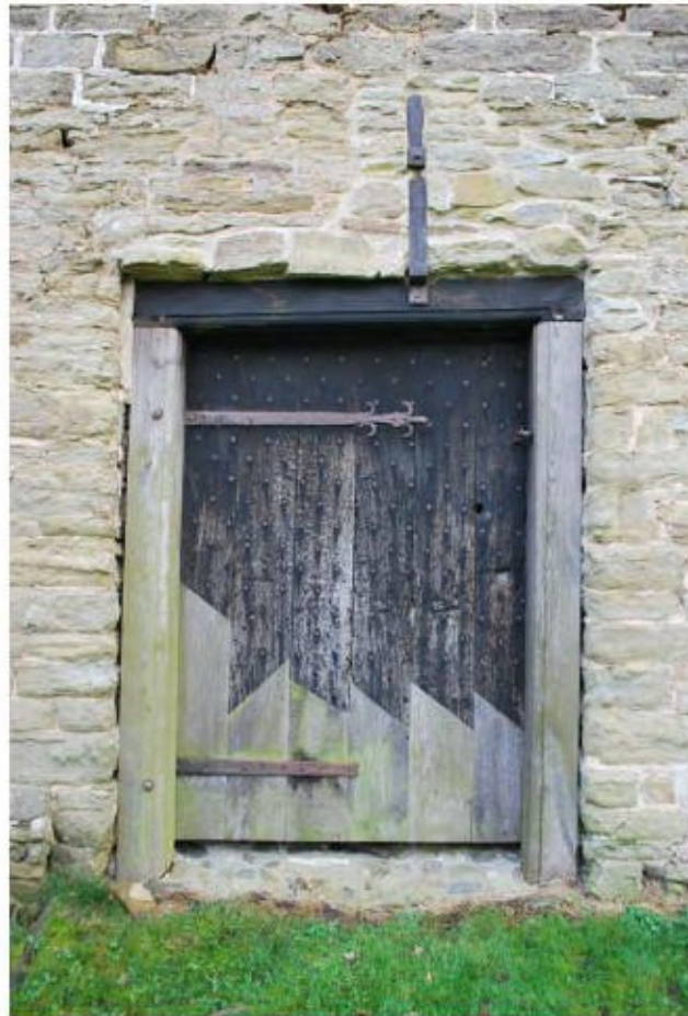
Photo 2. BARN 'A' - NORTH ELEVATION SPAB REPAIRS
