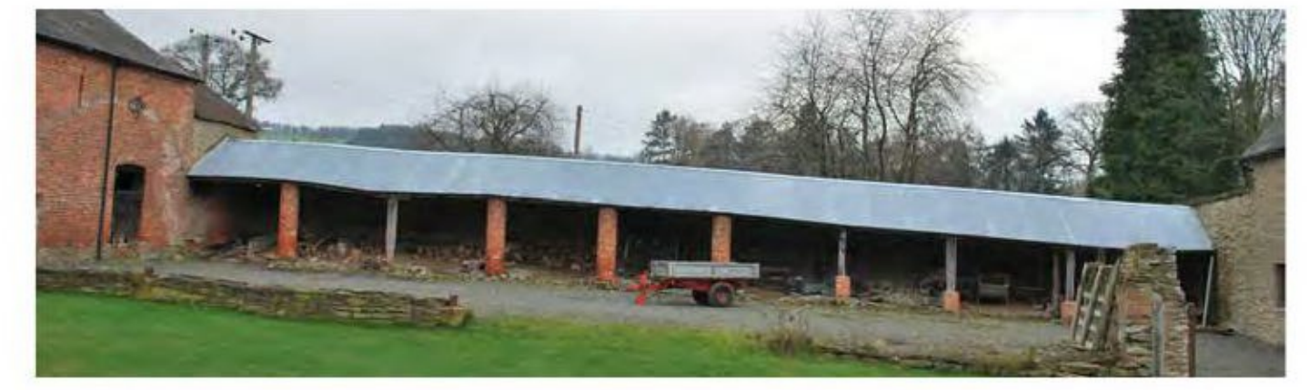
Photo 6. MAIN ELEVATION ALONG COURTYARD
