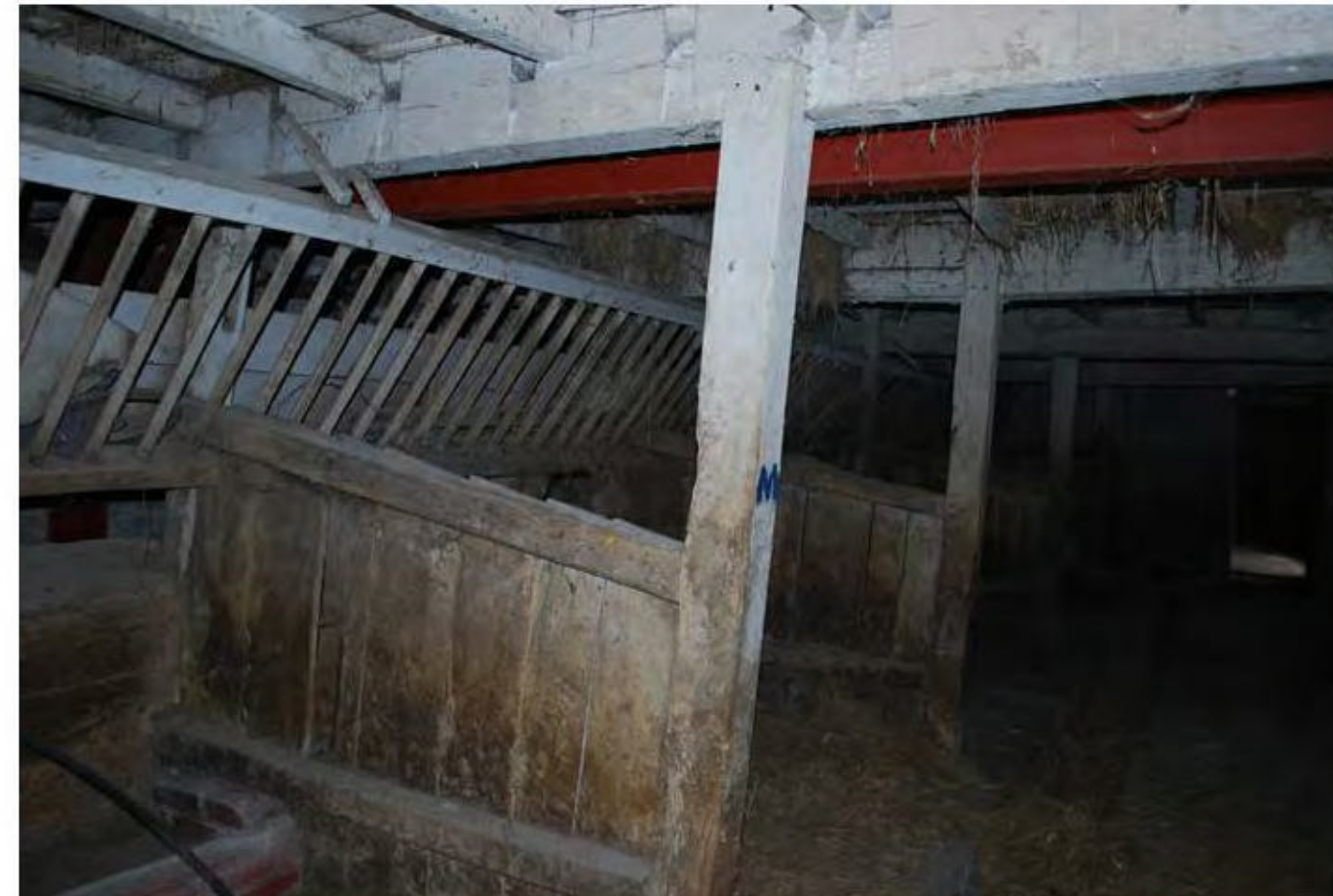
Photo 8. BARN 'C' - GROUND FLOOR STALLS & STRUCTURAL EMERGENCY REPAIRS
