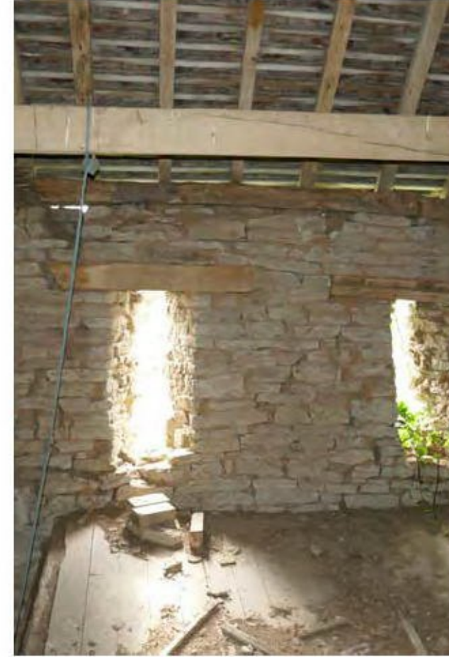
Photo 3. BARN 'A' - SOUTH ELEVATION SLITS
