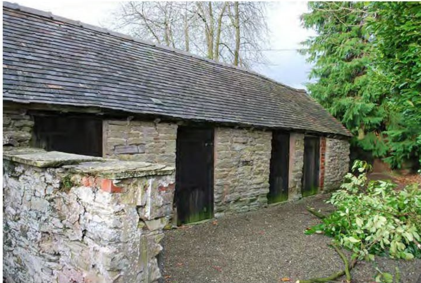
Photo 1. EAST ELEVATION FACING MAIN HALL & BACK OF HOUSE ACCESS
