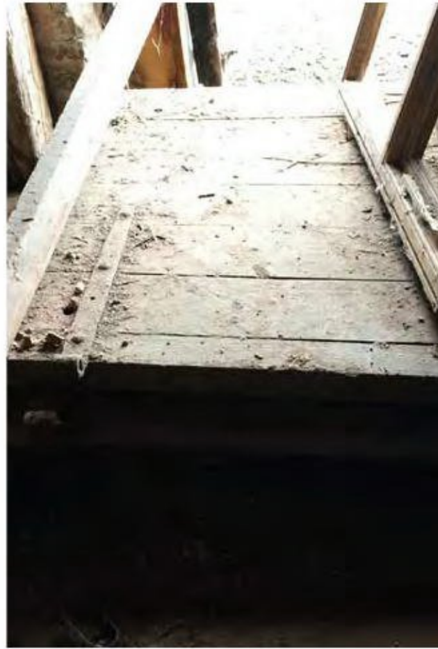
Photo 3. BARN 'A' - GF INTERIORS OLD DOORS PILED ON FLOOR
