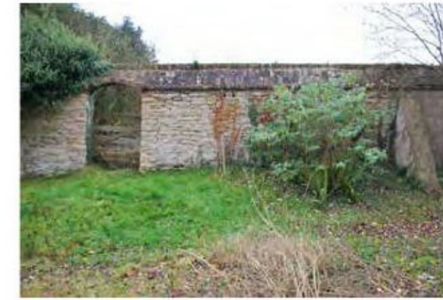
Photo 1B. GARDEN WALL TO THE SOUTH
