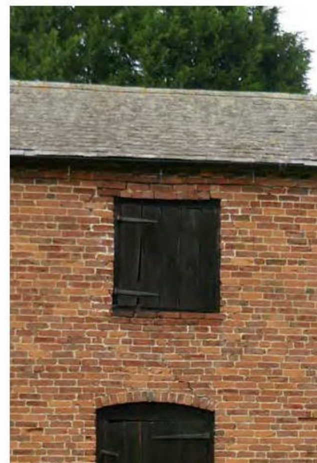
Photo 9. BARN 'C' - EAST ELEVATION LOFT OPENING
