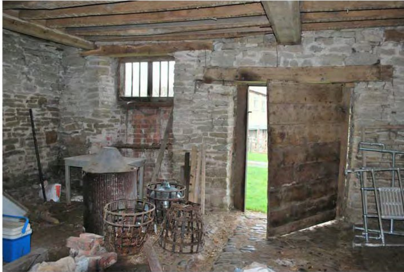
Photo 1. BARN 'A' - SOUTH-EAST CORNER (GF) STONE END BUILDING
