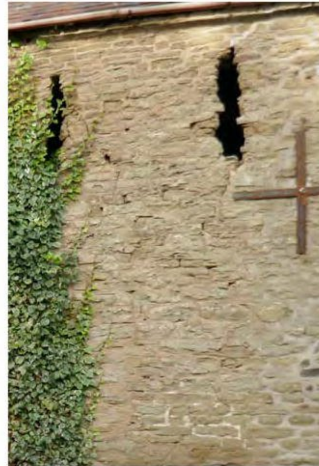
Photo 2. BARN 'A' - SOUTH ELEVATION SLITS
