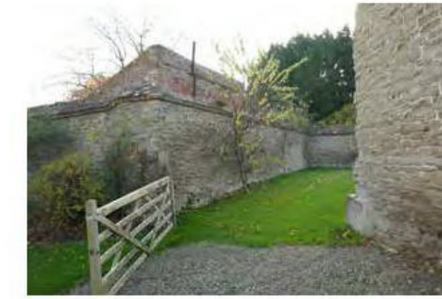
Photo 2. EAST ACCESS BETWEEN BARN 'A' & WALLED GARDEN
