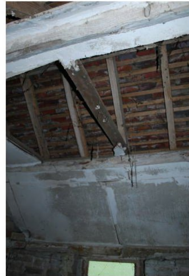
Photo 3A-C. TYPICAL INTERIOR
