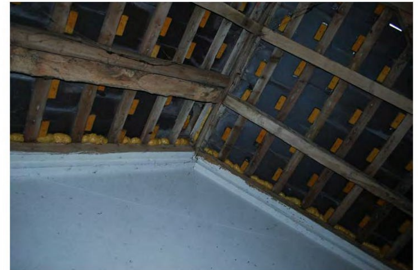
Photo 6. BARN 'B' - NON-ACCESSIBLE ATTIC CONVERTED STORAGE ROOM
