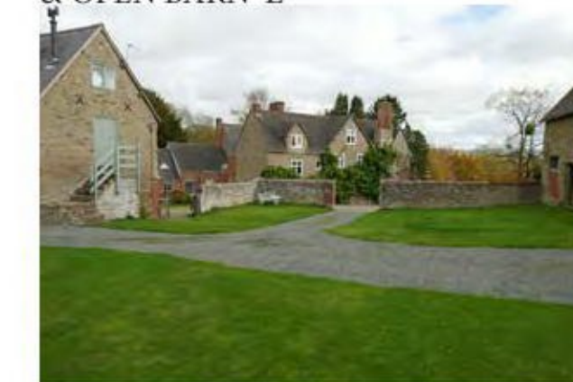
Photo 11. EAST: EAST WALL & ACCESS FACING MAIN HALL
