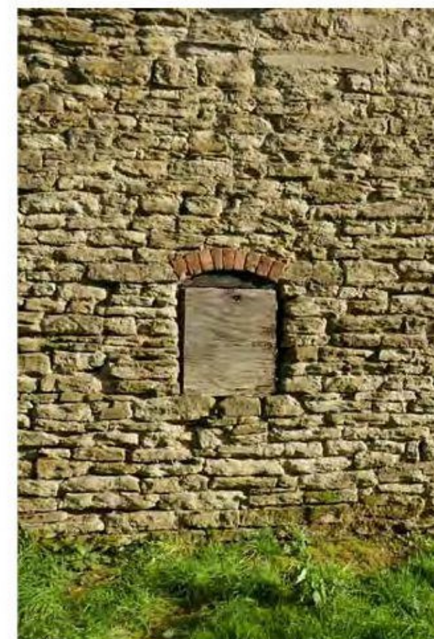
Photo 10. BARN 'C' - WEST ELEVATION GF OPENING
