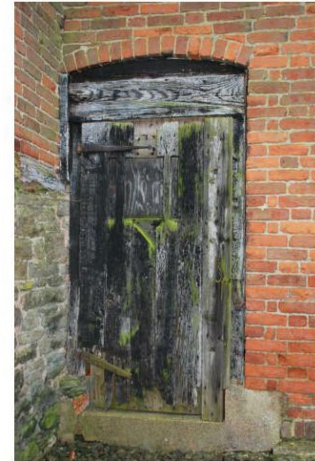
Photo 5. BARN 'A' - SOUTH ELEVATION SURVIVING WOVEN PANELS AT 1ST F.
