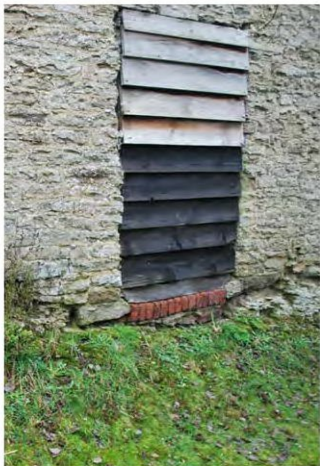
Photo 7. BARN 'B' - SOUTH ELEVATION BLOCKED DOOR
