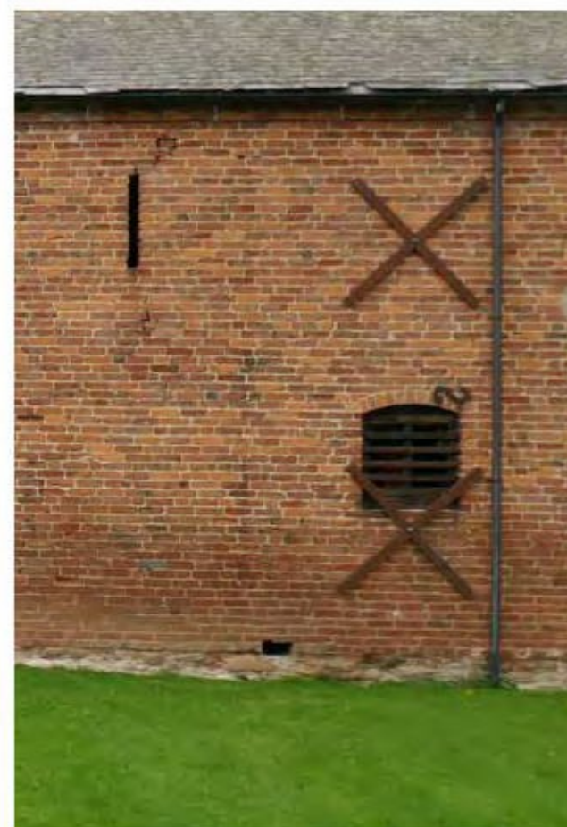
Photo 8. BARN 'C' - EAST ELEVATION SLITS & GF OPENING
