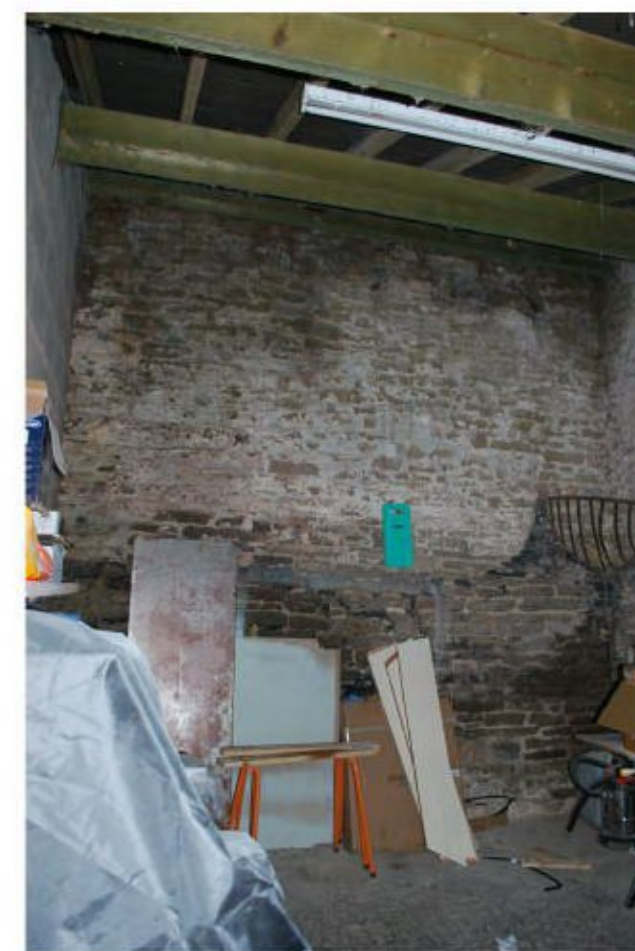
Photo 3C. NORTH UNIT - INTERIOR
