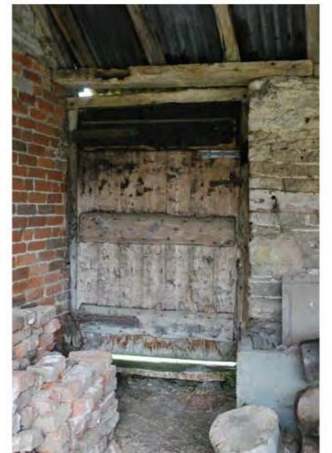
Photo 12. BARN 'C' & 'D' ACCESS TO OTHER PROPERTY
