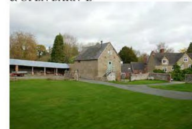
Photo 10. NORTH-EAST: OPEN BARN 'E', COACH HOUSE 'F' AND MAIN HALL ON THE EAST
