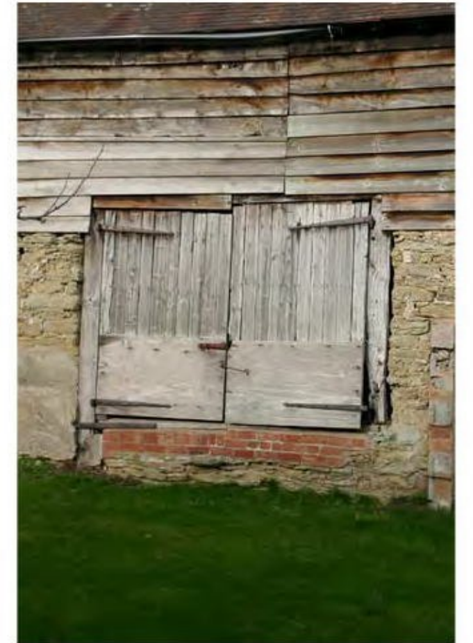
Photo 6. BARN 'D' - NORTH END STONE CONSTRUCTION AT 1ST F.
