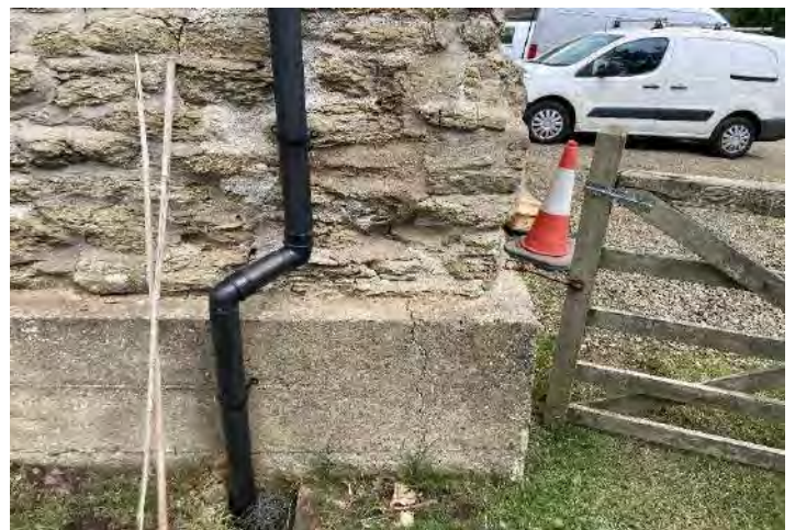
Plate 15 Infilled opening (& concrete underpinning?) of E end of southern limb of barns. Plate 16 Localised cracking within concrete.
