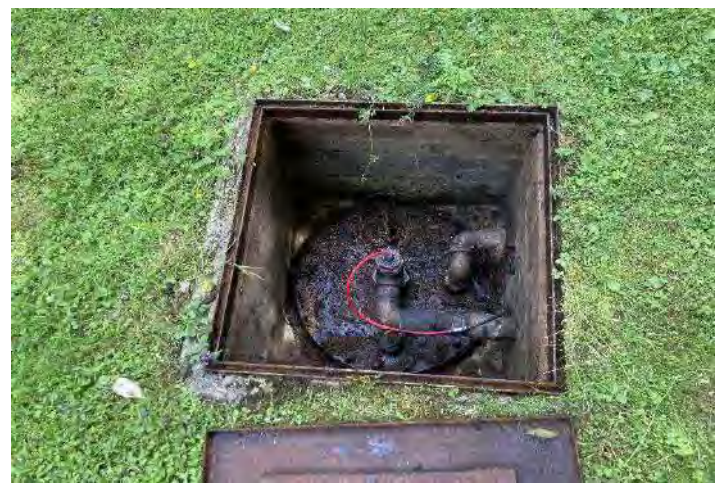
Plate 31 Manhole to redundant oil tank. Apparent breather pipe in background, to right of centre. Plate 32 Oil tank manhole.
