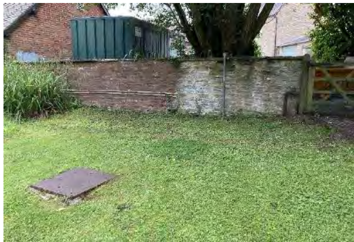
Plate 31 Manhole to redundant oil tank. Apparent breather pipe in background, to right of centre. Plate 32 Oil tank manhole.
