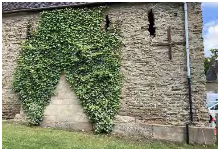
Plate 15 Infilled opening (& concrete underpinning?) of E end of southern limb of barns. Plate 16 Localised cracking within concrete.
