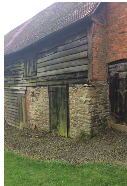
Photo 8. BARN 'A' & 'B' JUNCTION BETWEEN STONE, BRICK & TIMBER CLADDING
