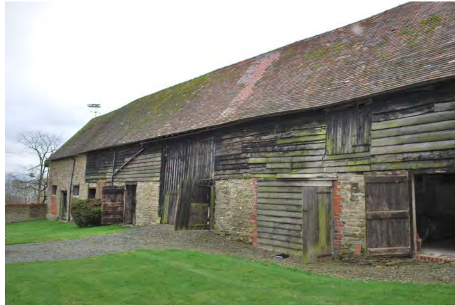
Photo 1. NORTH ELEVATION FACING COURTYARD & TILED ROOF
