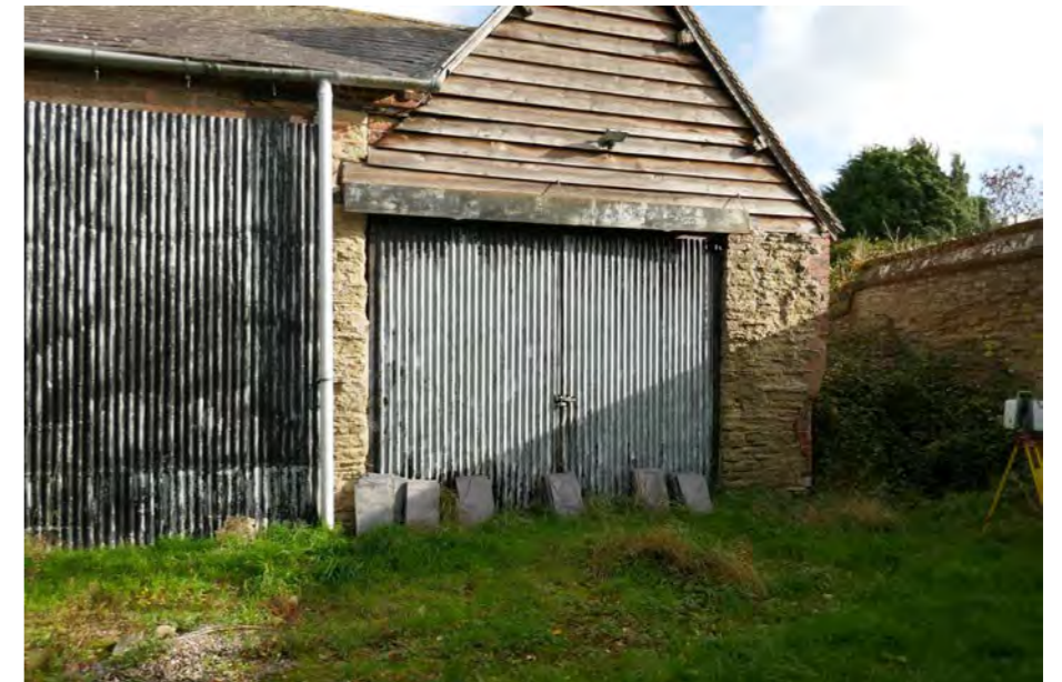
Photo 2. WEST ELEVATION FACING OTHER PROPERTY & CORRUGATED IRON DOORS
