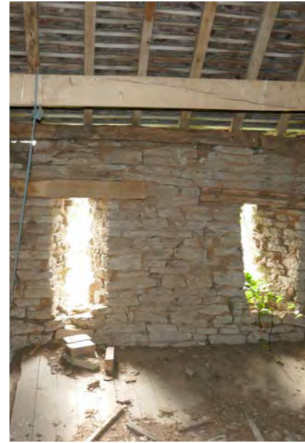
Photo 3. BARN 'A' - EAST END STONE CONSTRUCTION AT 1ST F.
