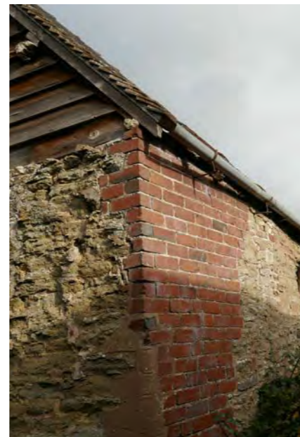
Photo 9. BARN 'B' - SOUTH-WEST CORNER & BRICK INFILLING
