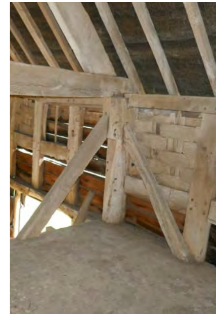
Photo 5. BARN 'A' - SOUTH ELEVATION SURVIVING WOVEN PANELS AT 1ST F.
