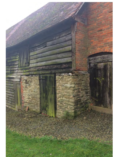
Photo 9. JUNCTION BETWEEN BARN 'A' & 'B' - SOUTH SIDE
