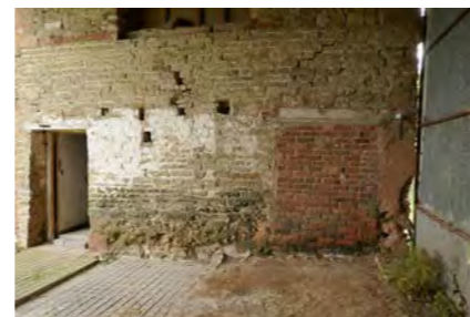
Photo 8. SOUTH GABLE WALL
