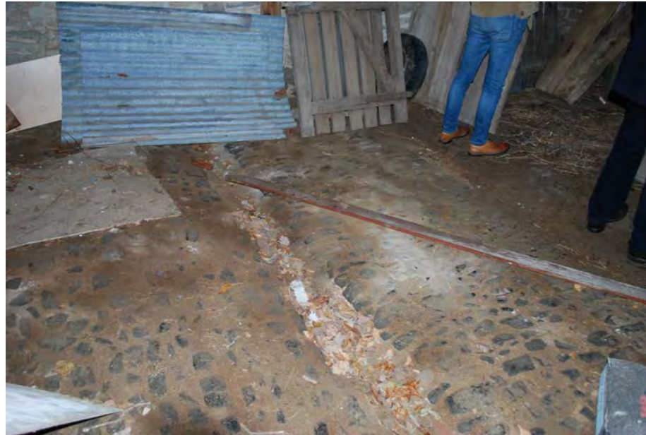
Photo 1. BARN 'A' - COBBLE FLOOR WITH DRAINAGE CHANNEL
