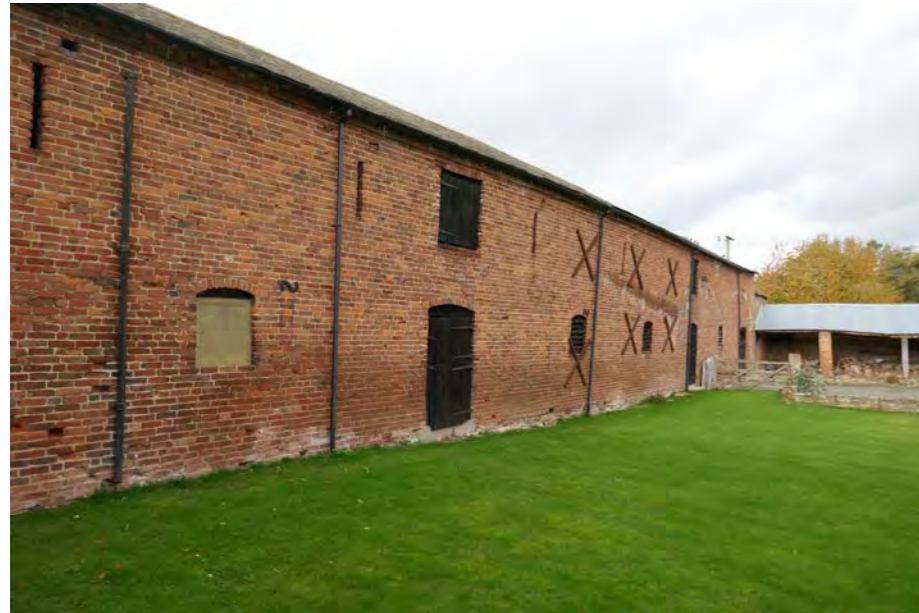
Photo 1. EAST ELEVATION FACING COURTYARD & SLATED ROOF
