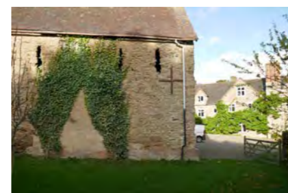
Photo 9. SOUTH-EAST END - SLIT OPENINGS & BLOCKWORK REPAIRS
