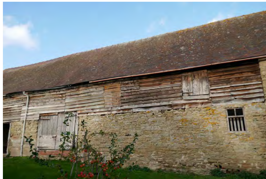
Photo 2. SOUTH ELEVATION FACING WALLED GARDEN & TILED ROOF
