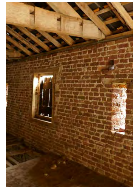
Photo 12. BARN 'C' - EAST ELEV. BRICK CONSTRUCTION AT 1ST F.
