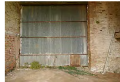
Photo 9. CORRUGATED IRON DOOR FACING OTHER PROPERTY
