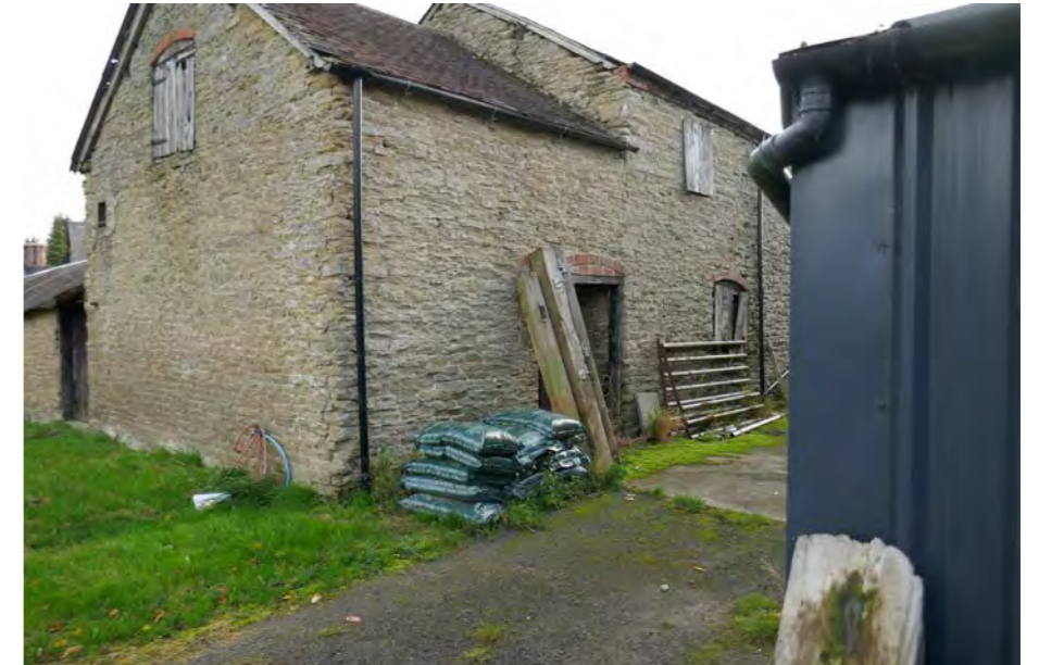
Photo 2. WEST ELEVATION FACING OTHER PROPERTY & TILED ROOF
