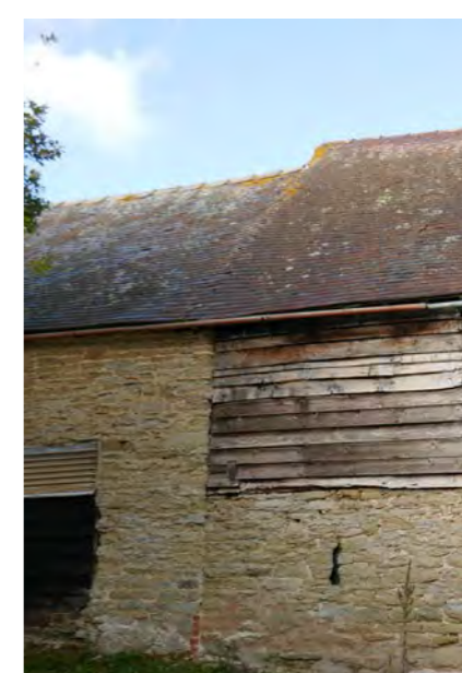
Photo 10. JUNCTION BETWEEN BARN 'A' & 'B' - NORTH SIDE
