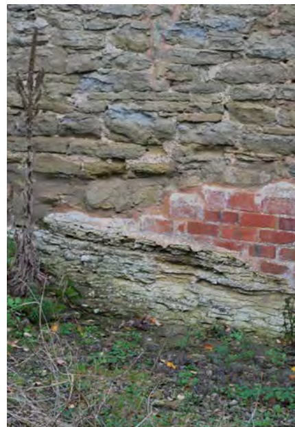
Photo 7. BARN 'A' - SOUTH ELEVATION WALL BUILT ON NATURAL ROCK
