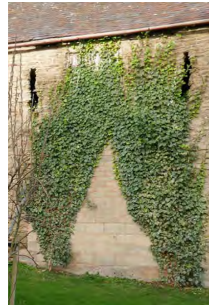
Photo 4. BARN 'A' - SOUTH ELEVATION BLOCKWORK INFILLING
