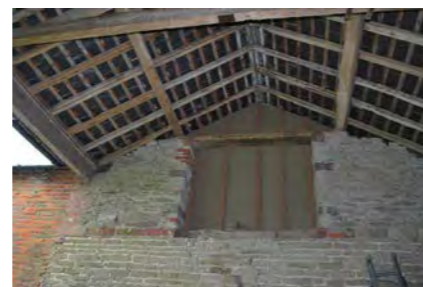
Photo 3. WALL BETWEEN BARN 'B' & 'C'
