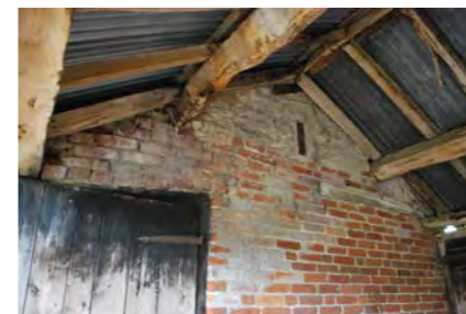
Photo 6. EAST ELEVATION - COLONNADE GABLE END
