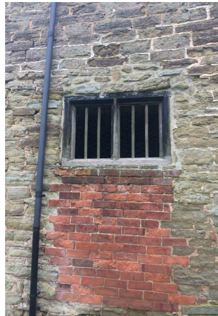
Photo 1. BARN 'A' - NORTH ELEVATION STONE WALL & BRICK INFILLING
