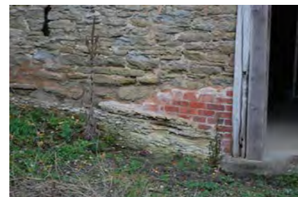
Photo 8. SOUTH ELEVATION BUILT ON NATURAL ROCK
