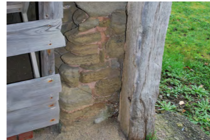
Photo 6. DELAMINATED STONE
