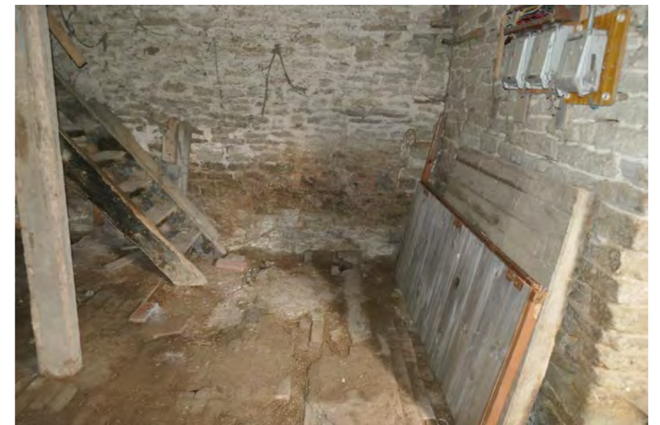
Photo 6. BARN 'D' - BRICK FLOOR
