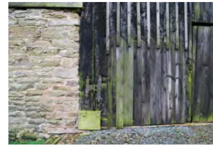
Photo 4. THRESHING BARN DOOR
