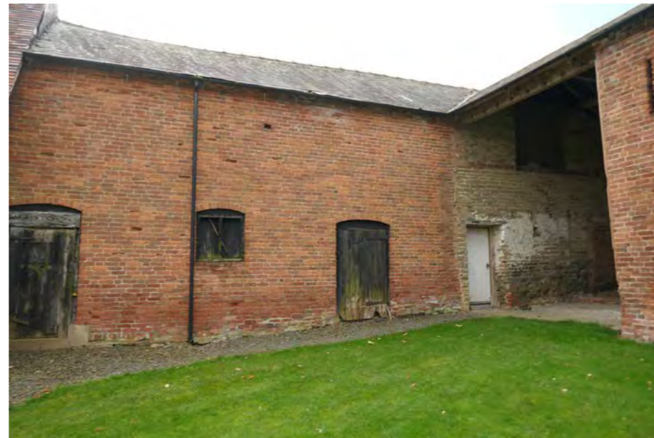
Photo 1. NORTH ELEVATION FACING COURTYARD & SLATED ROOF
