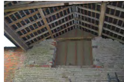
Photo 6. SOUTH GABLE WALL
