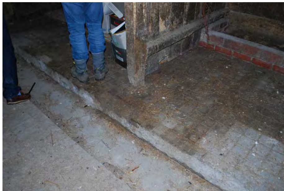
Photo 4. BARN 'C' - CONCRETE FLOOR WITH DRAINAGE CHANNEL & STALLS
