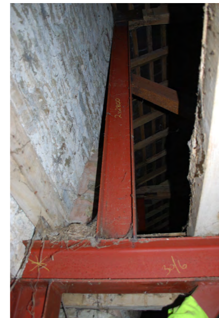
Photo 11. BARN 'C' - WEST ELEVATION STONE WALL & BUTTRESS
