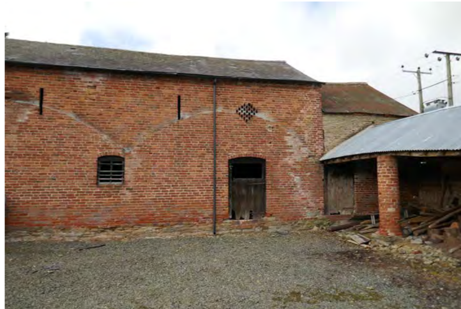
Photo 1. EAST ELEVATION FACING COURTYARD & CORRUGATED IRON ROOF
