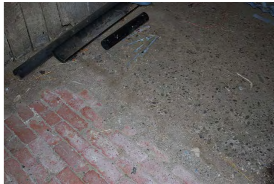
Photo 5. BARN 'C' - CONCRETE FLOOR & TRACES OF BRICK FINISH
