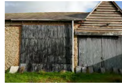
Photo 4. CORRUGATED IRON DOORS
