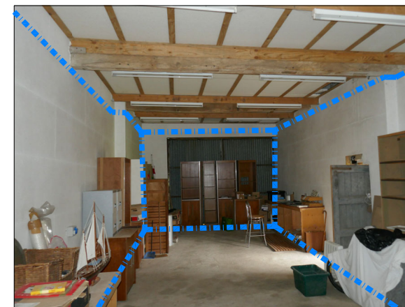
10 11 Remove modern internal lining to rediscover existing openings to North & South elevations.
