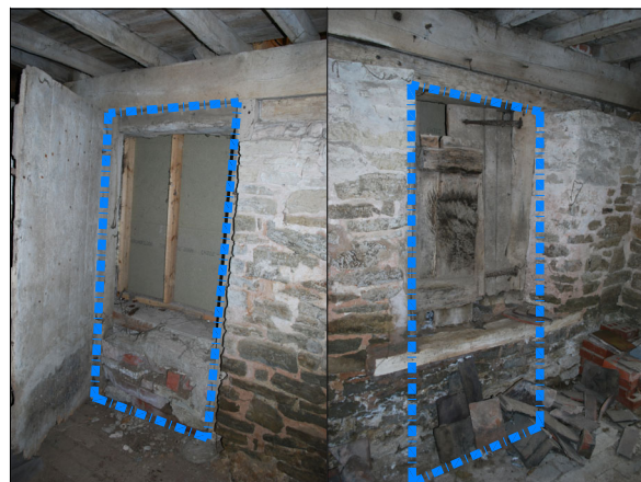
09 Alter/rediscover existing openings to improve GF circulation.
