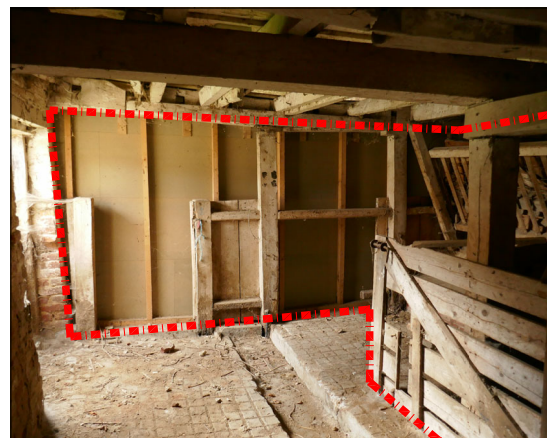
13 Remove stalls & modern dry lining to open up plan and allow more flexible use of GF.
