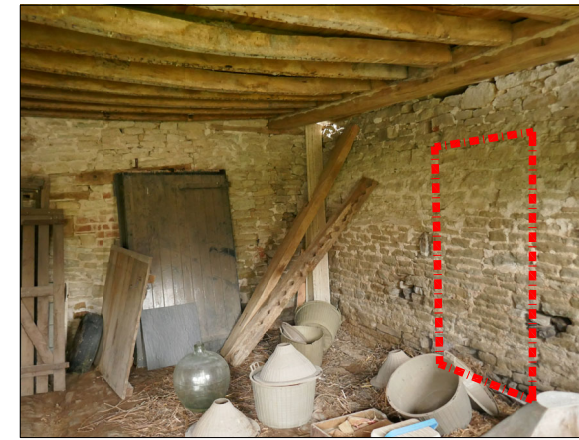
04 Create new opening for circulation at GF between proposed gym & recreational area.
