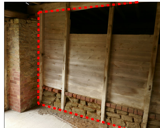
07 Remove modern stud partition & brick/stone plinth.
