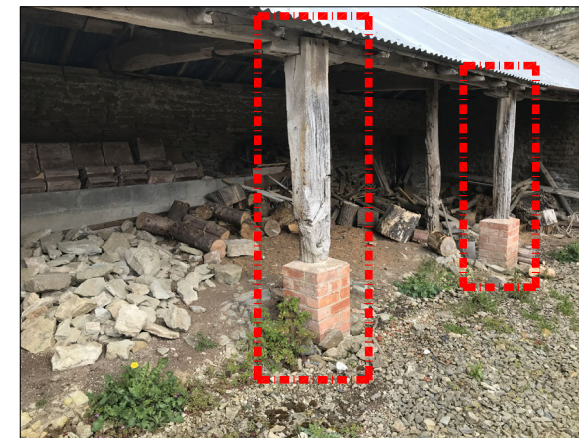
15 Remove timber propping to reinstate brick columns.
