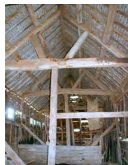
Examples of other barns with traditional ventilation woven panels.
