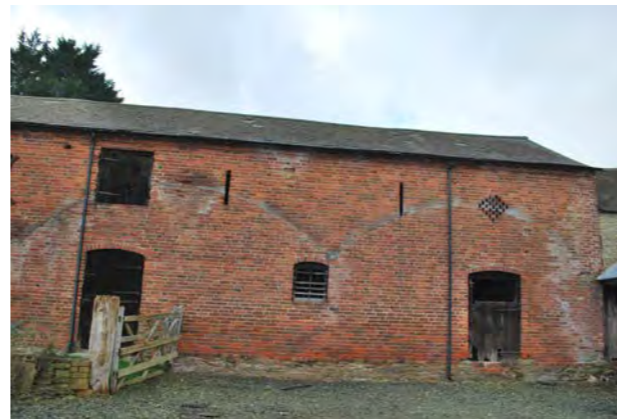
'Dutch' barn traces on West elevation - GQA 2020.
