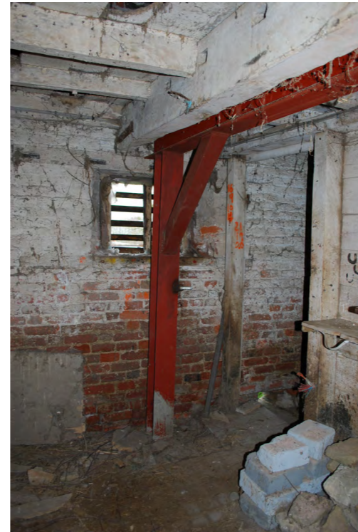
5. INTERNAL STEEL FRAME (EAST WALL)
