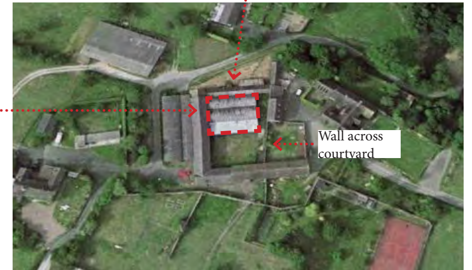
https://www.google.co.uk/intl/en_uk/earth/ - Aerial photograph of the 'Dutch' barns prior to demolition.
