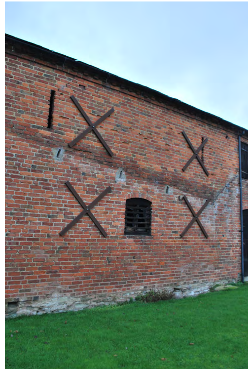
1. STEEL WALL TIES
