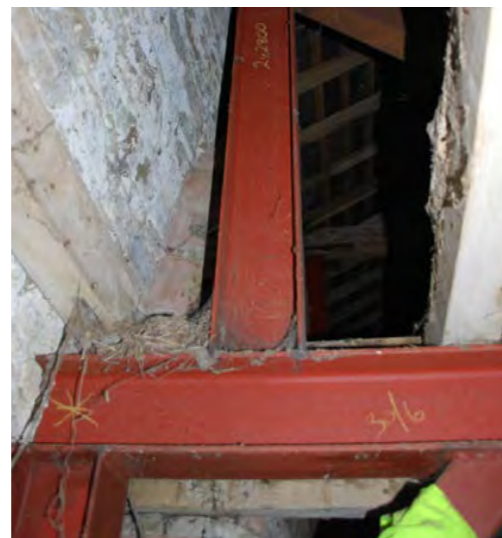
4. INTERNAL STEEL STANCHIONS (WEST WALL)
