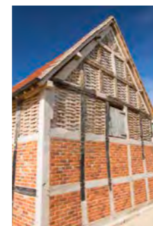
Examples of other barns with traditional ventilation woven panels.
