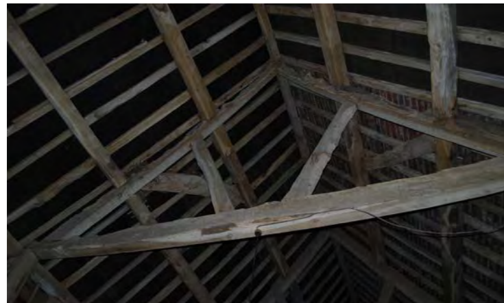
1. SIMPLE TRIANGULAR TRUSS WITH BRACES
