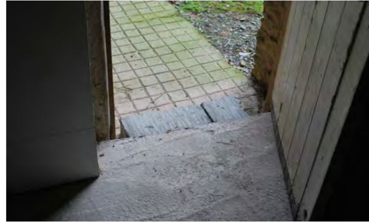
4. MODERN CONCRETE OR CEMENT SCREED
