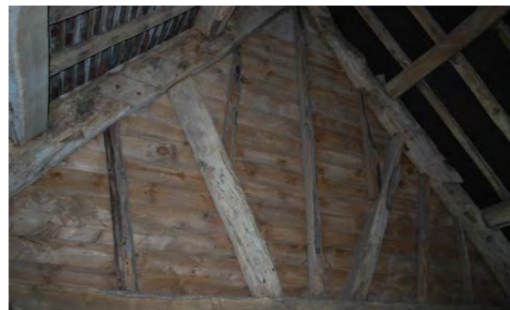
5. SIMPLE TRIANGULAR TRUSS WITH BRACES & MODERN BOARDING
