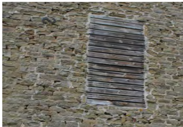
7. TIMBER SLATTED WINDOW OPENING
