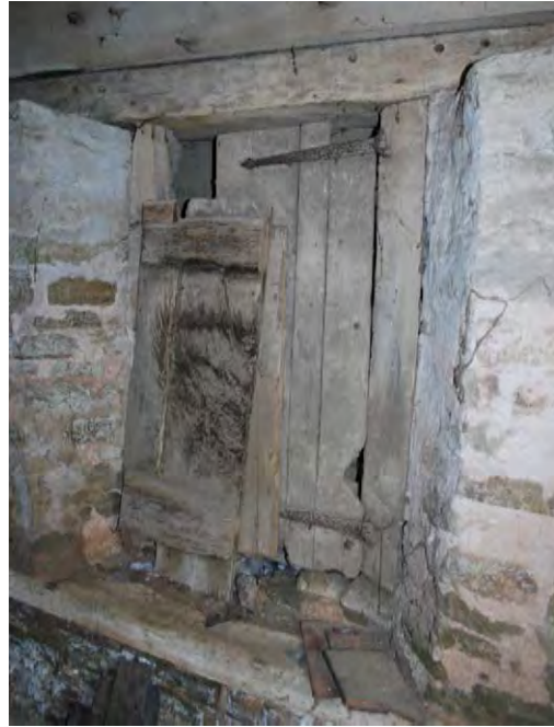
1. FRAGMENTARY REMAINS OF HISTORIC DOORS
