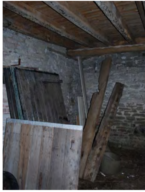
3. REDUNDANT HISTORIC DOORS
