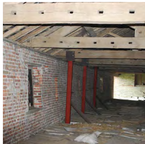
2. INTERNAL STEEL STANCHIONS (EAST WALL)
