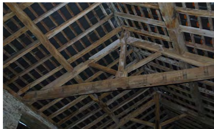
2. KING POST TRUSS MADE FROM RECYCLED TIMBERS
