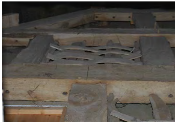
6. A SURVIVING EXAMPLE OF WOVEN STUD WORK
