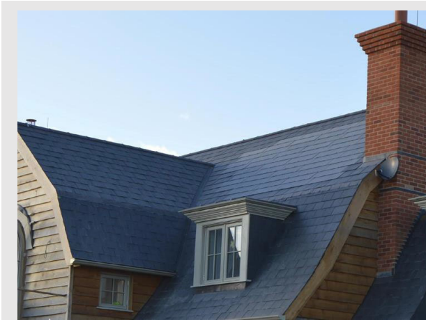
This example shows a PV slates. GB Sol slates current dominate the UK market. They are very discrete, used on listed buildings, and can be continuous in order not to see a border between regular slates. The efficient of the slates is lower than stand PV panels, and the costs are significantly higher.
