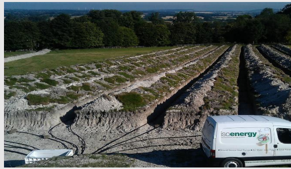
Horizontal ground loop.
