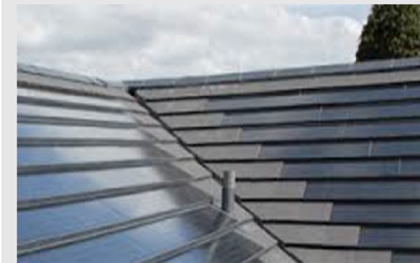
This example shows a typical roof PV tile. Standard panel is mounted on the GSE mounting system. Similar to PV slates, the PV tiles also form part of the roof structure. The costs are comparable with the standard PV.
