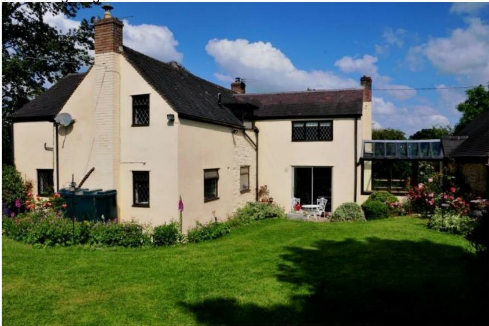
Evenwood Cottage is a much altered 19 th century small holding with a small outbuilding range.
