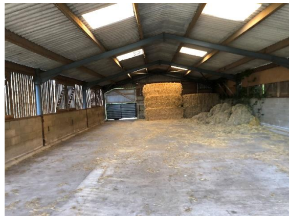
Photo 12: Internal view of B9
