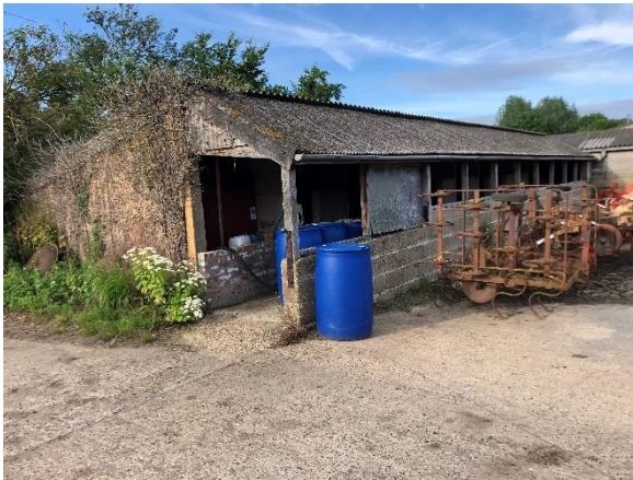
Photo 13: South eastern façade B10
