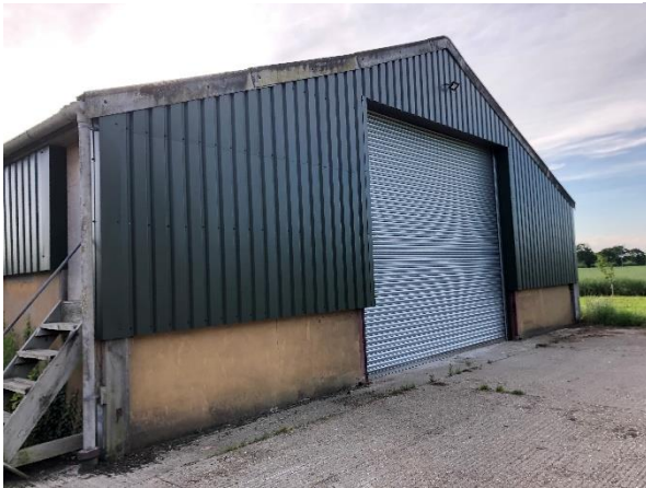
Photo 19: Eastern façade of B13
