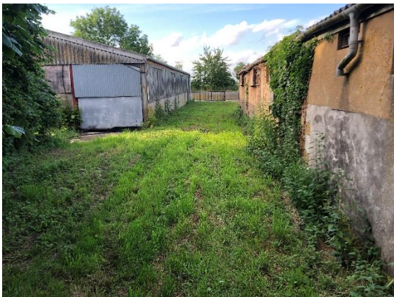
Photo 11: Southern end of B9, with B8 to east and mown grass between the two buildings
