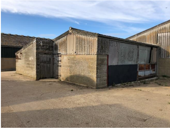
Photo 17: South eastern façade of B12
