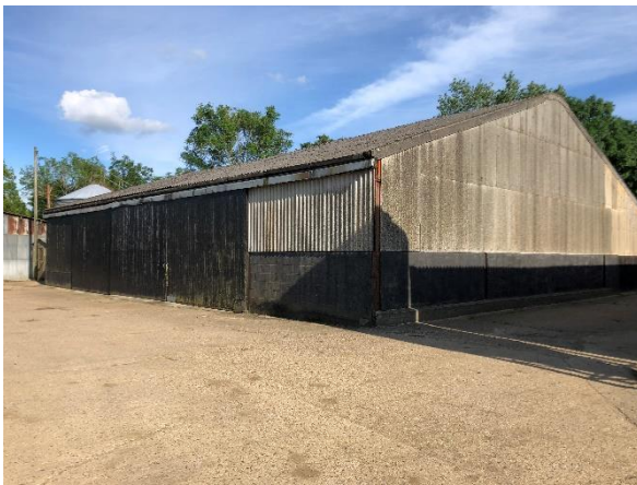
Photo 3: Building 2, northern and western facades
