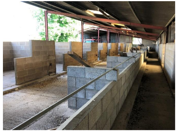
Photo 6: Internal view of B4
