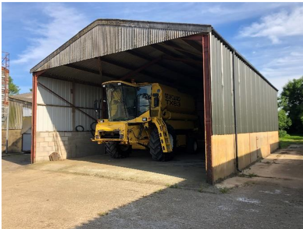
Photo 7: North western façade of B5
