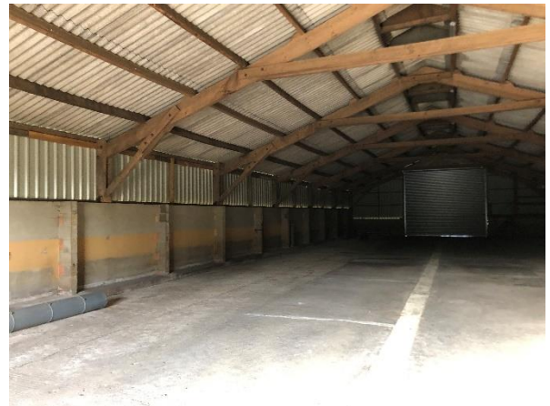
Photo 20: Internal view of B13
