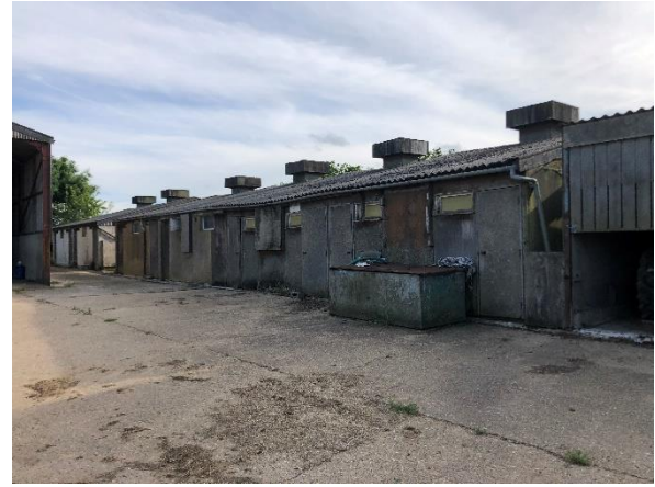
Photo 10: Northern end of B8, viewed from east
