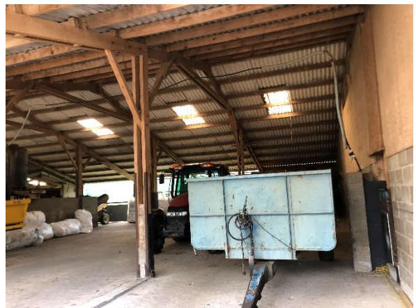
Photo 22: Internal view of B14
