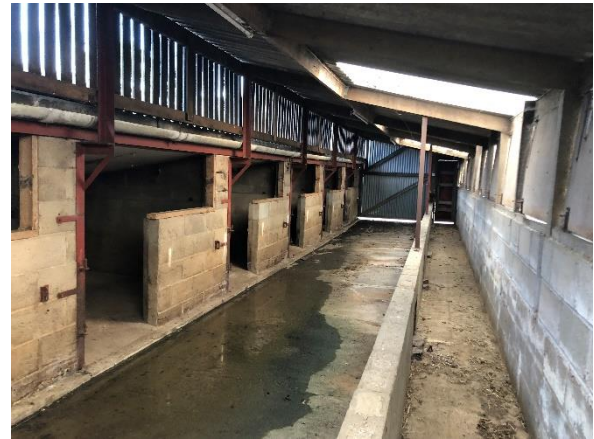
Photo 14: Internal view of B11
