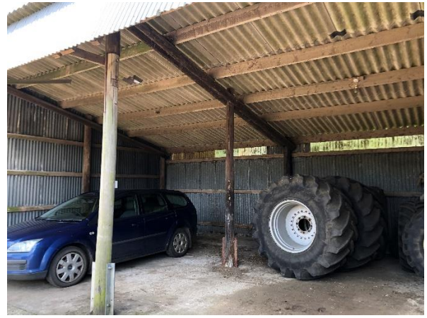
Photo 2: Internal view of B1 open section
