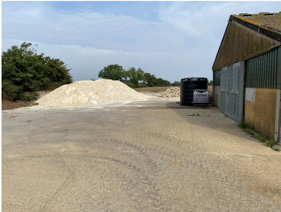
Photograph 15 – Asbestos clad barn, with heap of lime on adjacent hardstanding
