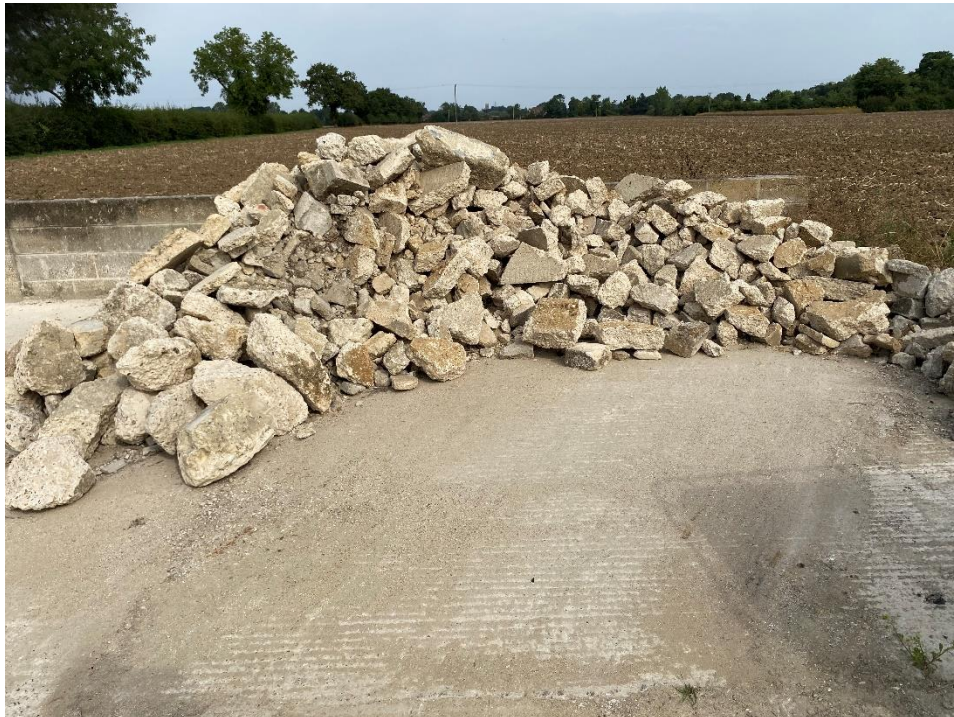
Photograph 16 – Heap of rubble, from demolition of on site building.
