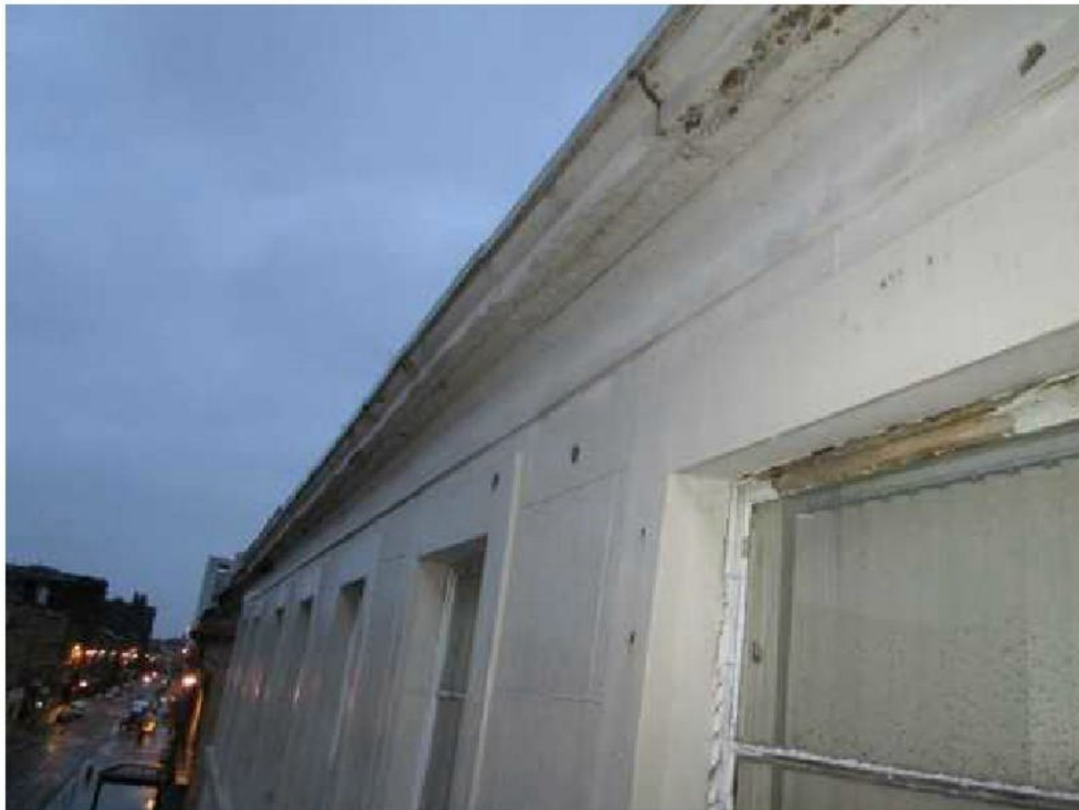
Previous Inspection Holes.
