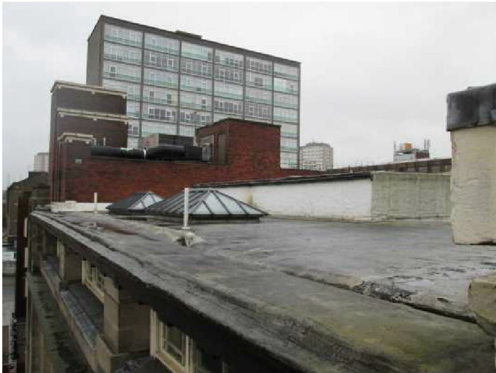
Roof Area (Rose Street)
