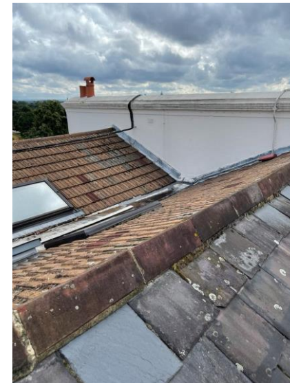
Flat 9 – Roof level showing ridge and parapet.
