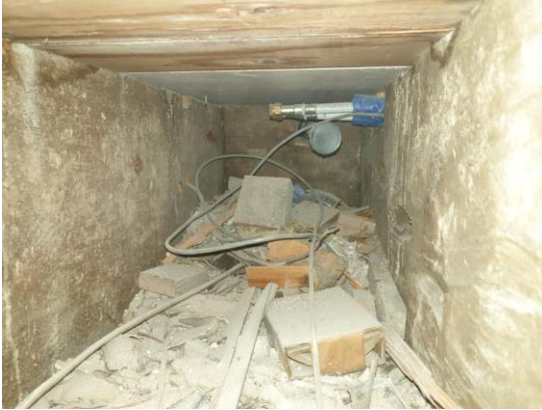
1 st Floor: Cavity under floorboards/ joists
