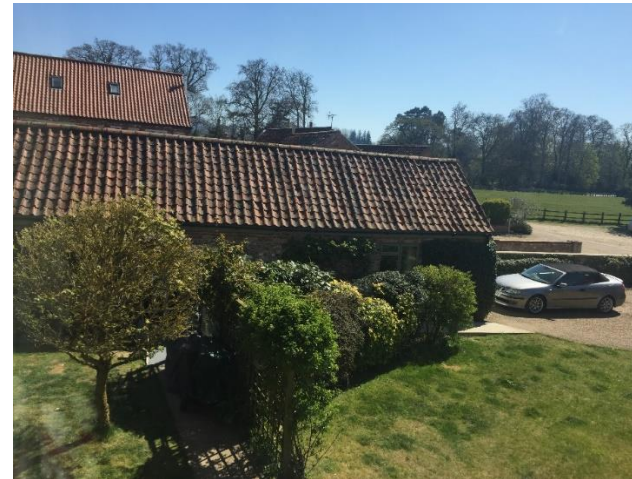
View of annex from man house upstairs window.
