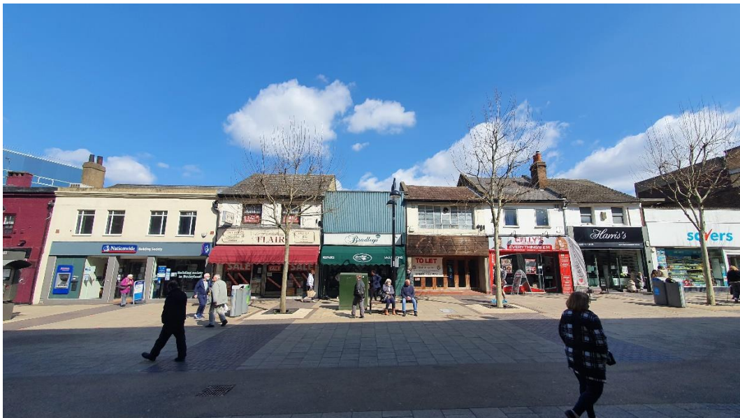
Existing Street View
