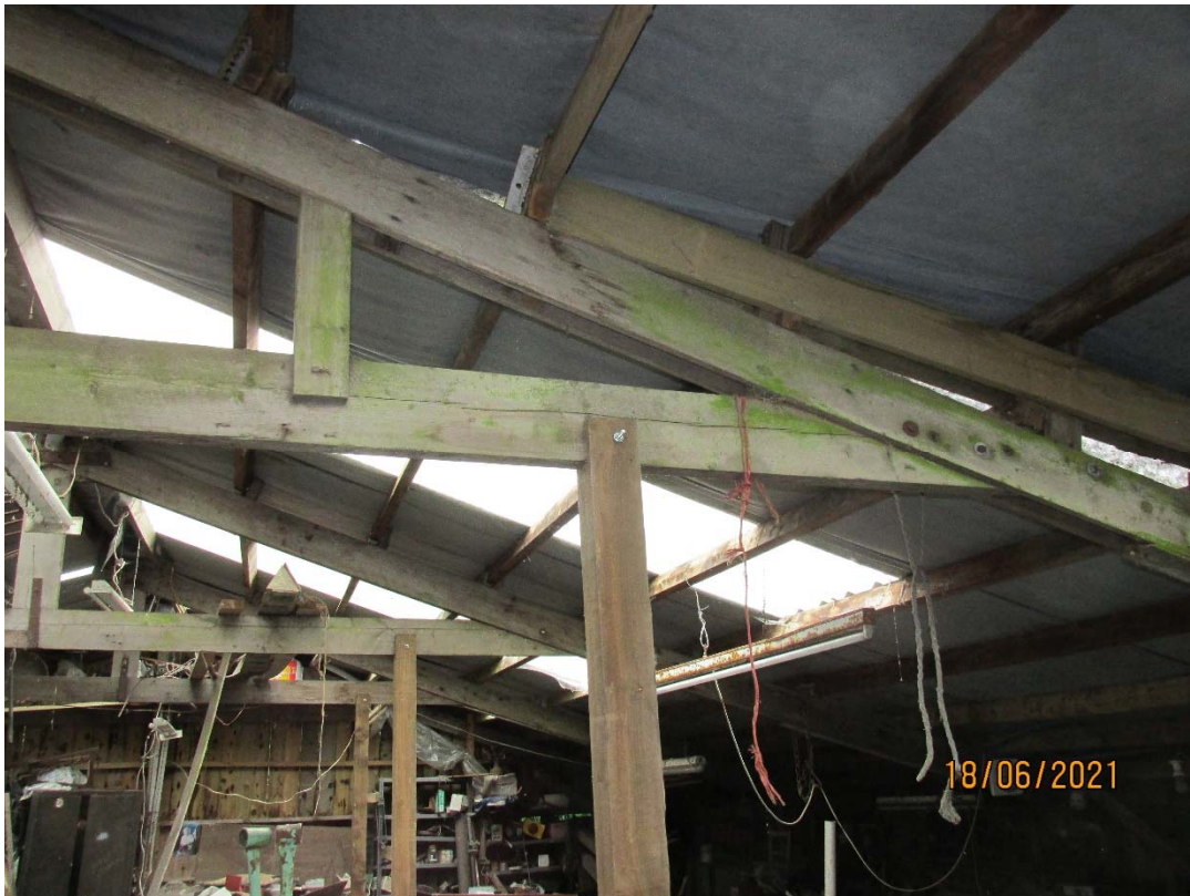
Internal view of Barn showing part of structural timber support frame
