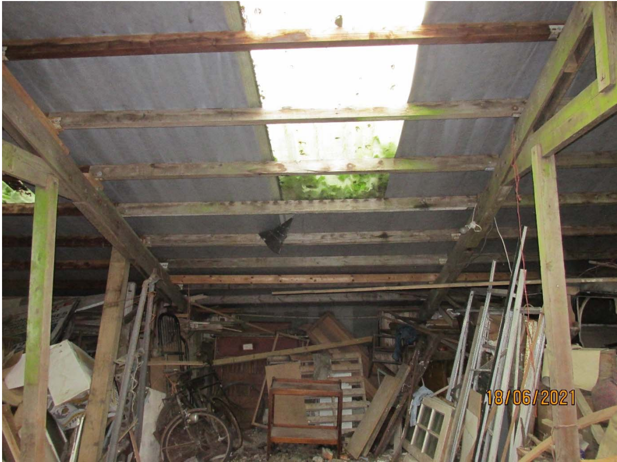
Internal view of Barn showing part of purlins spanning between frames
