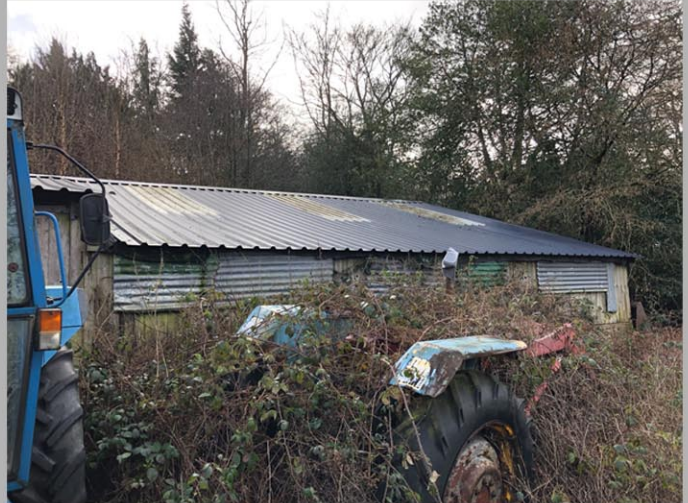
View looking south
