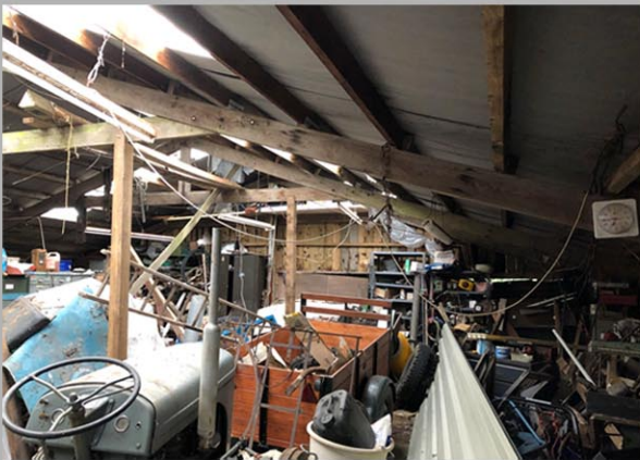
Internal view showing structure
