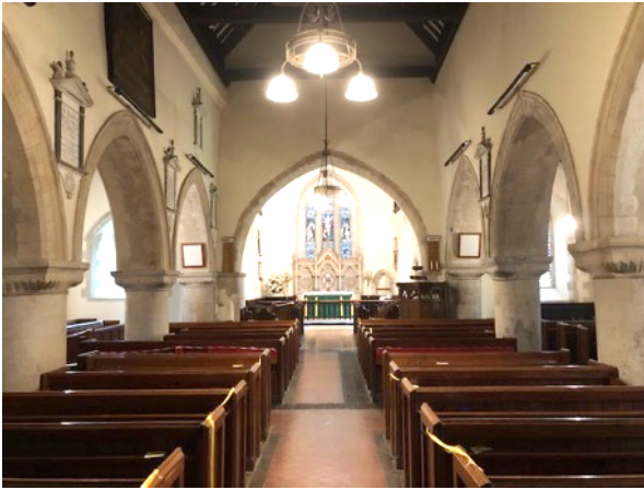
1 Interior looking east. The modest scale of the arcade offsets the loftiness of the roof.
