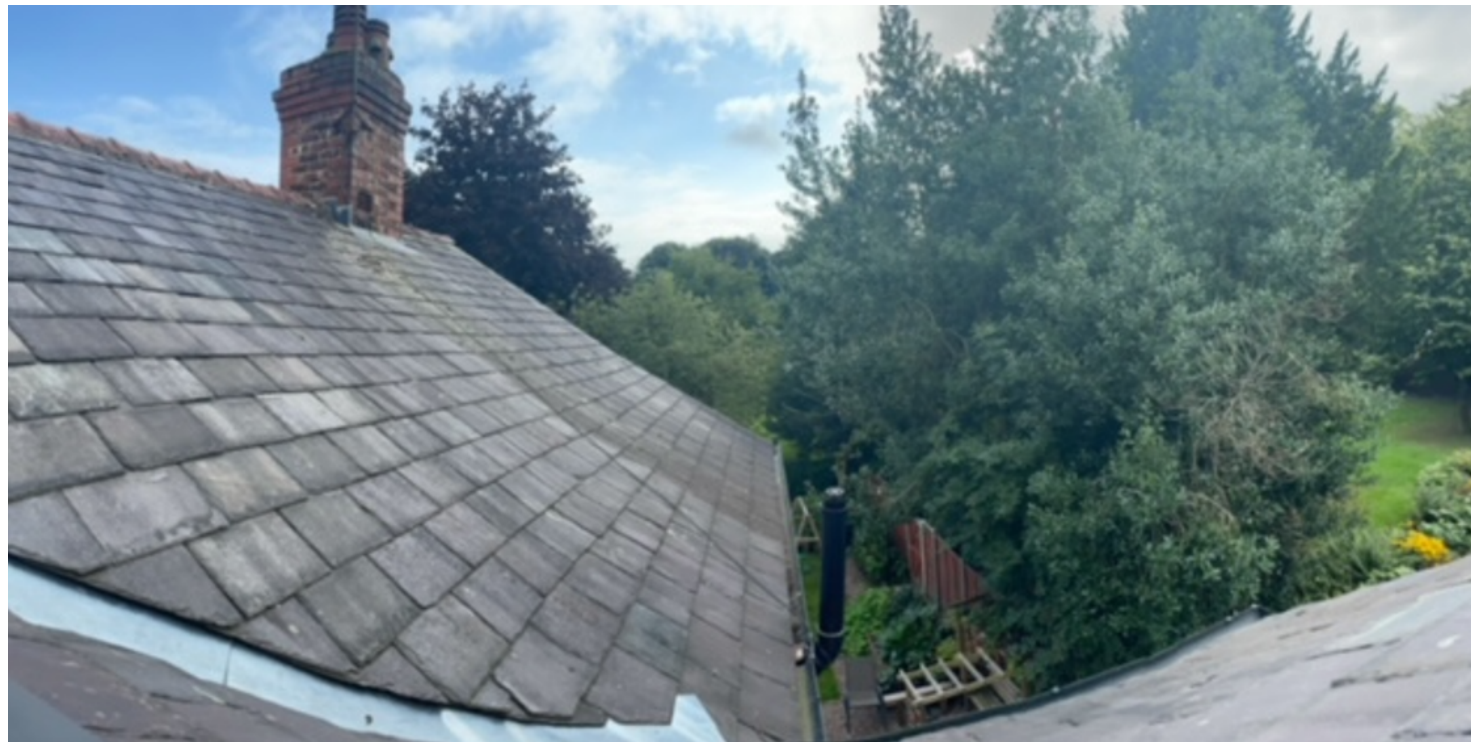
3. Photo looking south (from rooflights)
