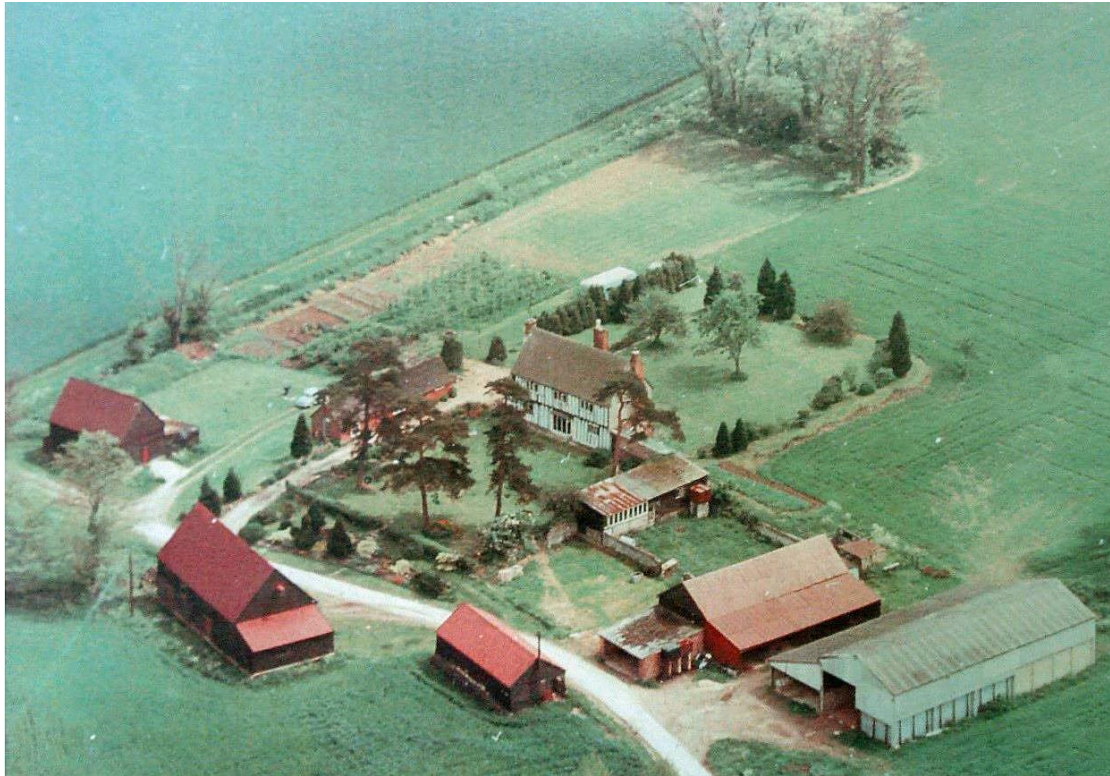
Figure 9. An aerial view of circa 1970 from the north-west showing Barn 3 to the extreme left with a new roof of corrugated iron matching those of the other farm buildings. The adjoining shed to the rear appears to have an almost flat roof several feet below the barn's eaves and the outline of a red central door is just visible in the western gable. The latter corresponds with the reference to a western entrance in the listing description of 1984.
