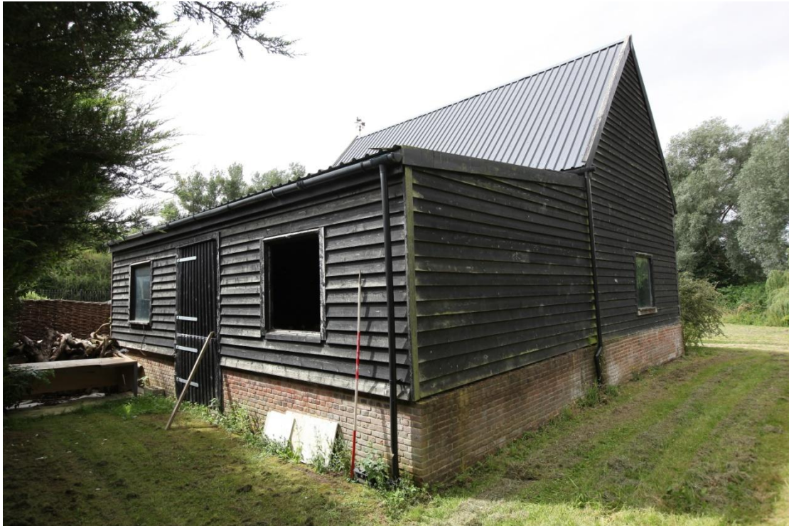
Illus. 7. Barn 3 from the south-east showing its recently built lean-to rear addition designed as loose boxes for horses. The plinth and cladding of the new structure are identical to those of the barn which was extensively renovated and altered at the same time.
