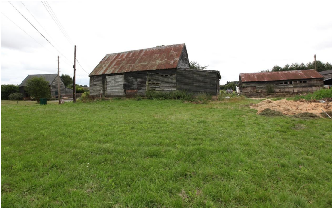
Illus. 2. A general view of the site from the north showing Barn 3 to the left, Barn 1 in the centre and Barn 2 on the right. Barn 2 appears to have been built as a cart lodge in the 18 th century but is listed as 16 th century and consists largely of re-used timber of that period. Barn 1 is a late medieval threshing barn of three bays truncated on the west (just as Barn 3 has been truncated on the east).
