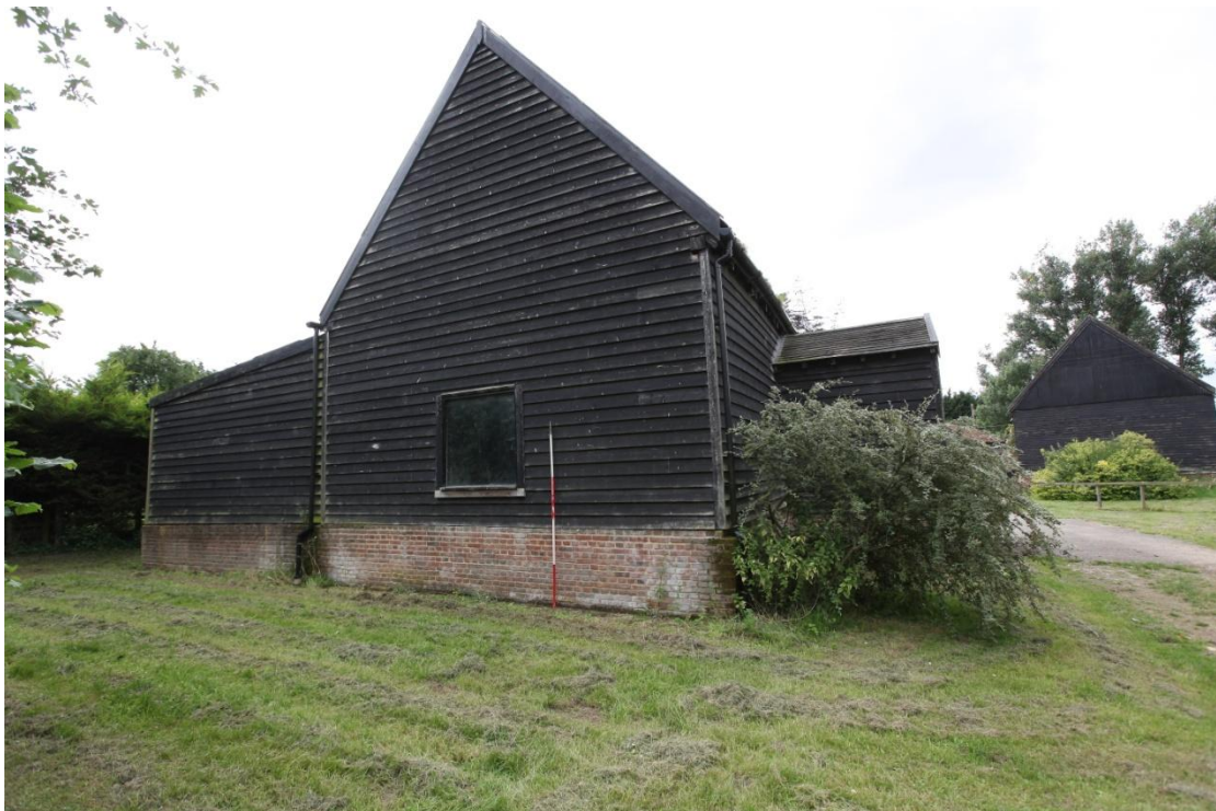
Illus. 6. The external eastern gable with the lean-to rear extension of 2003 on the left. The English Bond brick plinth of the main barn is integral to that of the lean-to, evidently having been replaced when the latter was built, and the weatherboarding of both structures is also identical. The original gable is open-framed and the remaining building either continued into the foreground or adjoined an earlier structure in this position as shown on 19 th century maps.
