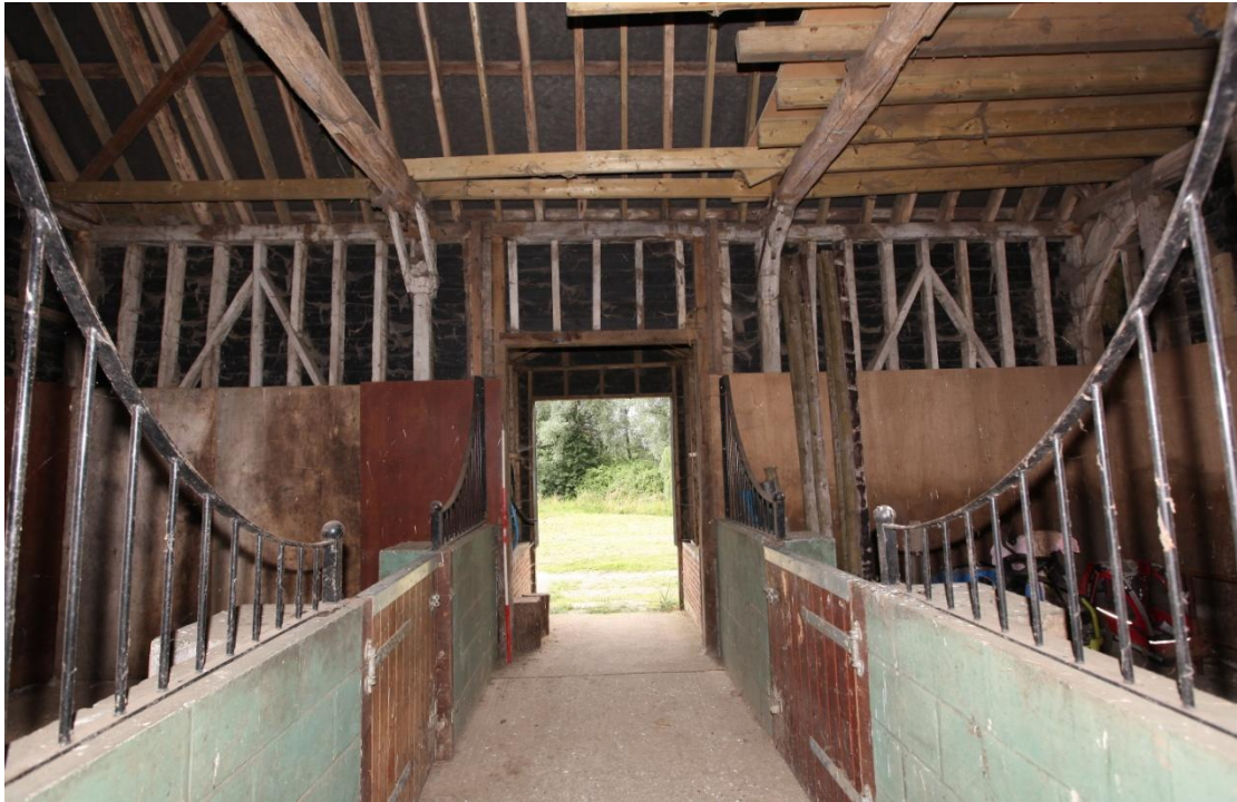
Illus. 9. The northern interior showing its whitewashed original studwork which originally consisted of three bays of identical length with symmetrical framing and no evidence of an entrance. The jambs and lintels of the present porch are insertions of 2003. The short studs above the lintel have been altered, and the central stud bears paint scars and nails for missing diagonal primary braces identical to those of the end bays.
