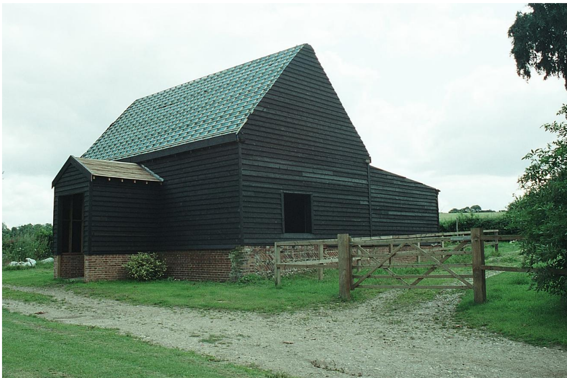
Figure 10. The building in 2004 as its conversion into a stable was nearing completion.
