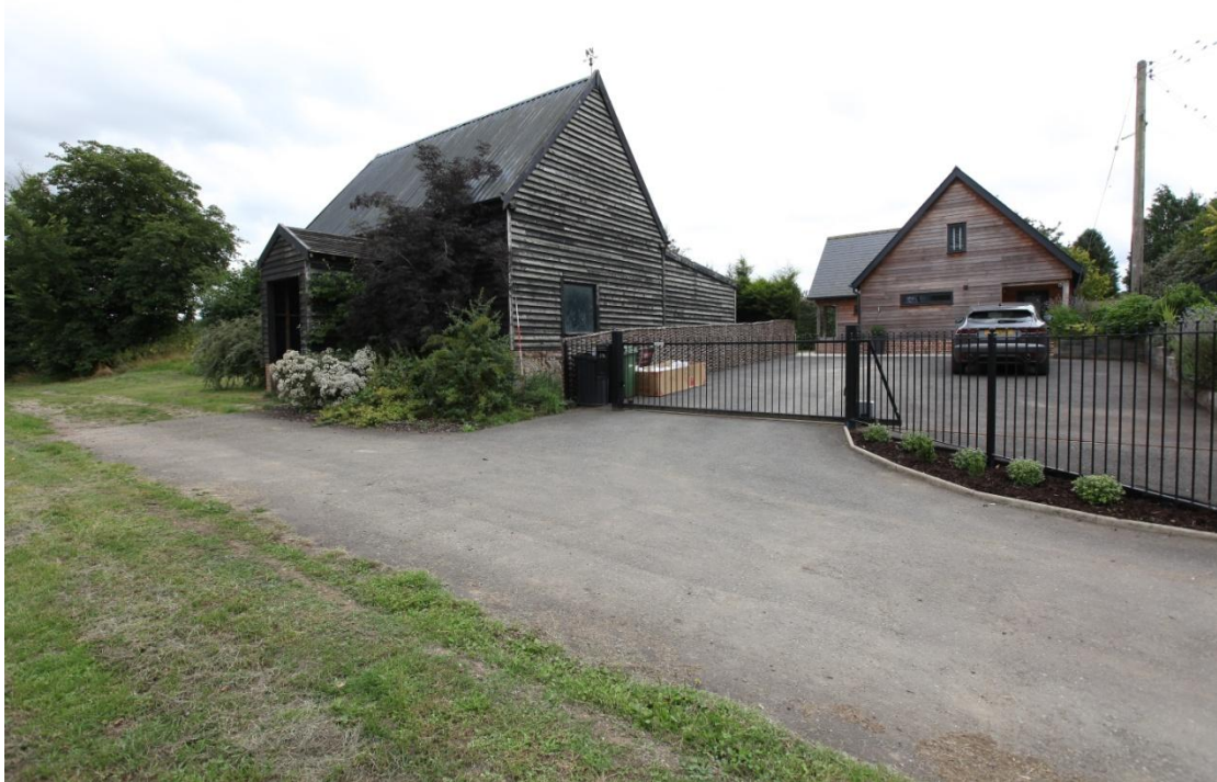
Illus. 3. Barn 3 from the north-west showing its close proximity to the recently built dwelling known as Bower Hall Cottage on the right. The listing description of 1983 refers to an entrance in the western gable but there is no longer any trace of this in the weatherboarding or plinth which have since been renewed (see illus. 13)
