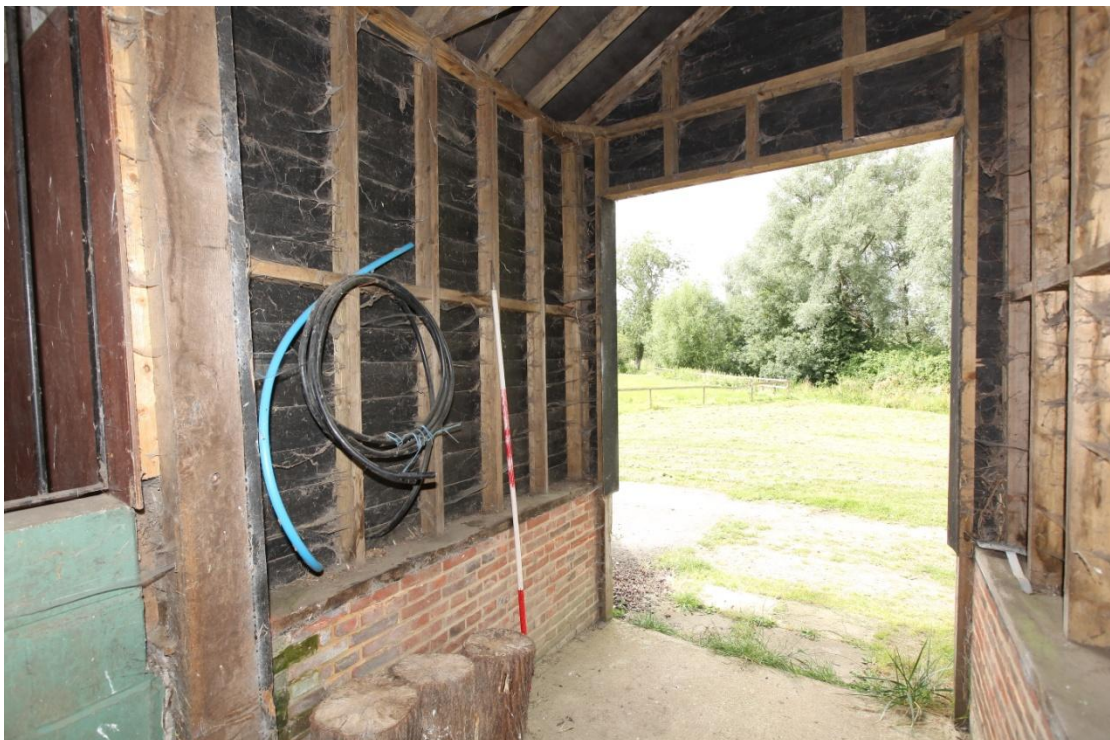
Illus. 8. The western interior of the northern porch of 2003 showing its modern softwood studs and brick plinth laid in traditional English Bond. The listing description refers only an entrance in the western gable and the surviving framing above suggests that no doorway existed in this position when the barn was first built (illus. 9).
