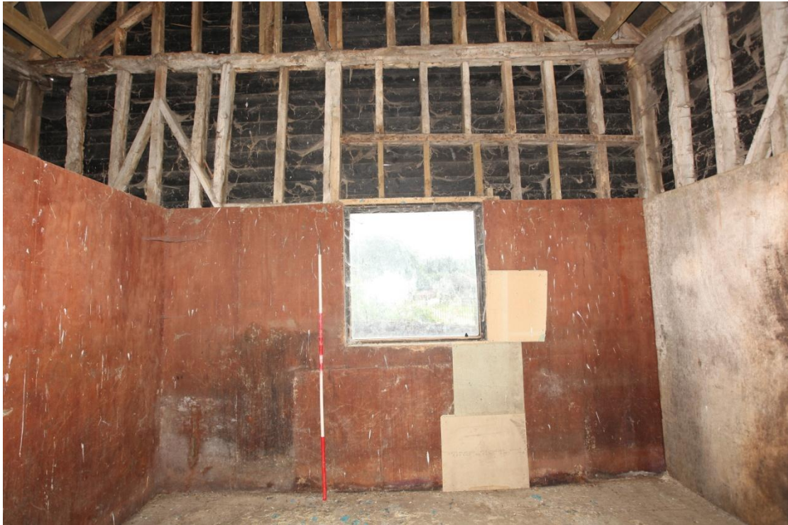
Illus. 13. The western internal gable showing the re-used tie-beam with empty pegged mortices for substantial flat-sectioned studs in the manner of the 17 th century and before. The short horizontal lintel ostensibly of the gable door mentioned in the 1984 listing survives to the left of the central post while the lintel of a tall, wide entrance lies to the right. The nails in the latter indicate it too was re-used and as the plinth has been rebuilt it is impossible to establish whether this entrance was original or an insertion.
