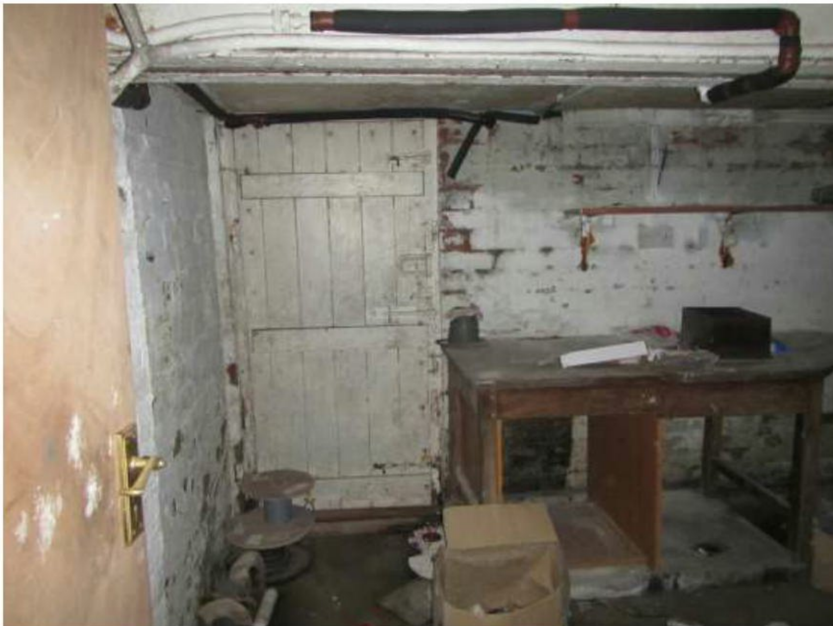
Photograph 18 – Cellar within Building 1.
