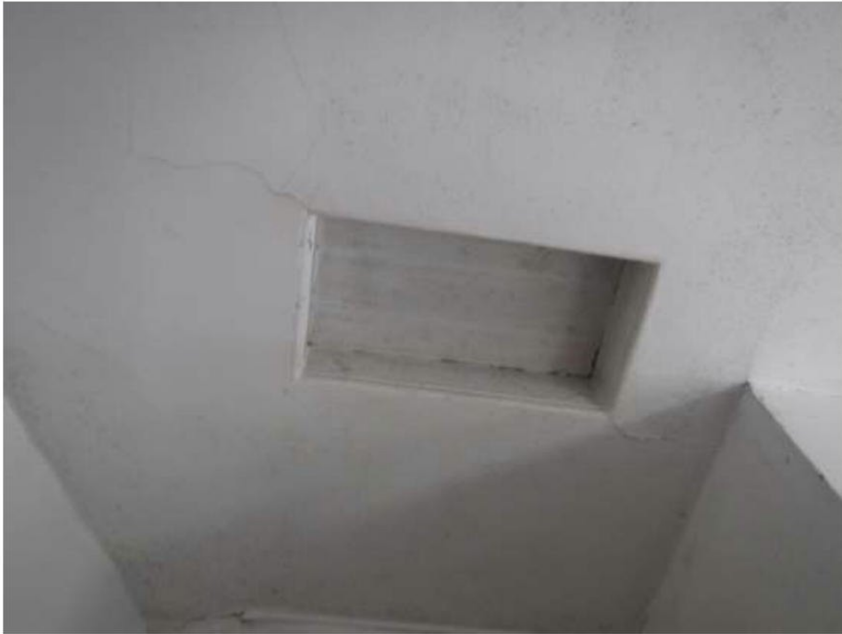
Photograph 17 – View of small loft hatch to Loft 2.
