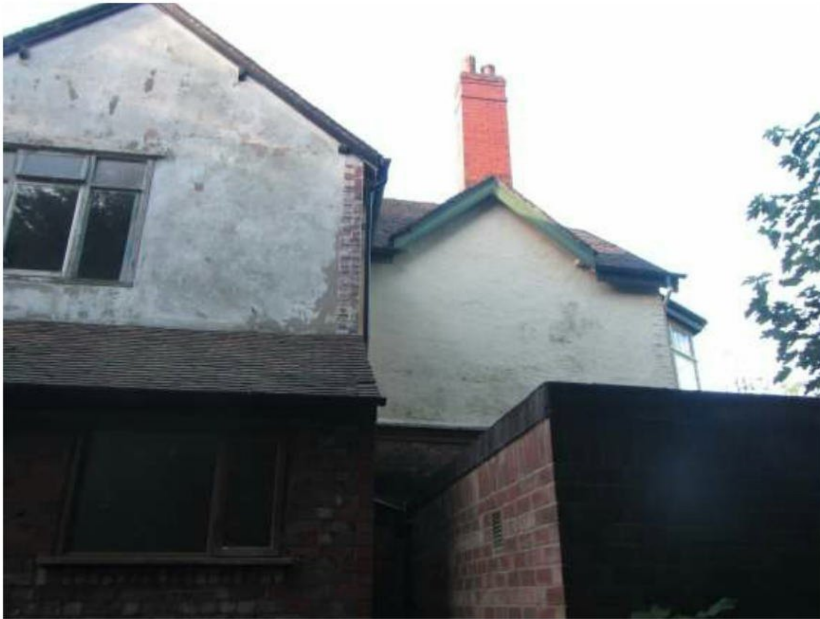
Photograph 11 – Extensions on the northern aspect of the building.
