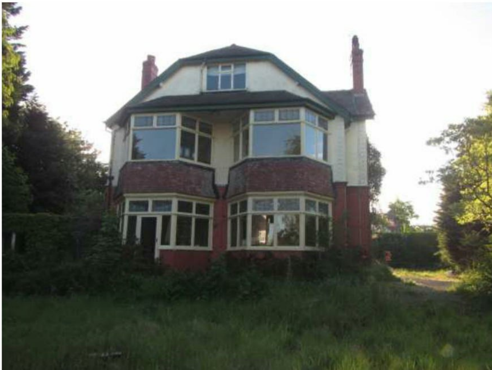
Photograph 8 – View of hanging tiles on the western aspect of the building.
