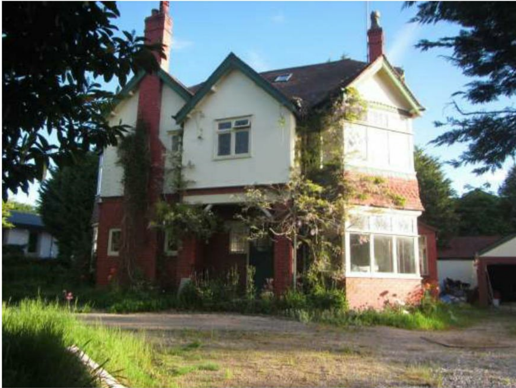
Photograph 1 – Southern aspect of Building 1.
