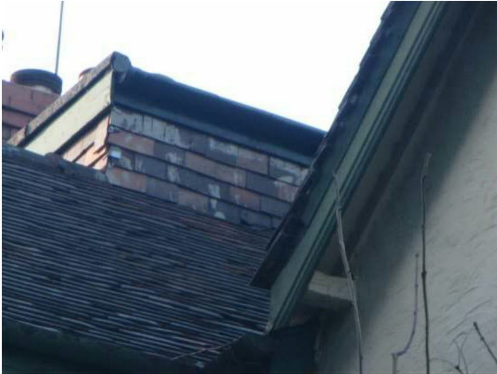
Photograph 5 – Close view of dormer window.
