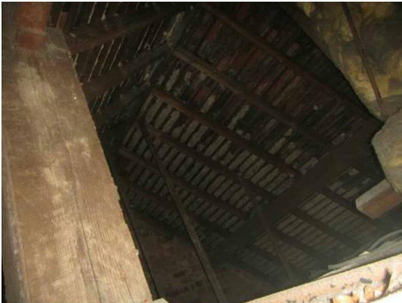
Photograph 16 – View of Loft 2, within Building 2.
