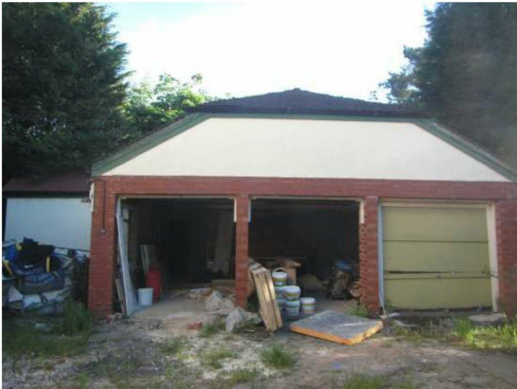
Photograph 12 – Southern aspect of garage (Building 2).
