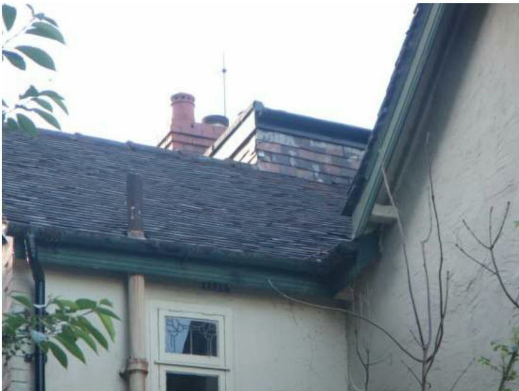
Photograph 4 – View of dormer on the north-eastern aspect of the building.
