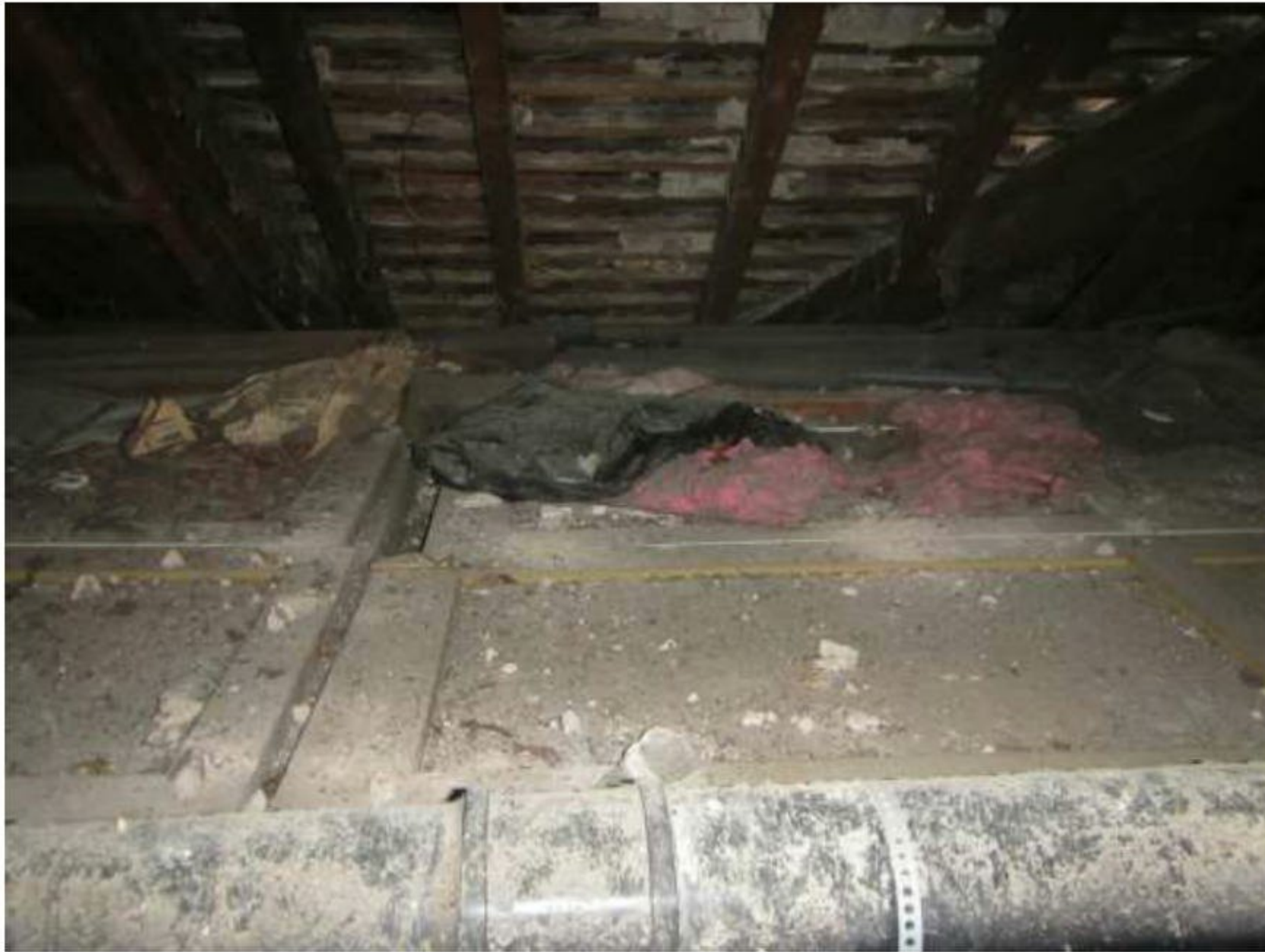
Photograph 15 – View of Loft 1, within Building 1.
