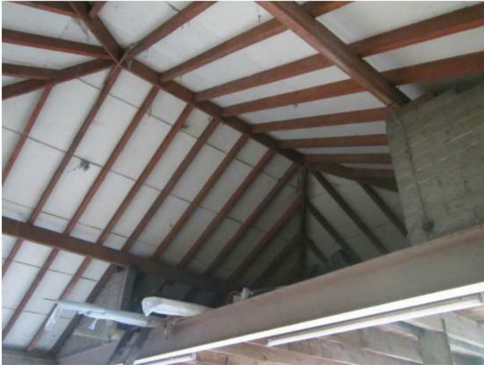
Photograph 19 – Mezzanine section within Building 2.
