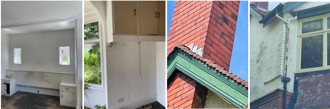
Chimney breasts affected by soot/salt
