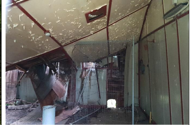
Photograph 3: Internal view of billiard hall.
