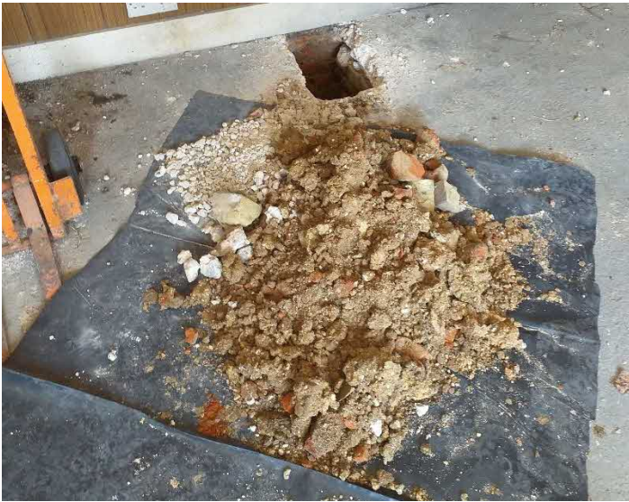
Photo 13: View of soil arisings hand dug from trial pit TP-3.
