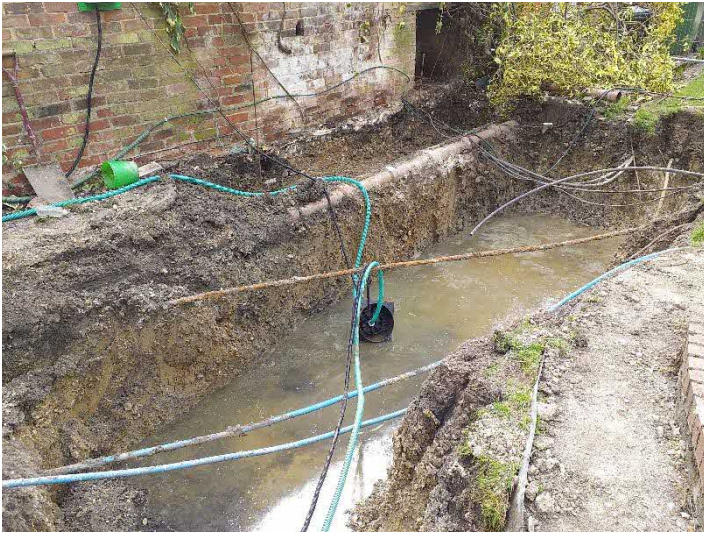
Photo 4: Extent of current remedial excavation to the north of the garage.
