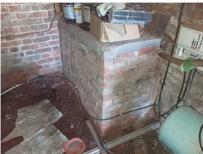
Photo 12: Brick structure within the boiler room.
