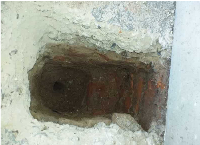
Photo 14: View of below ground brickwork exposed within TP-3.
