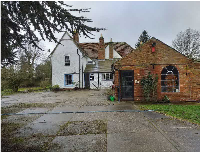
Photo 2: Rear elevation to the property.
