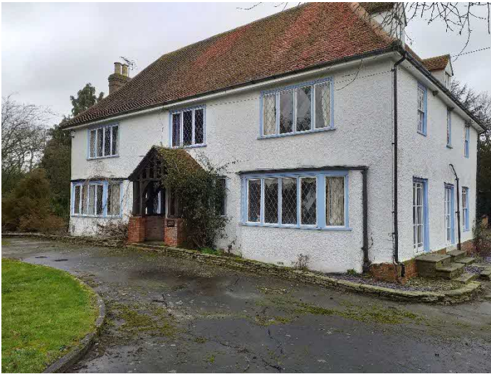
Photo 1: Front elevation to the property.
