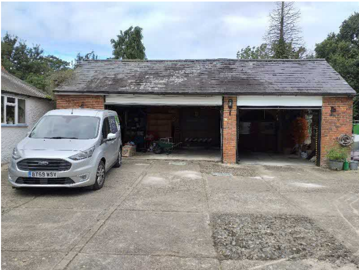
Photo 5: View of the garage door openings to room 1 (right) and room 2 (left).
