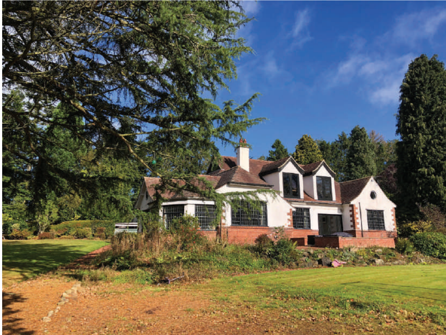
Existing Site Photograph
