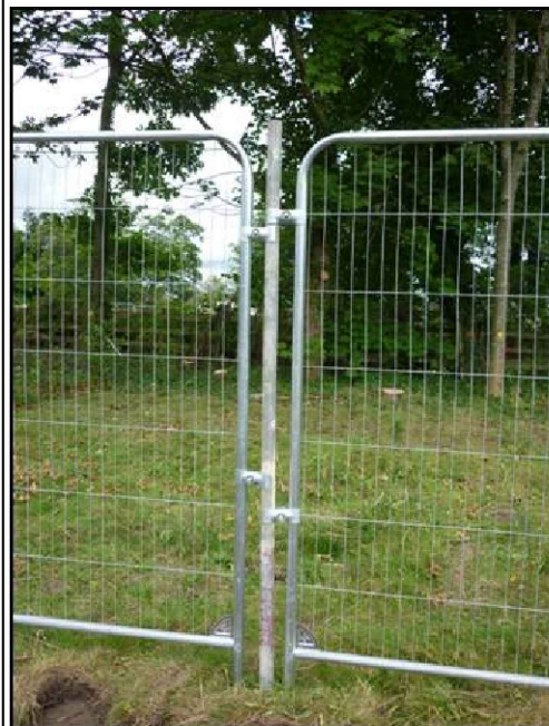
Tree Protective Fencing Specification
