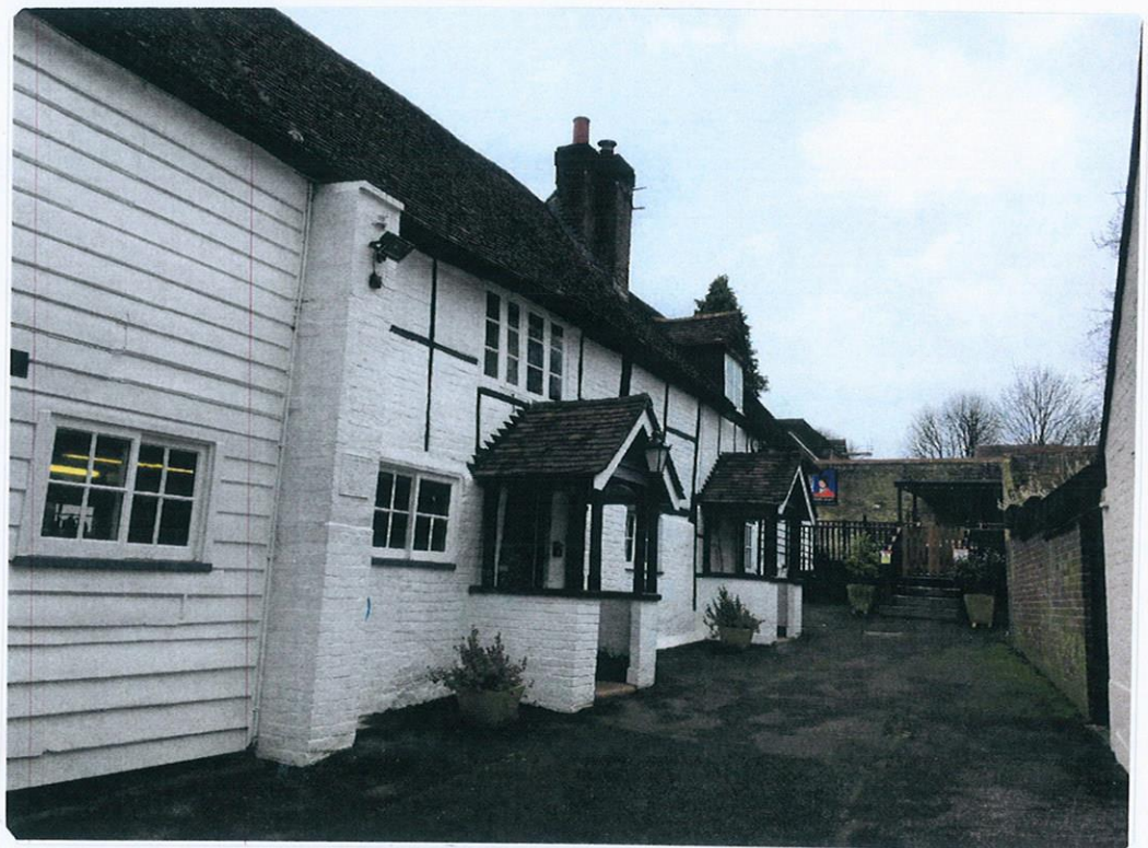
GENERAL VIEW TO EAST ELEVATION RETAINED MAIN ENTRANCE AND ENTRANCE PORCH IN FOREGROUND. 'NORTH PORCH' IN BACKGROUND TO BE 'REINSTATED FOR ACCESS.'
