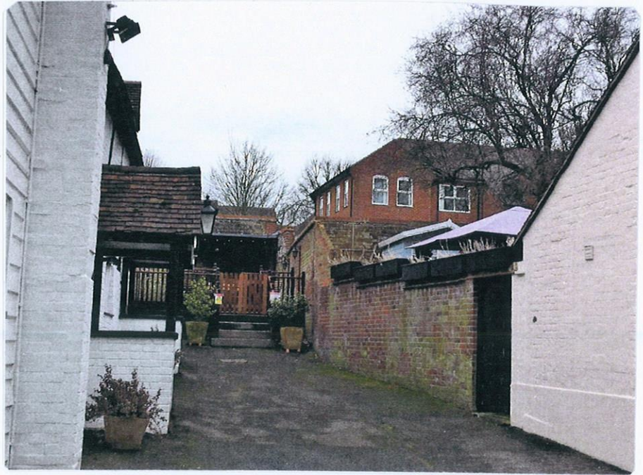
EAST ELEVATION GENERAL VIEW TO REAR. RETAIN RIGHT OF WAY TO EXISTING ADJACENT SPRING ARDENS.
