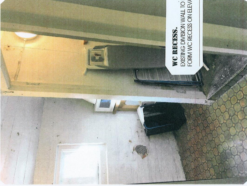
FLOOR COVERING. EXISTING SHEET FLOOR COVERING TO BE REMOVED AND REPLACED WITH TIMBER BOARDED FLOOR.
