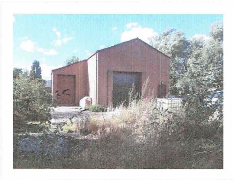
Photo 2: Front view showing side room.
